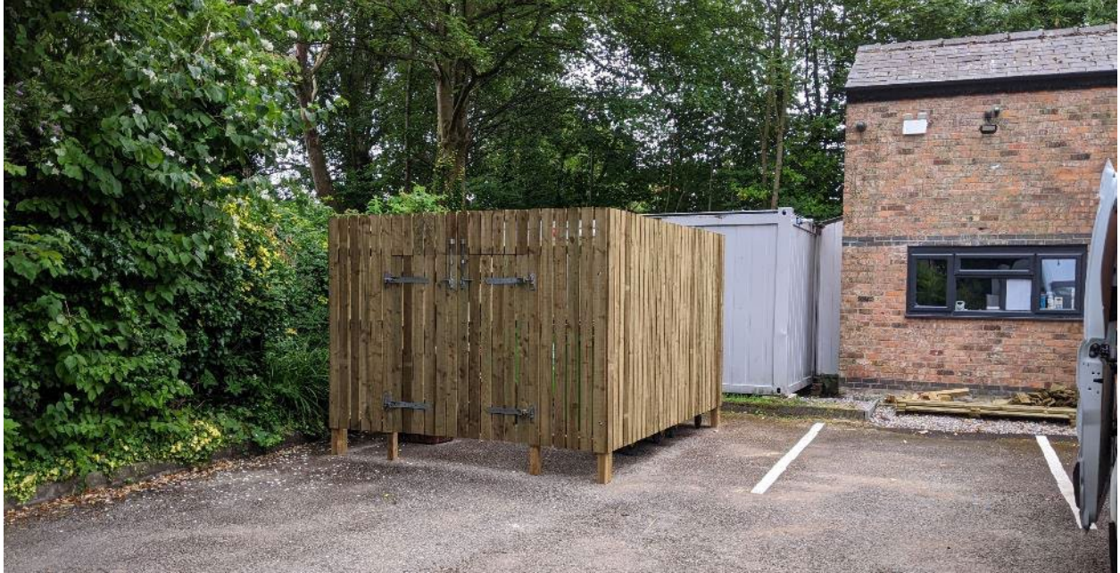
Portacabin units installed as an extension to the annexe building within the southwestern corner of the site.
