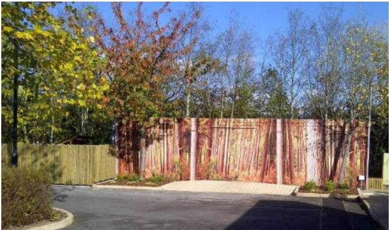
Example of portacabin unit wrapped in woodland blending external wrapping.
