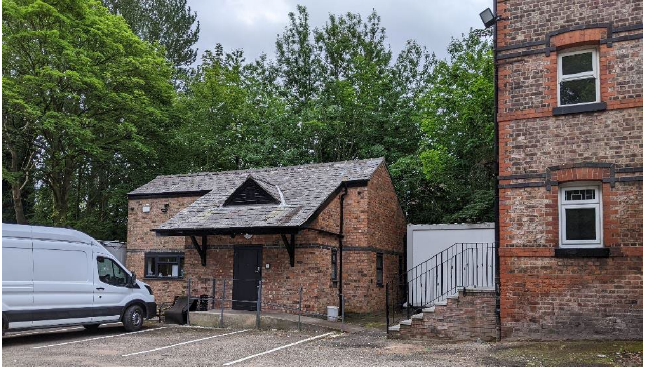
Standalone Portacabin unit installed between the two primary buildings adjacent to the southern site boundary.
