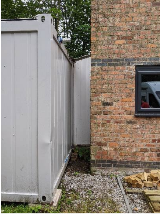
Lean to structure connecting the three units to the annexe dining room building.
