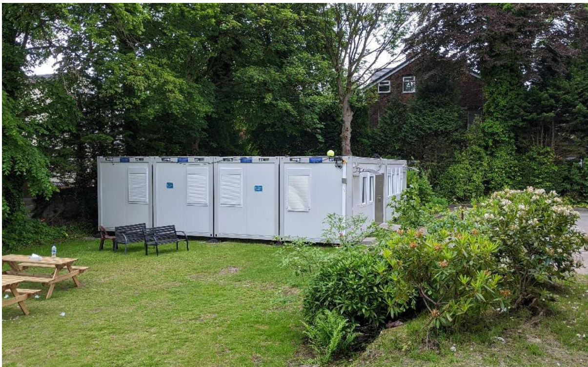
Alternative view of the existing portacabin units from inside the site looking westwards. This view is not visible from the street scene
