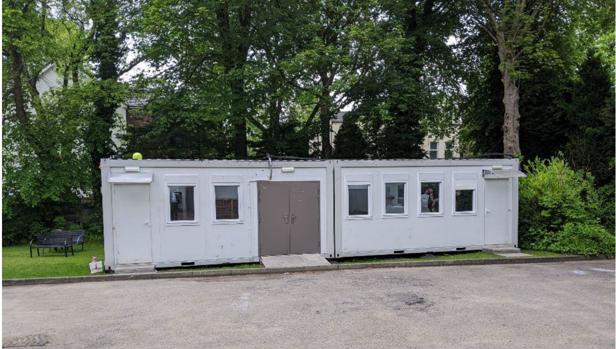
Group of 8 connected portacabin units utilised as a large lecture room and assembly hall. View from the car parking area inside the site looking at the front of the units.
