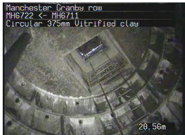
MH6711X_f5eb8ef0-e23a-47c7-a54e-6493bf9cd807_20230718_120421_809.jpg, 00:08:21, 28.56 m Finish node, manhole, reference: MH6711
