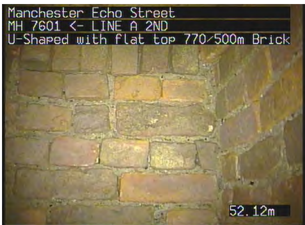
LINE A 2NDX_ac6685d6-facc-4cc7-843f-db48eacf1117_20230717_1 30916_805.jpg, 00:24:37, 52.12 m Finish node, other special chamber, reference: LINE A 2ND, CAPPED END
