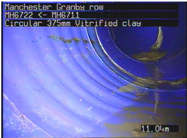
MH6711X_4480029e-3ef1-42c4-8b16-6c9c30b20e4c_20230718_115425_171.jpg, 00:03:02, 11.04 m Line deviates right
