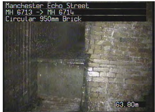
MH 6713X_9ce91352-b92b-42e0-80f4-d611e9deeb8e_20230717_141718_632.jpg, 00:07:05, 63.80 m Finish node, manhole, reference: MH 6714
