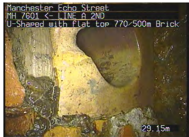
LINE A 2NDX_6a6d3177-ca9d-4338-b095-2fee5614ffd7_20230717_1 24902_822.jpg, 00:05:45, 29.15 m Connection other than junction at 11 o'clock, 150mm dia
