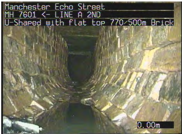
LINE A 2NDX_4e5e1bfd-56a2-4a5f-9853-9e0d99b1fb99_20230717_1 24118_824.jpg, 00:00:03, 0.00 m Water level, 5% of the vertical dimension
