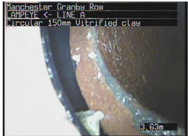
LINE A X_9b2ea69f-8408-4bd3-a7da-bb8931d14aa4_20230718_102 730_868.jpg, 00:00:45, 3.63 m Line deviates right
