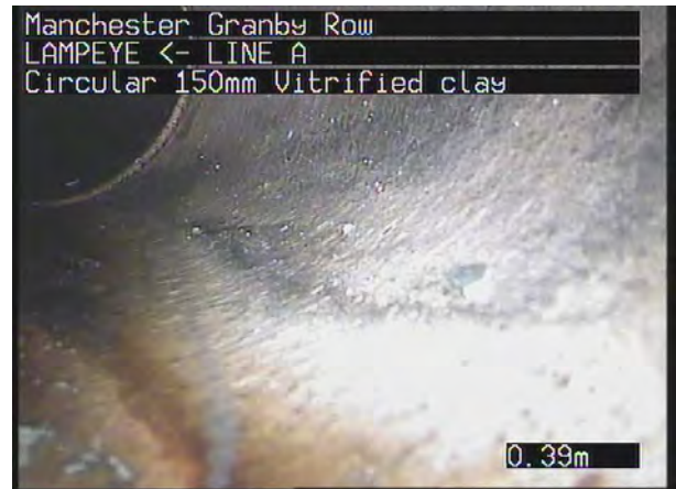
LINE A X_83d8cf41-2026-4e8f-abae-7f84a1be78ba_20230718_10265 4_487.jpg, 00:00:15, 0.39 m Line deviates left
