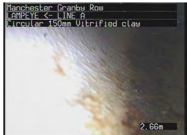
LINE A X_85c09618-66b1-4316-b75e-7aa76ab088d5_20230718_102 713_325.jpg, 00:00:28, 2.66 m Line deviates up
