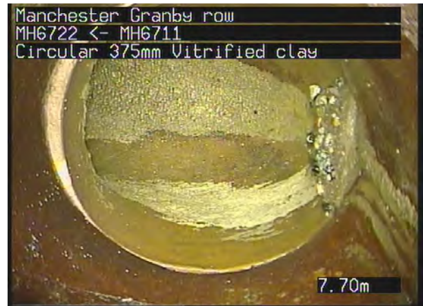
MH6711X_ee74eb02-5856-4f5e-ba34-1166509d1127_20230718_115156_785.jpg, 00:01:24, 7.70 m Junction at 03 o'clock, 150mm dia
