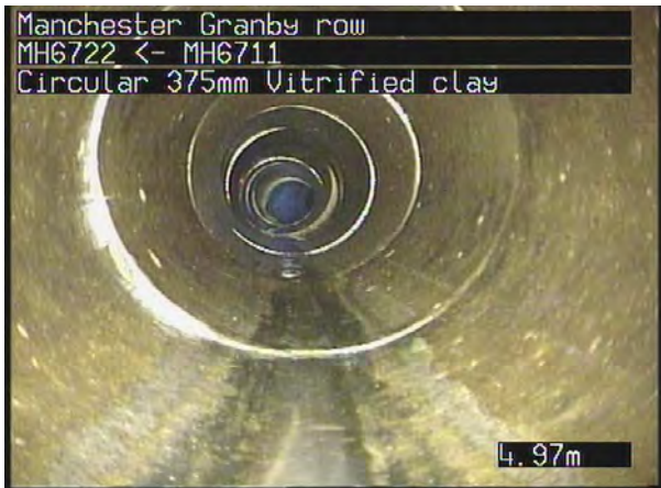
MH6711X_2bbe285a-c8cb-437b-a62b-d3c48068656a_20230718_115132_087.jpg, 00:01:05, 4.97 m Water level, 5% of the vertical dimension
