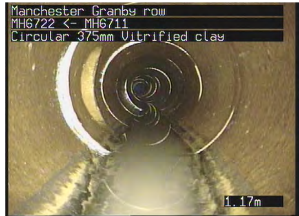
MH6711X_48877146-9bc1-418d-a4c0-126d9dfa3414_202307 18_115027_501.jpg, 00:00:17, 1.17 m Water level, 10% of the vertical dimension
