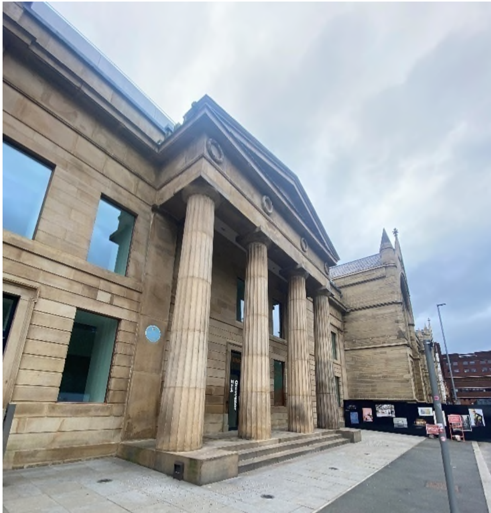
Figure 4.7 – Listed Building 6: Former Town Hall Façade, taken from Cavendish Street looking south (Author's own, 2023)
