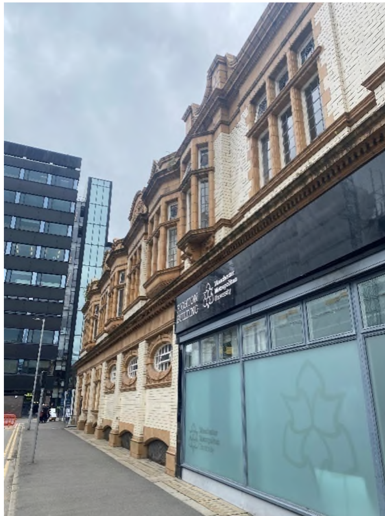
Figure 4.5 – Listed Building 4: Righton Building (Authors own, 2023)
