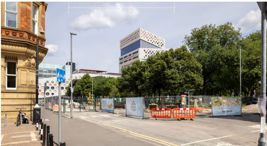
Figure 6-4. View towards Site looking north-east across All Saints Park, with Proposed Development (Planit, 2023)
