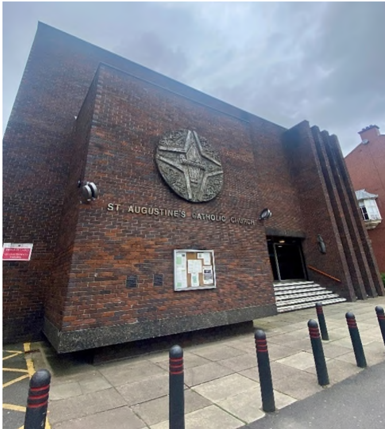
Figure 4.3 - Listed Building 2: Roman Catholic Church of St Augustine (Authors own, 2023)
