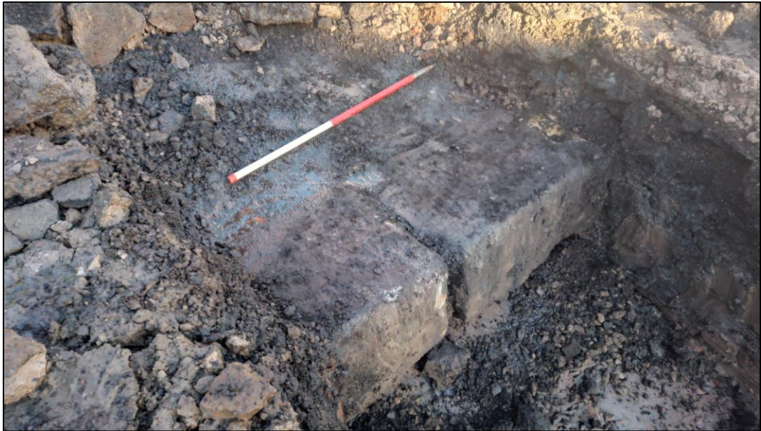
Plate 17: Canal side coping stones, looking north
