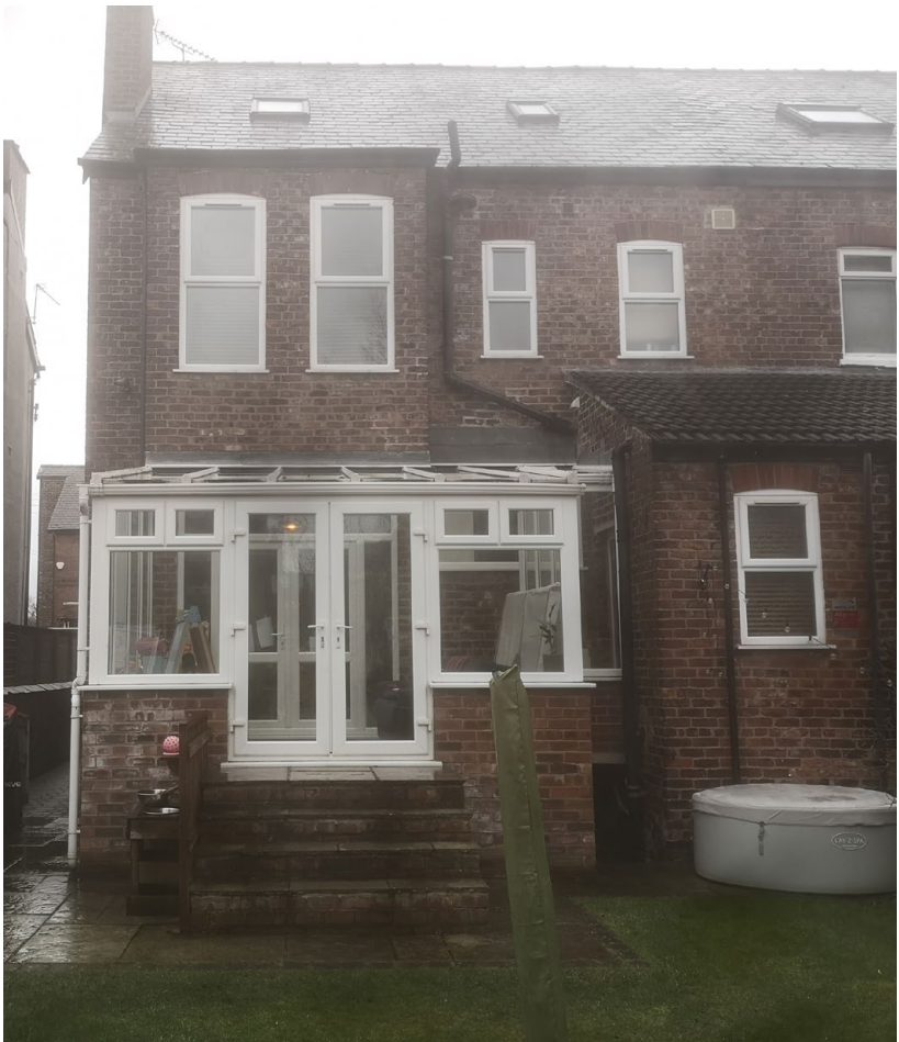
Rear elevation and existing conservatory
