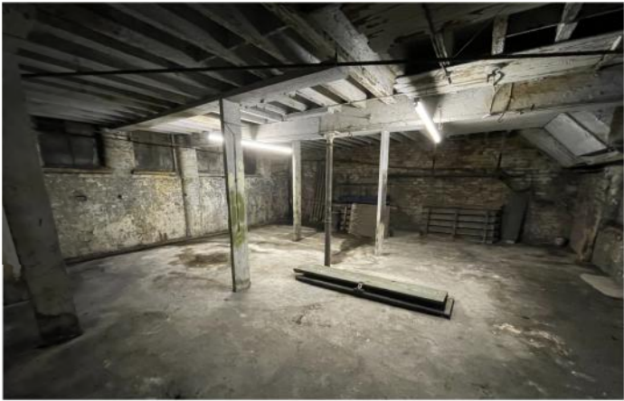
Non-original boxing out of primary beam concealing fire damage.
