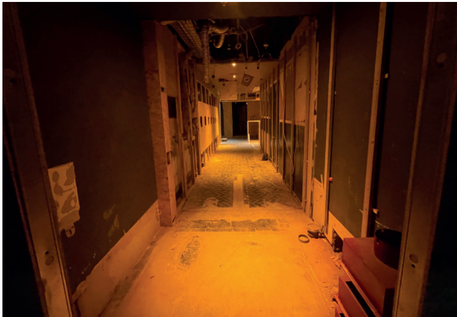
8 View down the corridor
