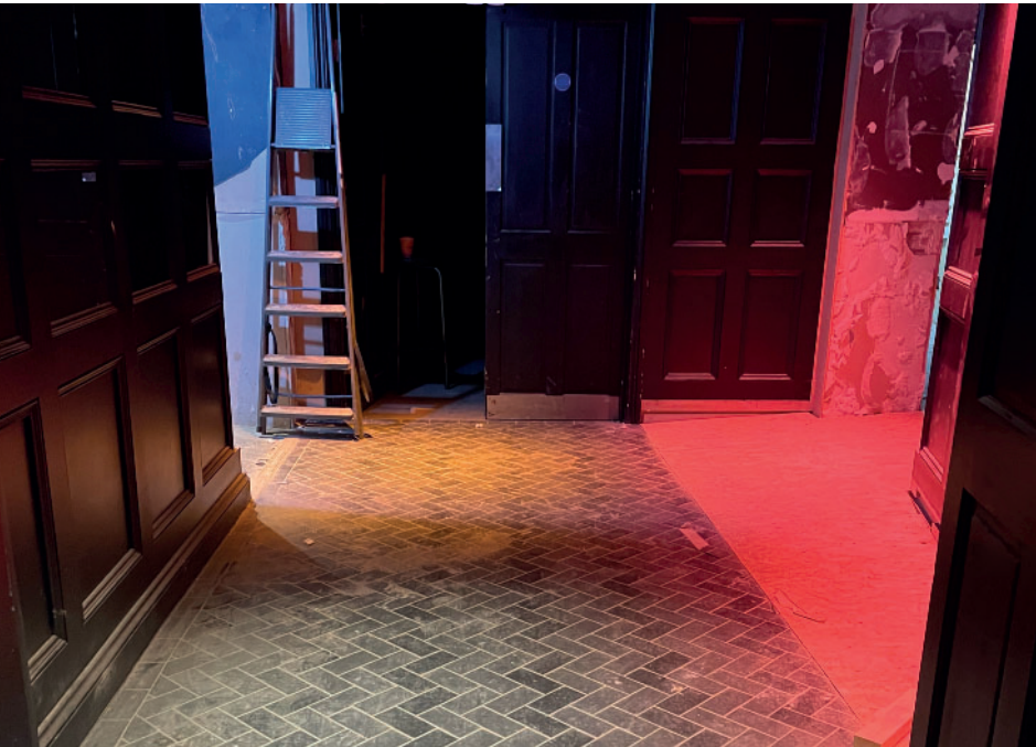
11 View along the corridor
