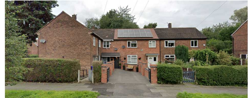
Fig. 21: Existing houses along Longhurst Road
