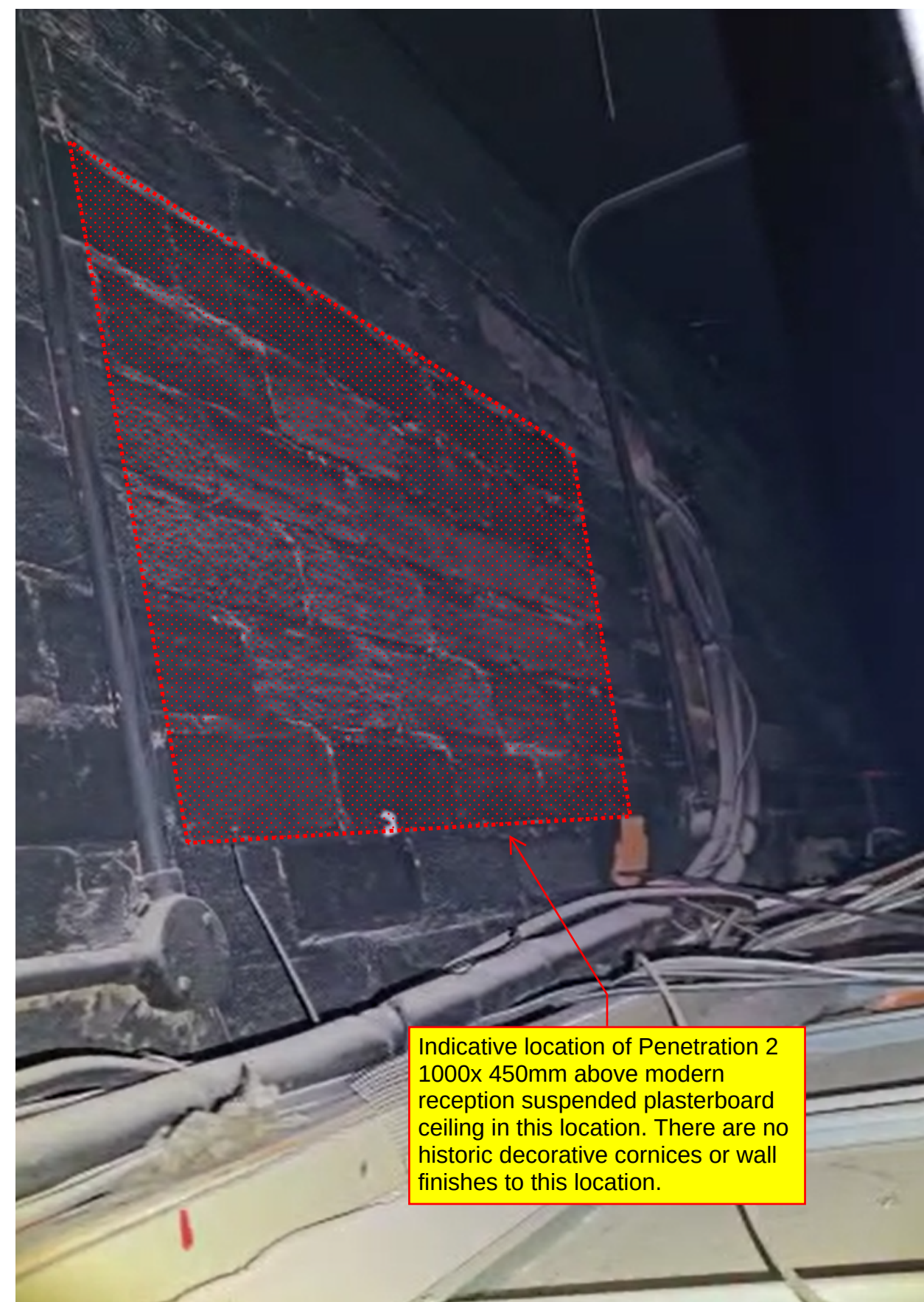
Ground Floor Reception Penetration 2 Photograph 008
