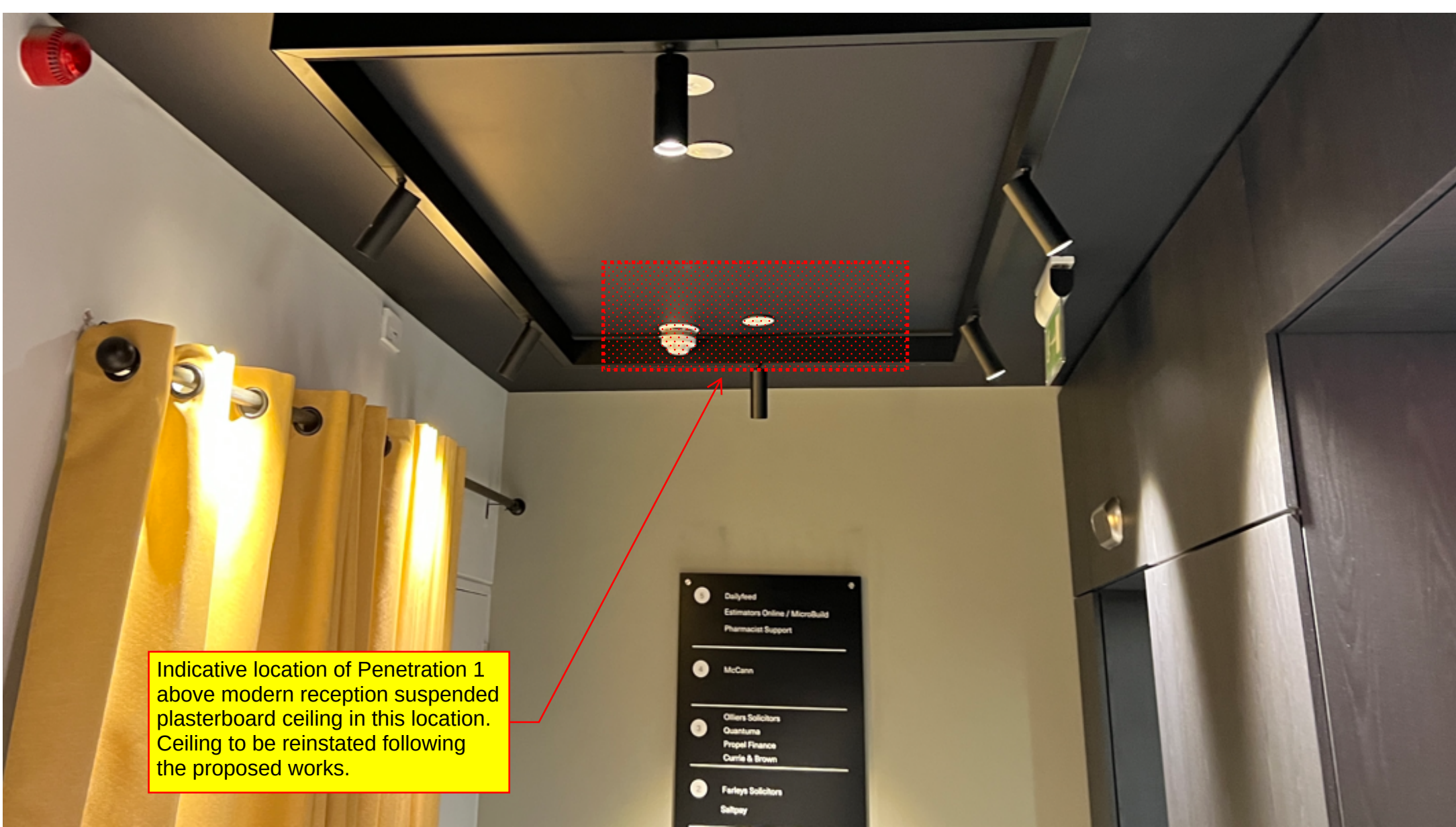
Ground Floor Reception Penetration 1 Photograph 005
