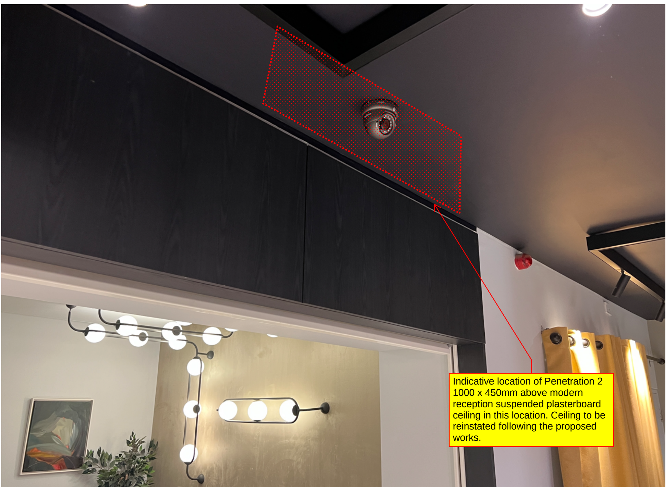
Ground Floor Reception Penetration 2 Photograph 007
