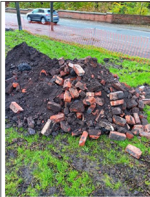
Made ground removed from infilled cellar
