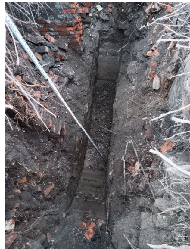
Extent of pit at 5mbgl
