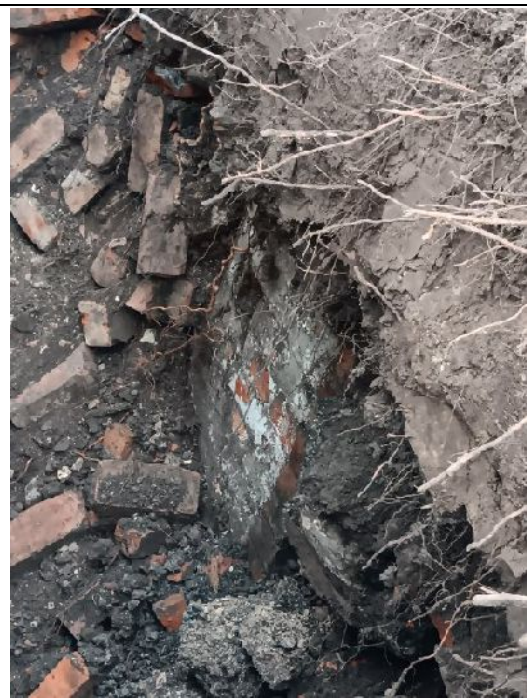
Evidence of side walls from former cellars
