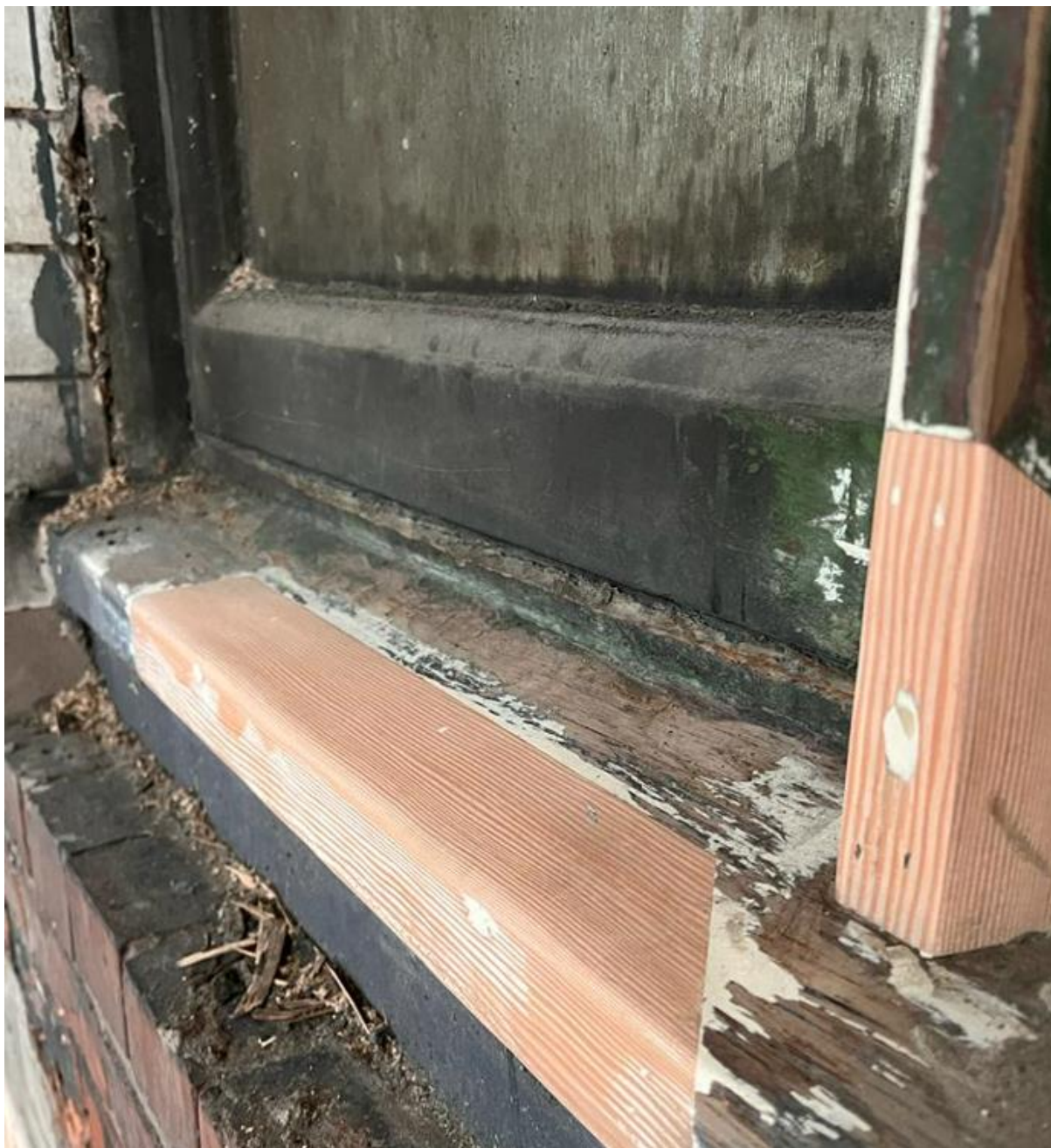
Figure 63: WP.0.08 Repair (Credit CubicWorks Ltd. 2022)
