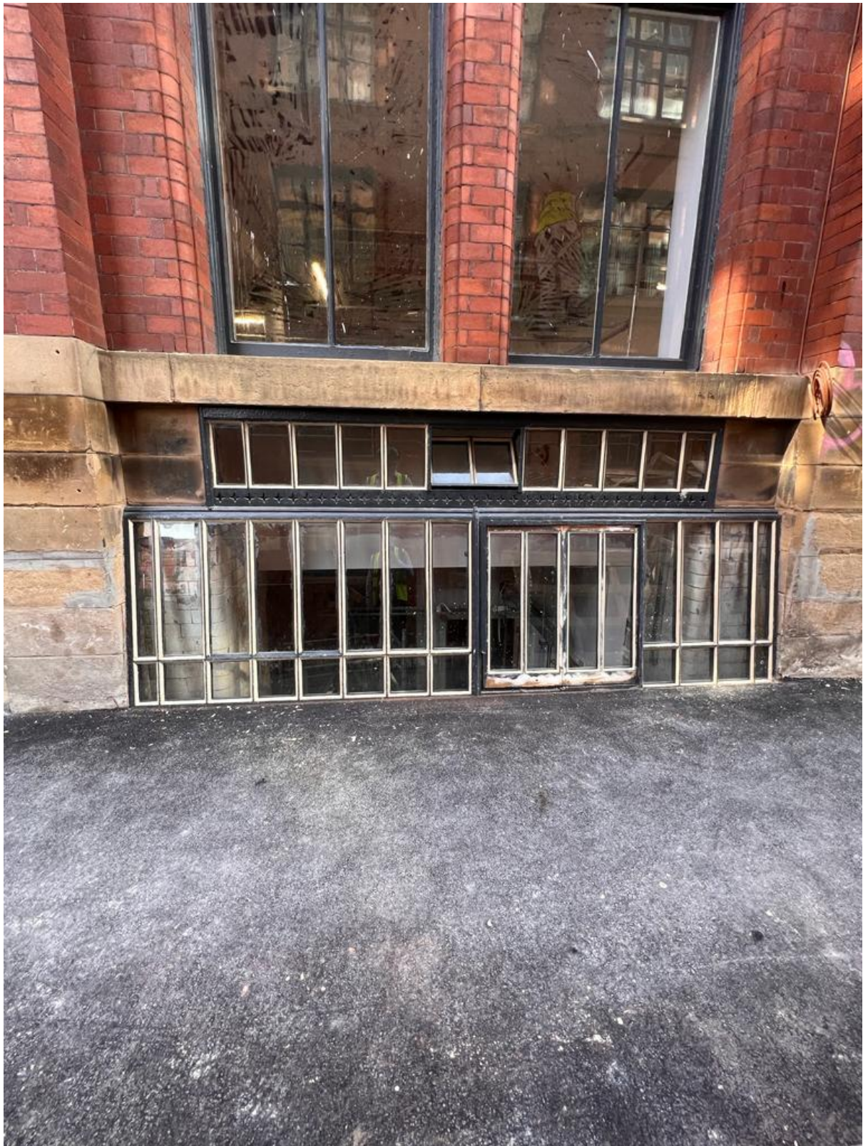
Figure 107: W1-16 & W1-17 (Credit CubicWorks 2023)
