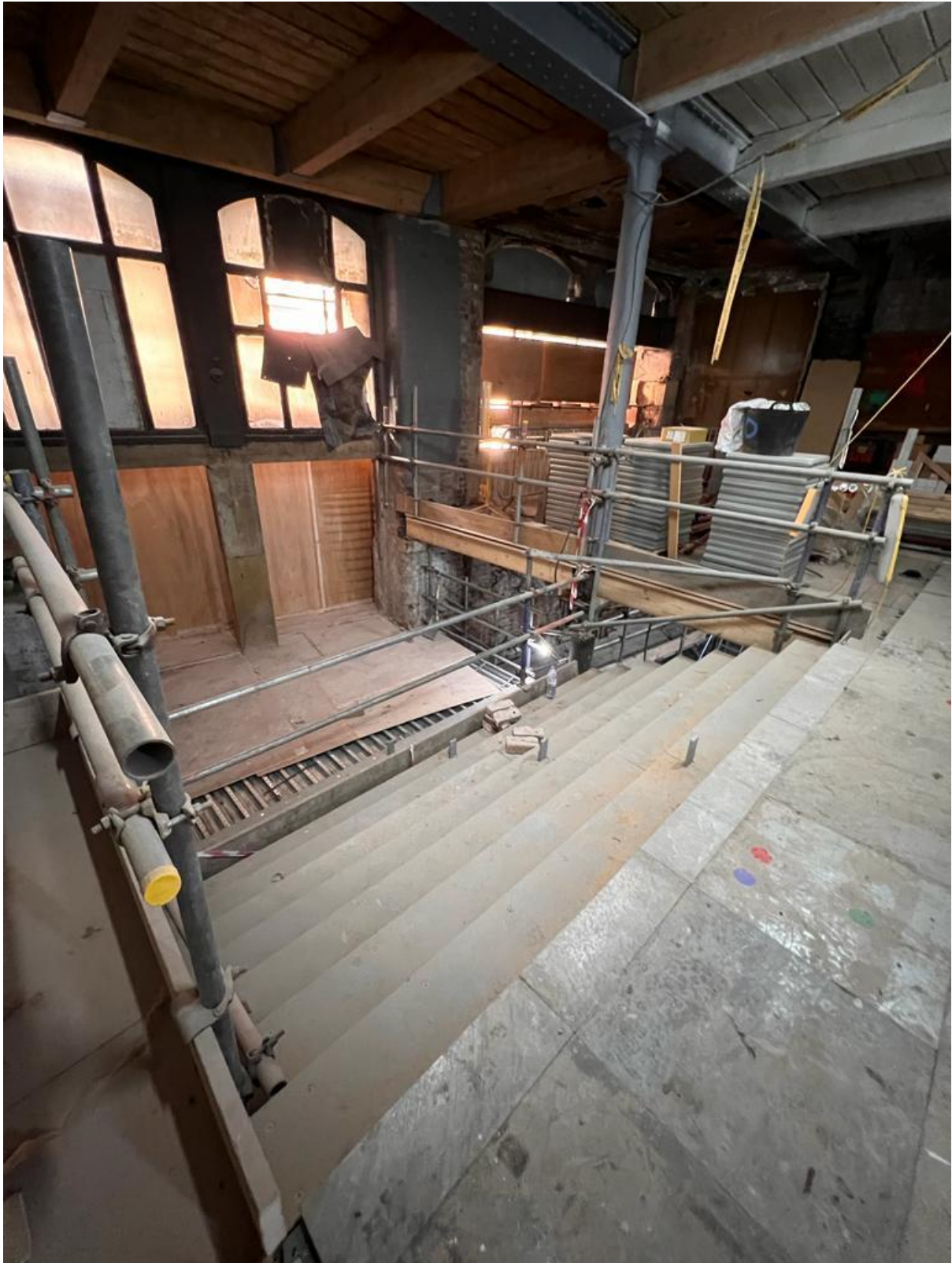
Figure 69: Internal View of the reception windows (Credit CubicWorks 2022)
