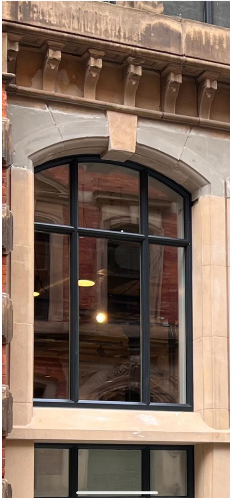
Figure 79: WP.0.01 External (Credit CubicWorks 2023)
