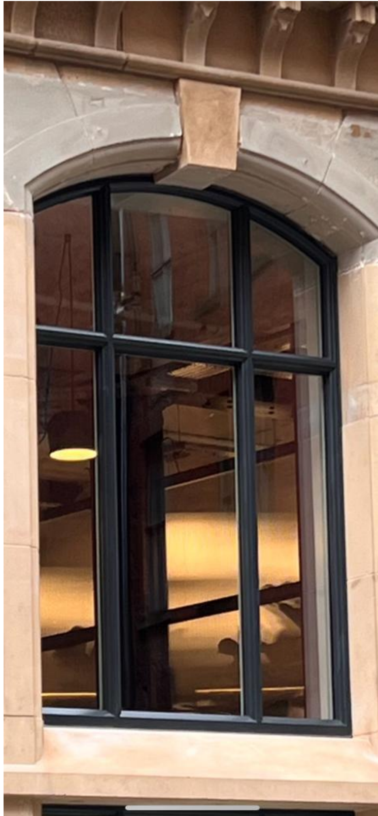
Figure 77: WP.0.02 External (Credit CubicWorks 2023)
