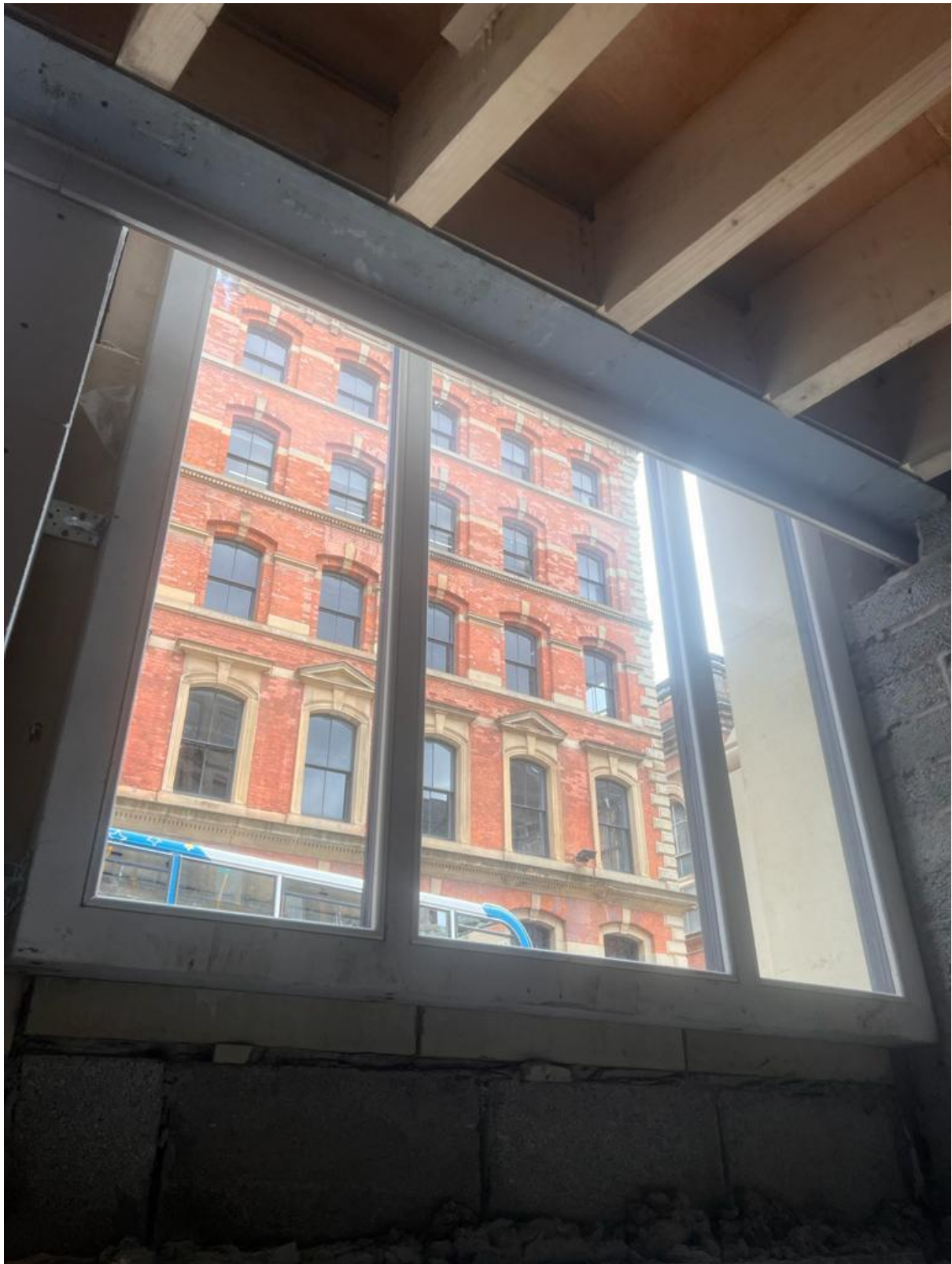
Figure 85: WP.-2.01 Internal (Credit CubicWorks 2023)
