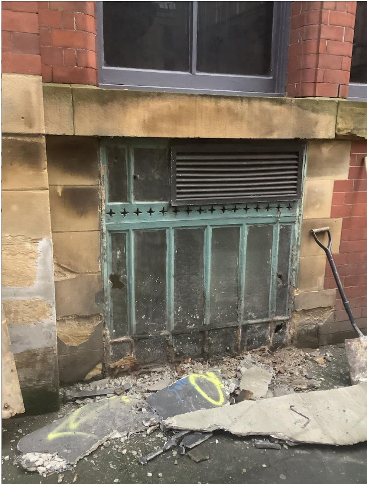
Figure 100: W-1 05 (Credit Bridge 2021)
