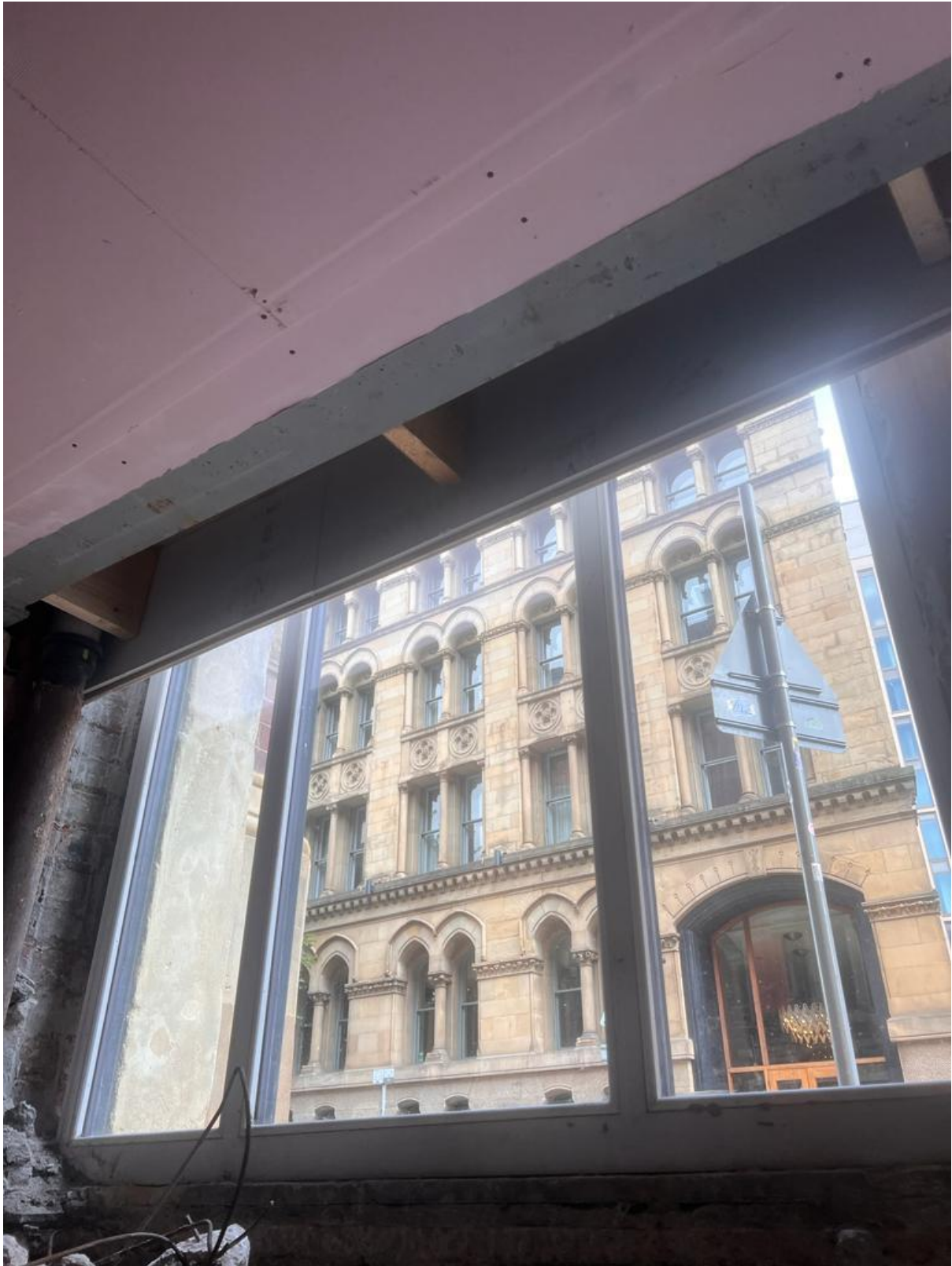
Figure 83: WP.-2.04 Internal (Credit CubicWorks 2023)
