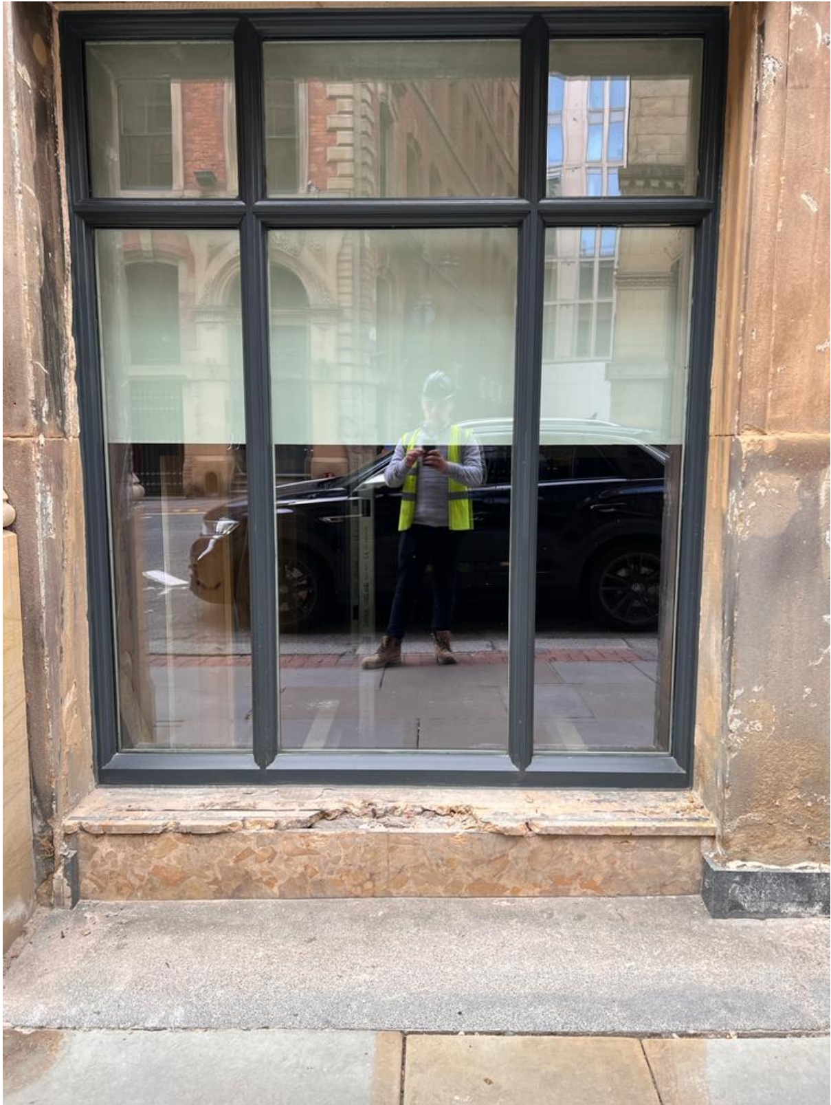
Figure 80 : WP.-2.03 External (Credit CubicWorks 2023)
