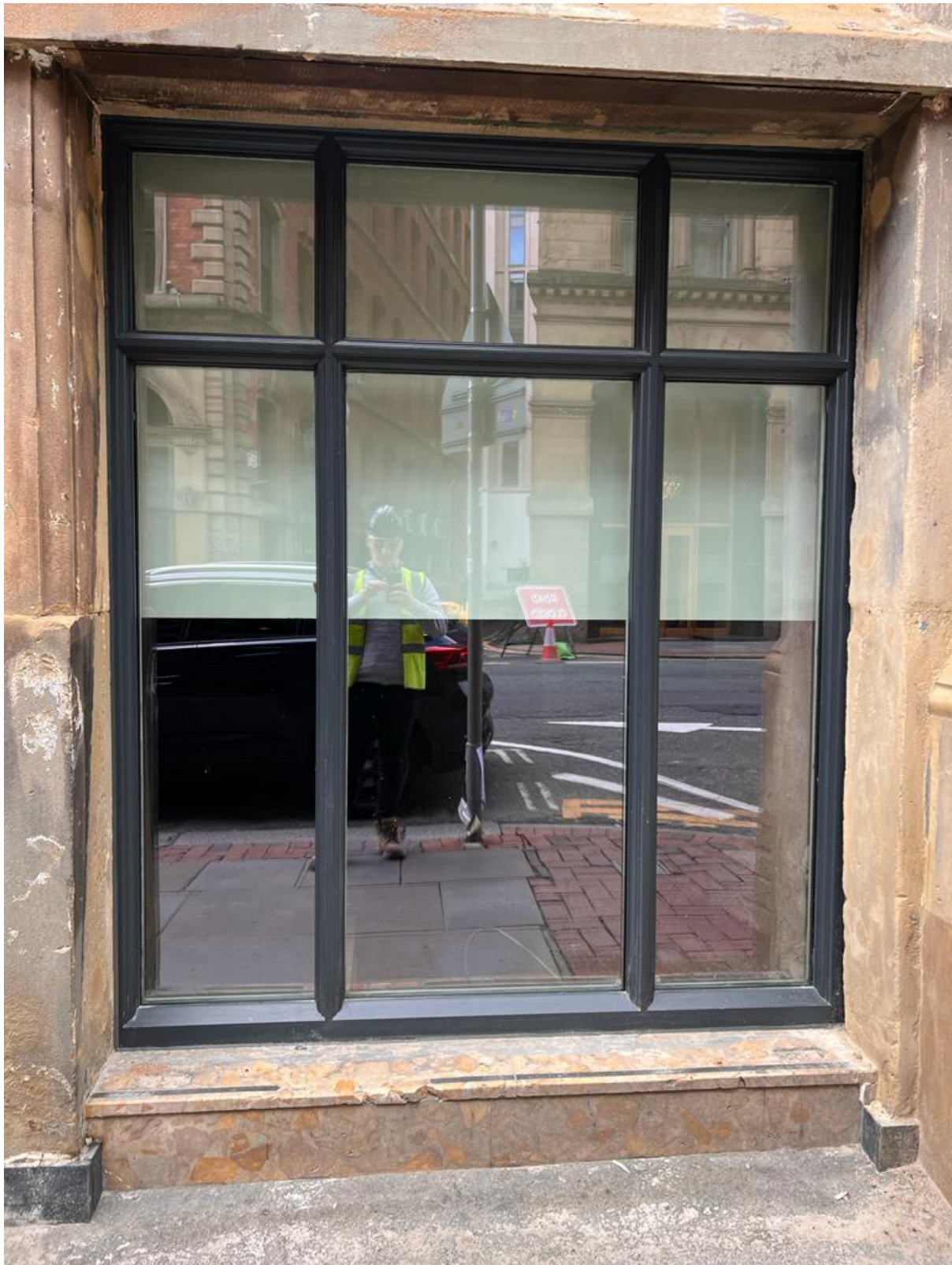
Figure 82: WP.-2.04 External (Credit CubicWorks 2023)
