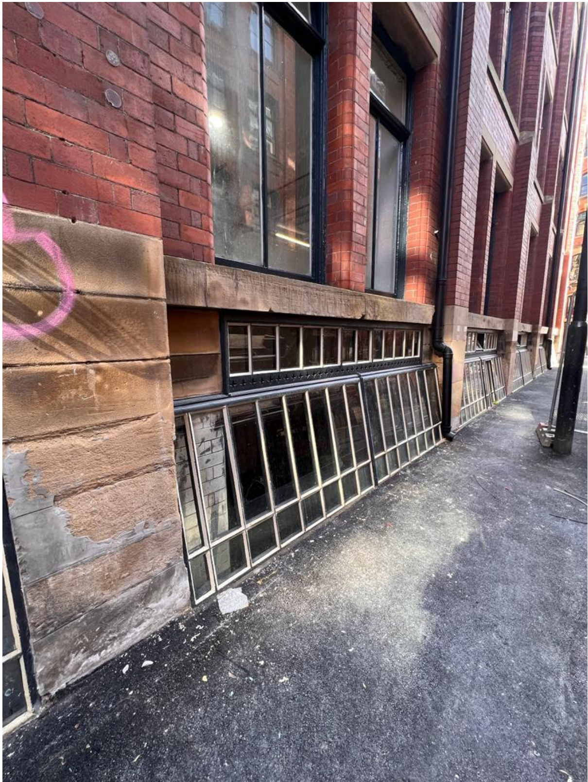
Figure 106: W1-14 & W1-15 (Credit CubicWorks 2023)
