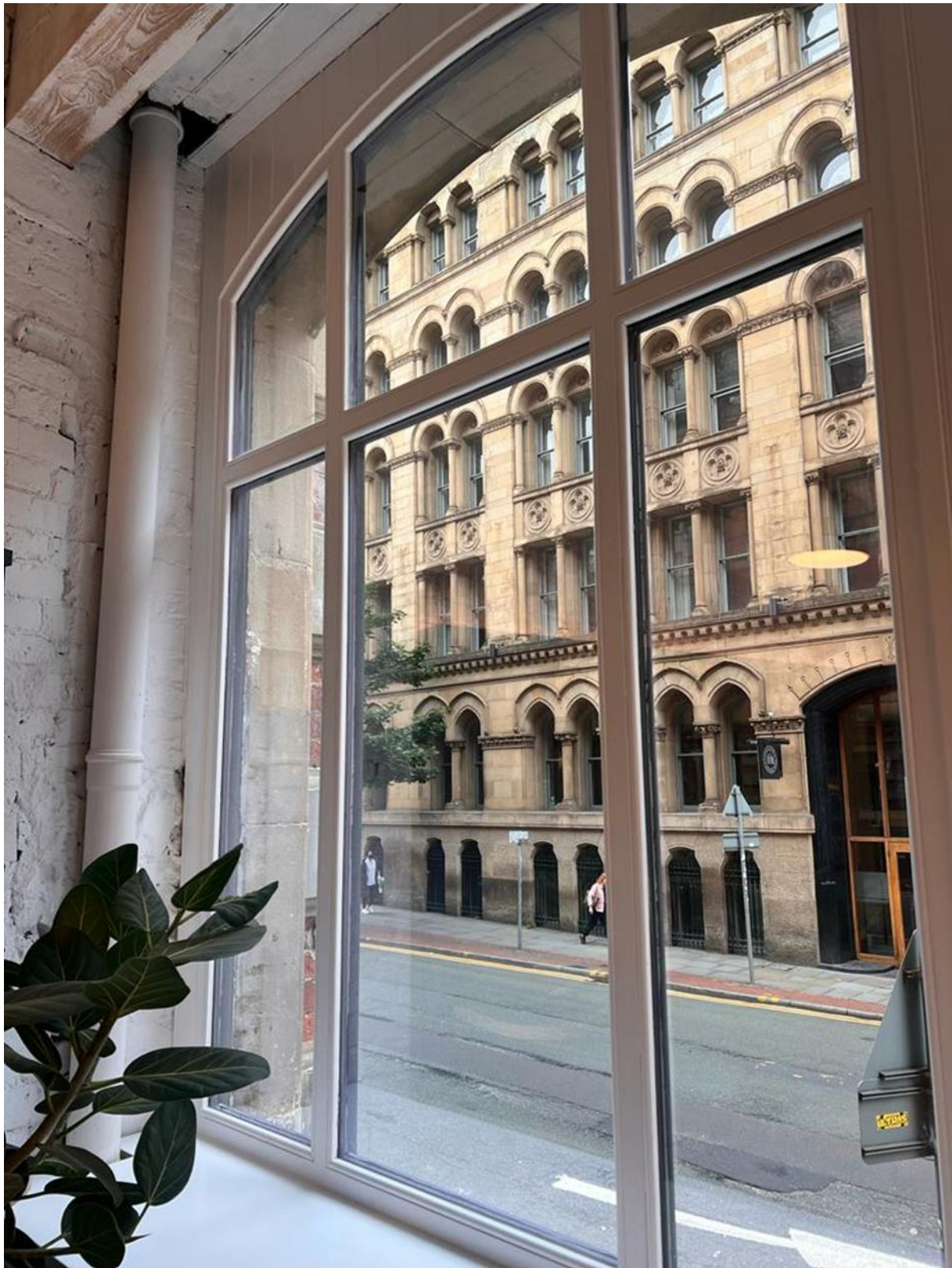
Figure 72: WP.0.06 Internal (Credit CubicWorks 2023)
