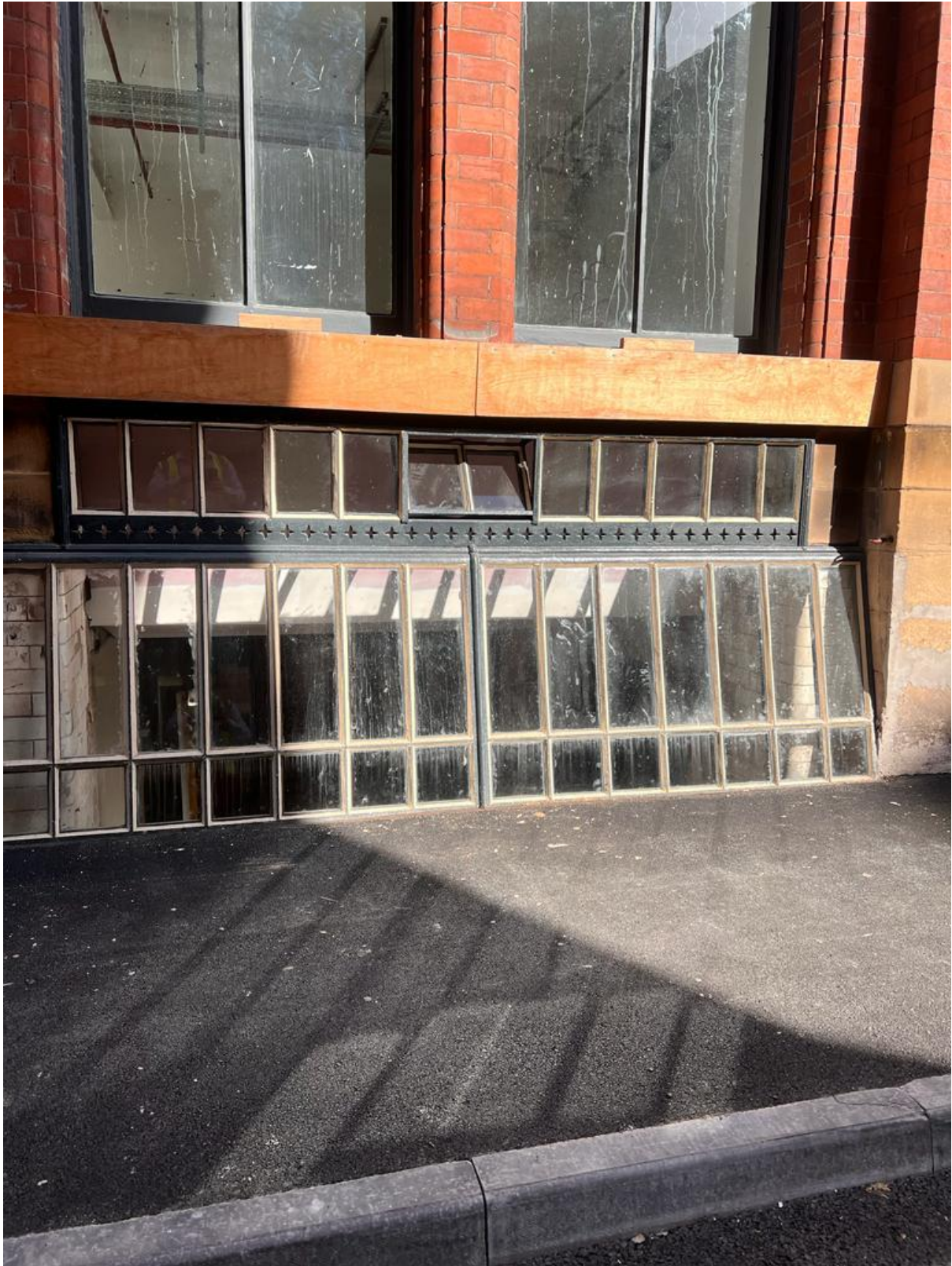
Figure 102: W-1 06 & W1-07 (Credit CubicWorks 2023)
