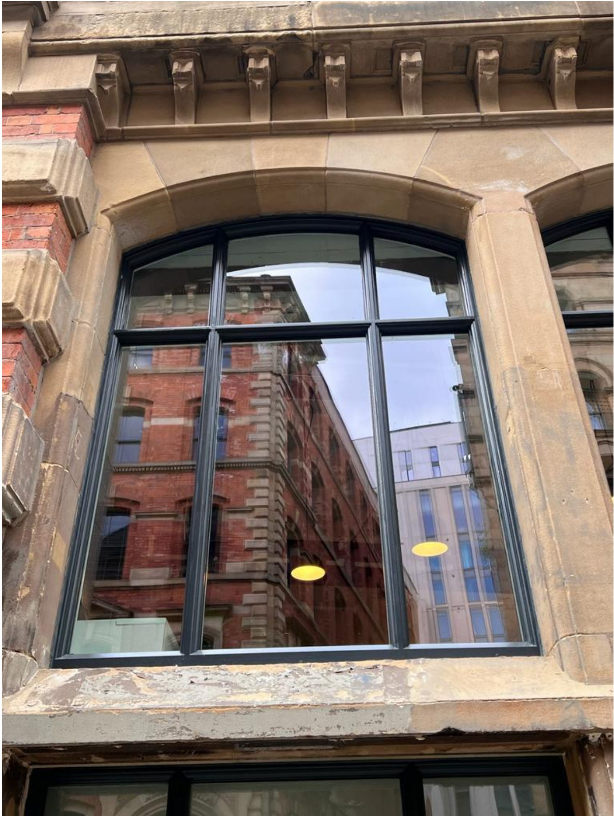
Figure 75: WP.0.05 External (Credit CubicWorks 2023)
