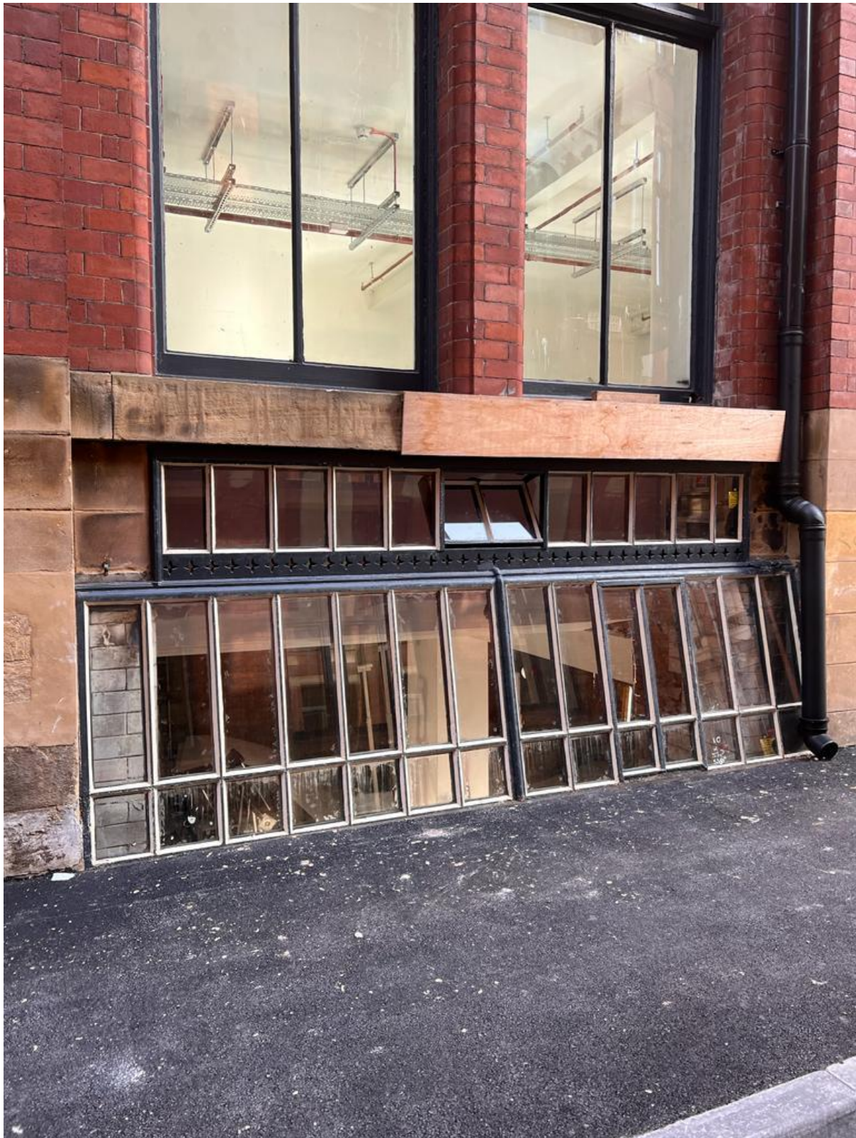
Figure 103: W1-08 & W1-09 (Credit CubicWorks 2023)
