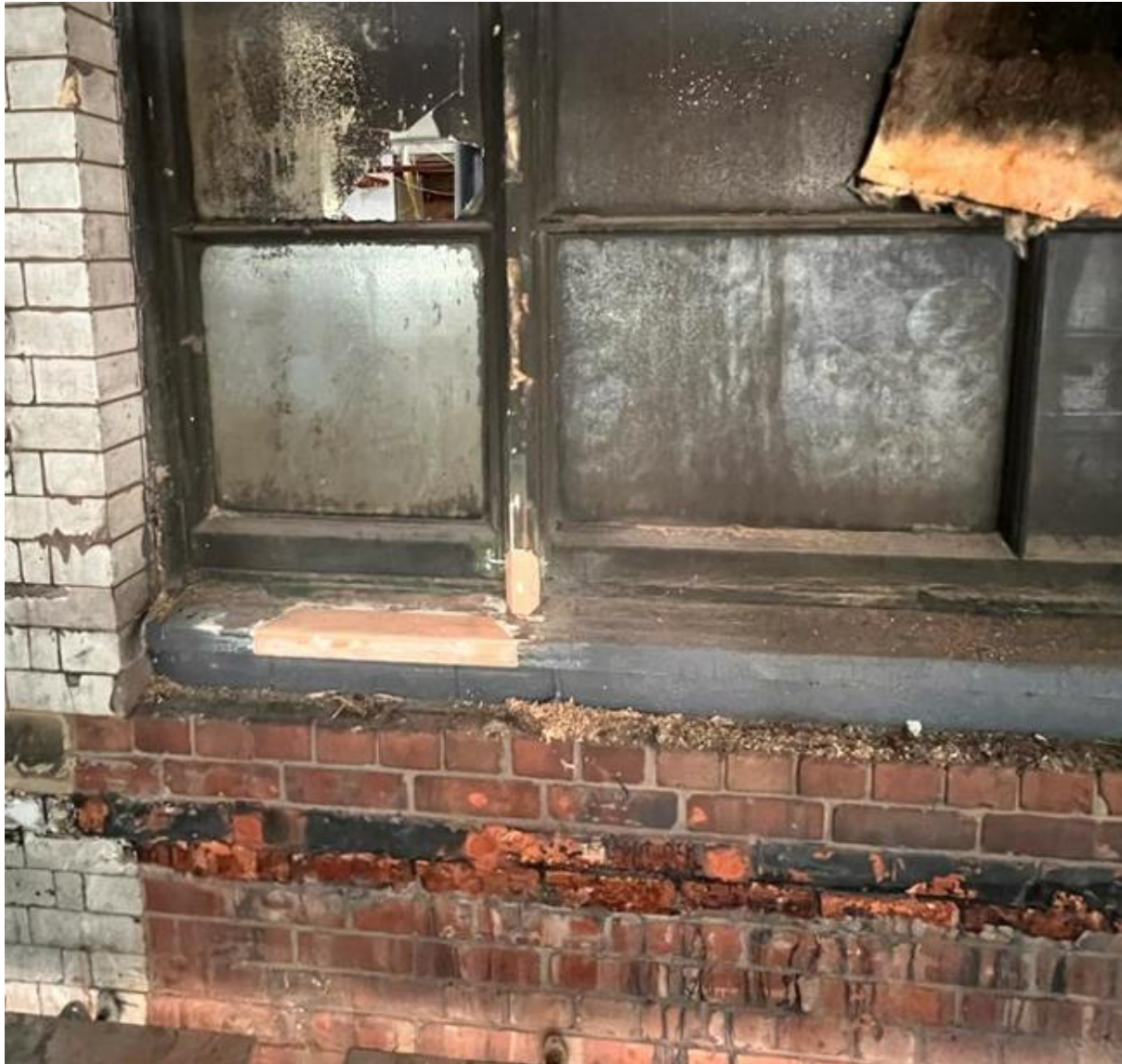
Figure 64: WP.0.08 Repair (Credit CubicWorks Ltd. 2022)
