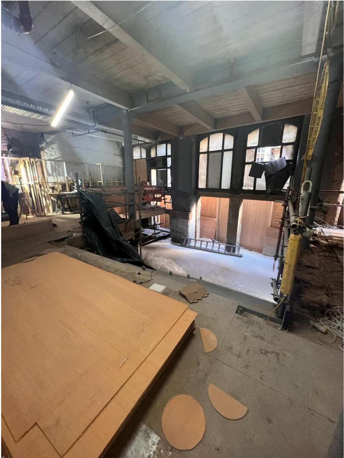
Figure 70: Internal View of the Reception Windows (Credit CubicWorks 2022)
