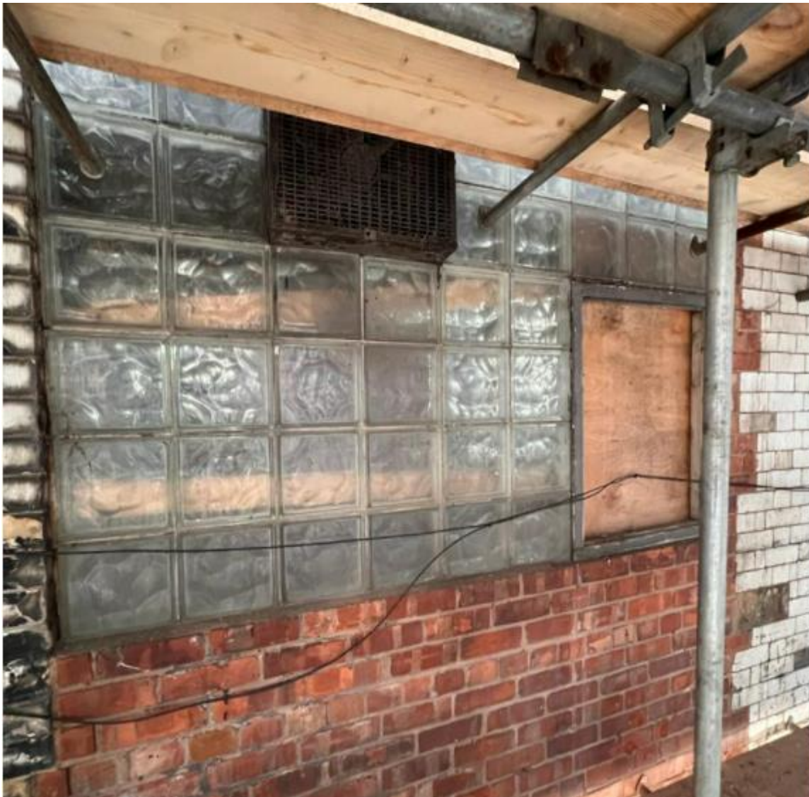
Figure 66: External view of WP.0.11 (Credit CubicWorks Ltd. 2022)
