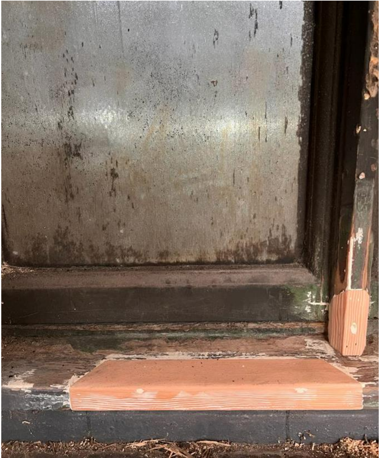
Figure 62: WP.0.08 Repair (Credit CubicWorks Ltd. 2022)
