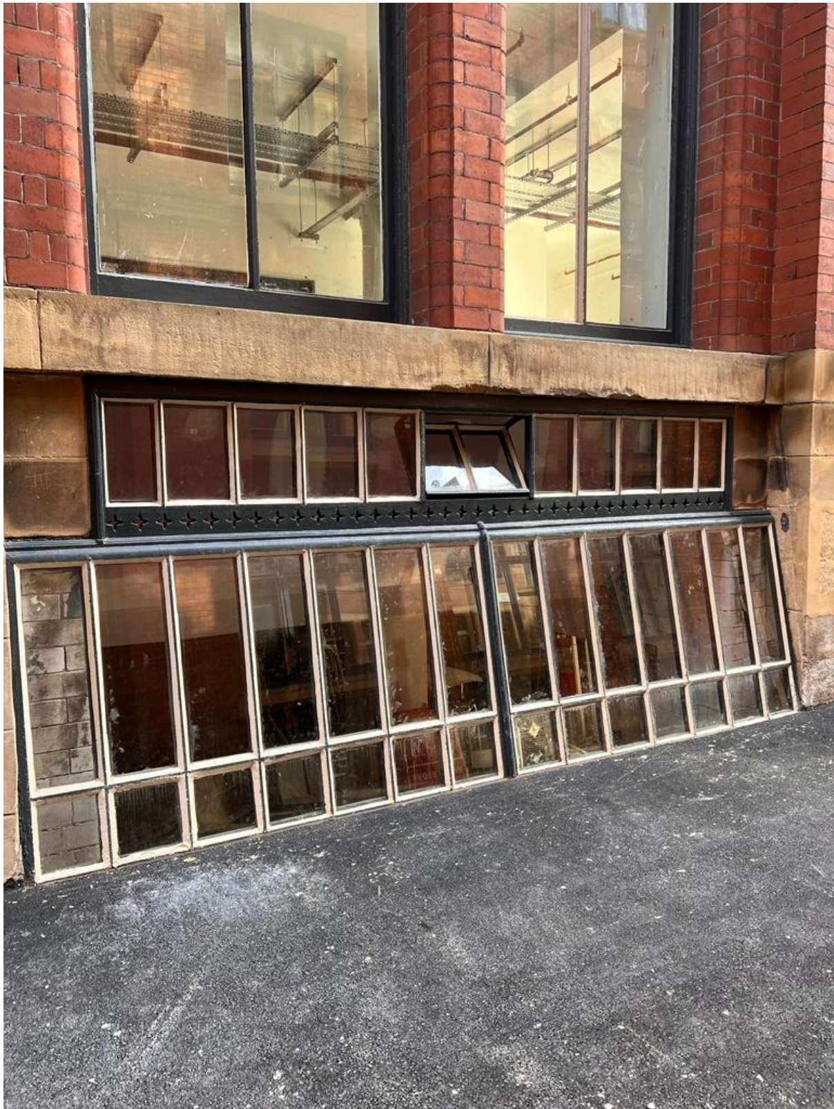
Figure 104: W1-10 & W1-11 (Credit CubicWorks 2023)
