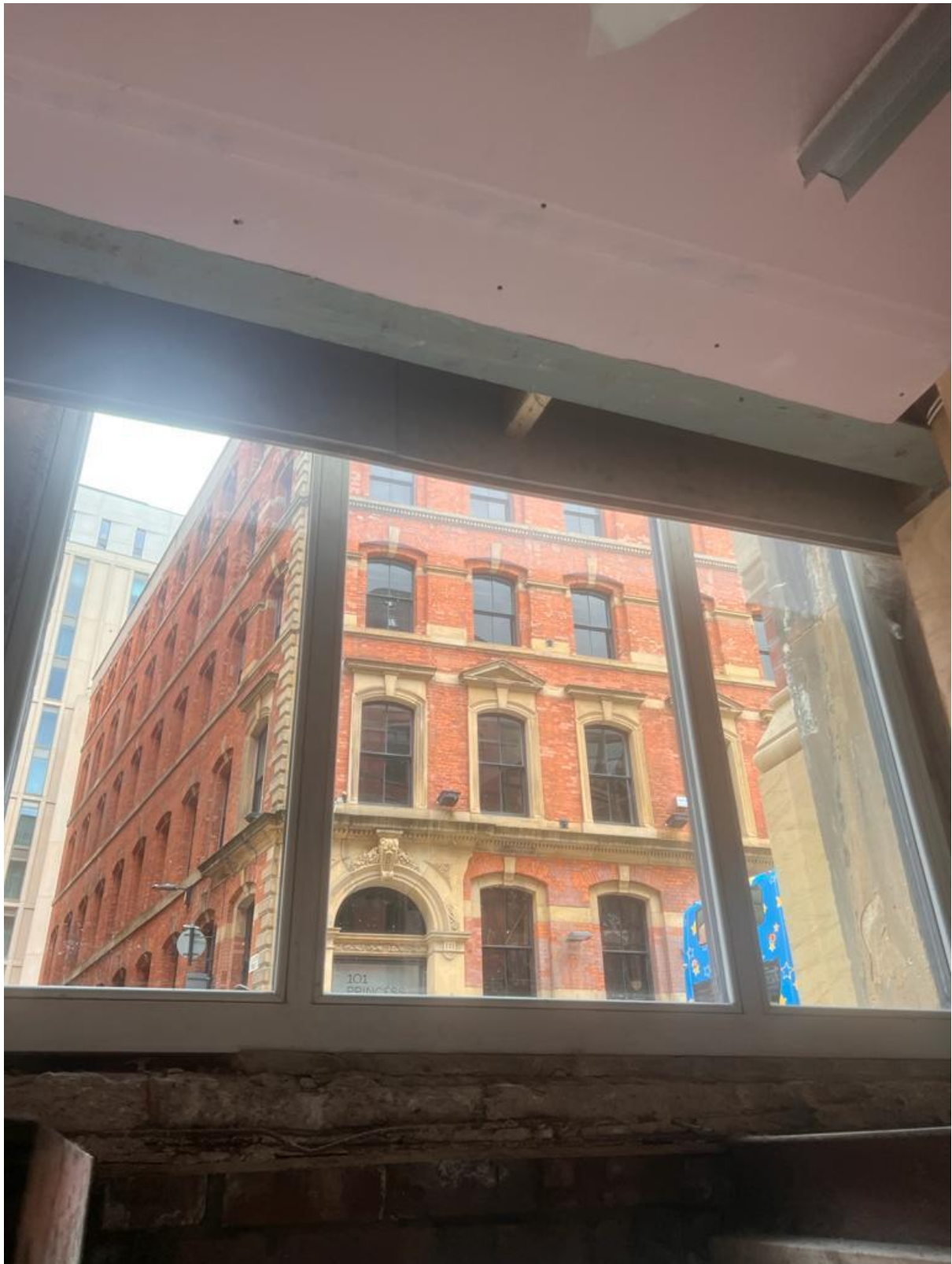
Figure 81: WP.-2.03 External (Credit CubicWorks 2023)
