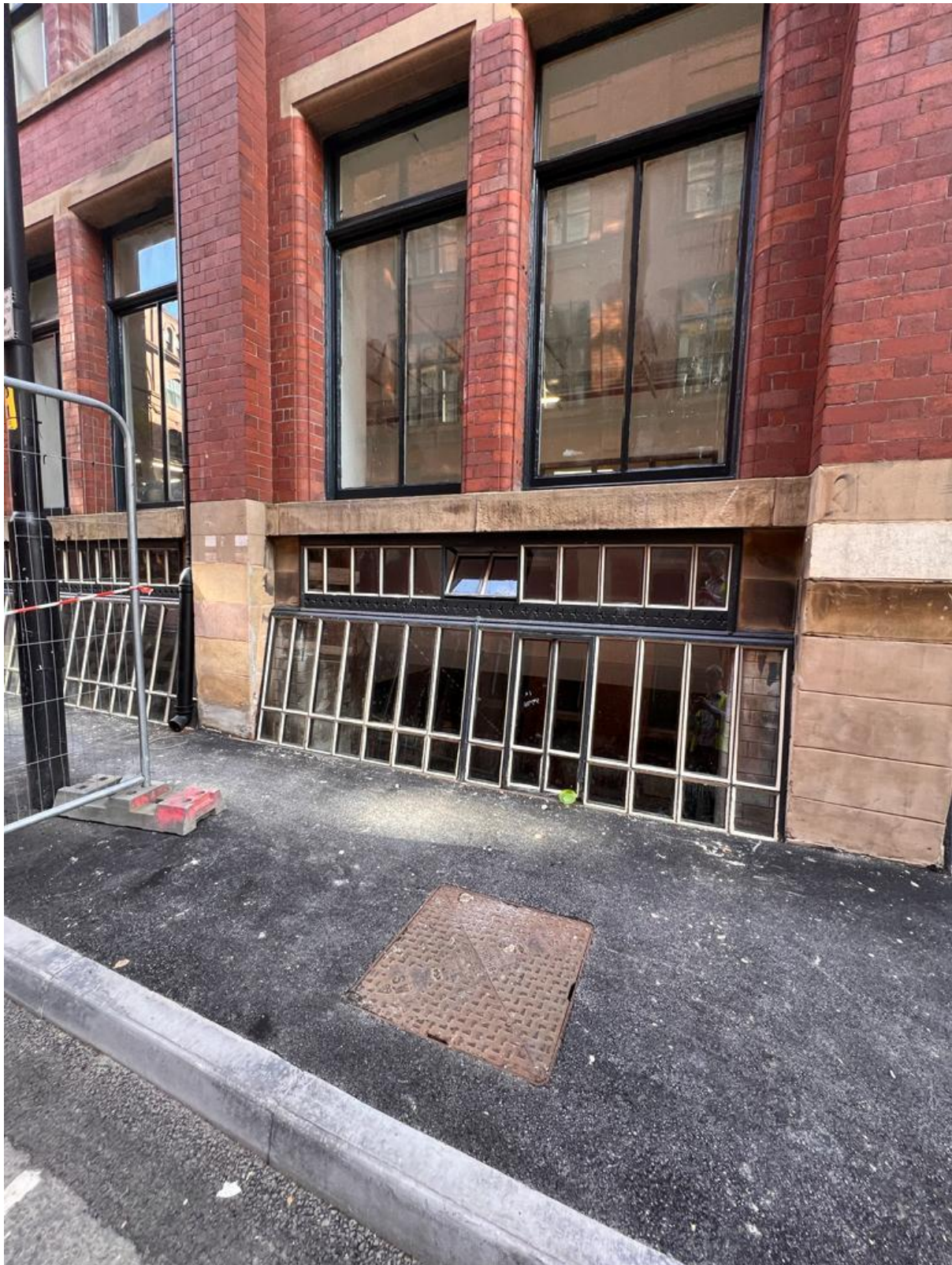
Figure 105: W1-12 & W1-13 (Credit CubicWorks 2023)
