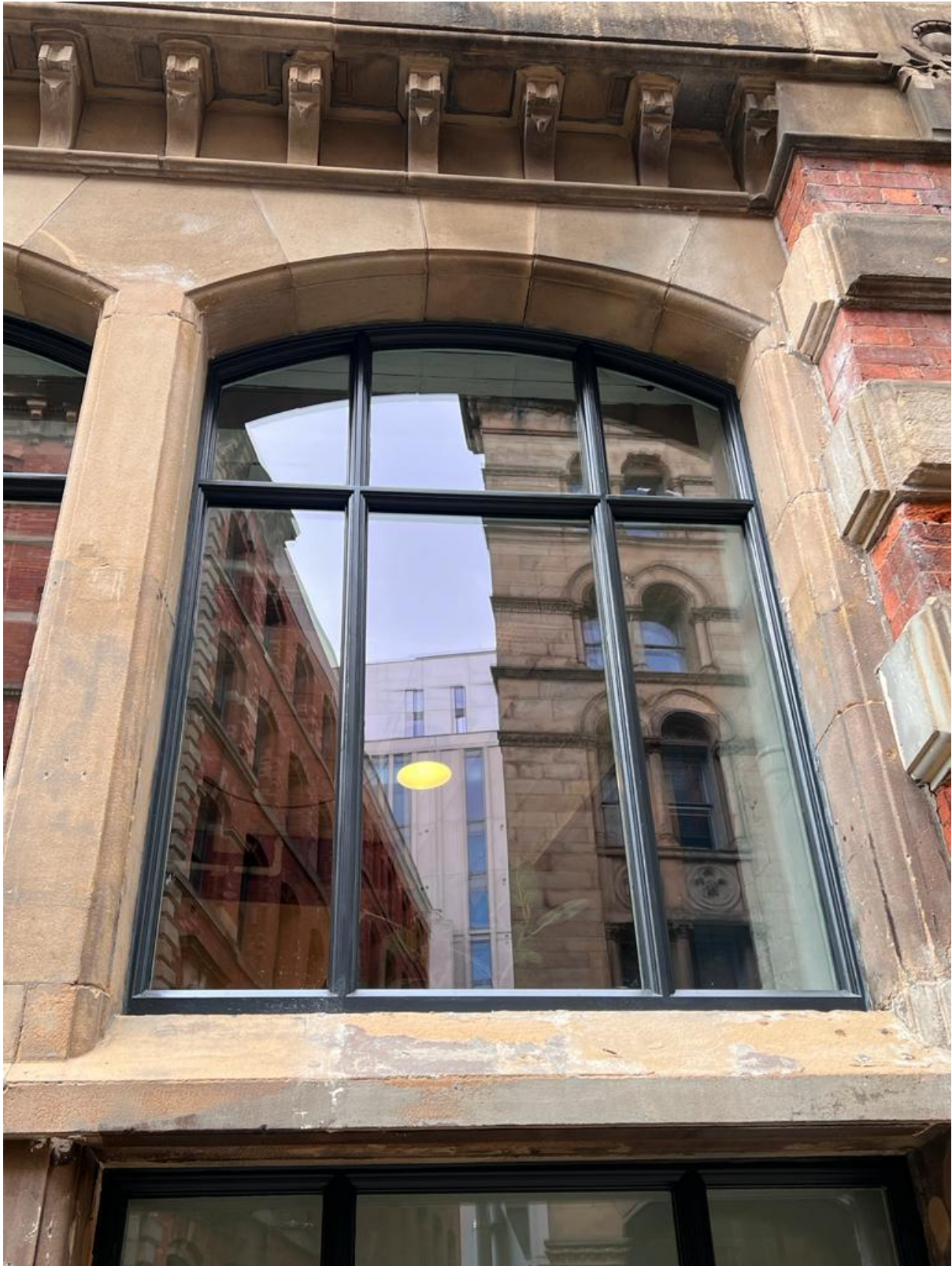
Figure 73: WP.0.06 External (Credit CubicWorks 2023)
