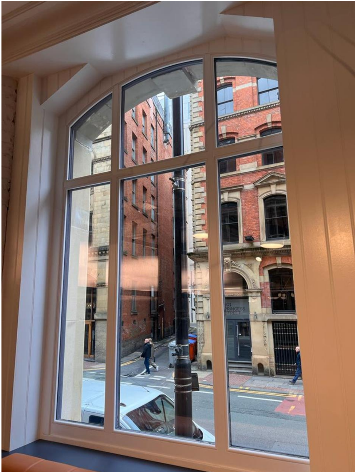
Figure 76: WP.0.02 Internal (Credit CubicWorks 2023)
