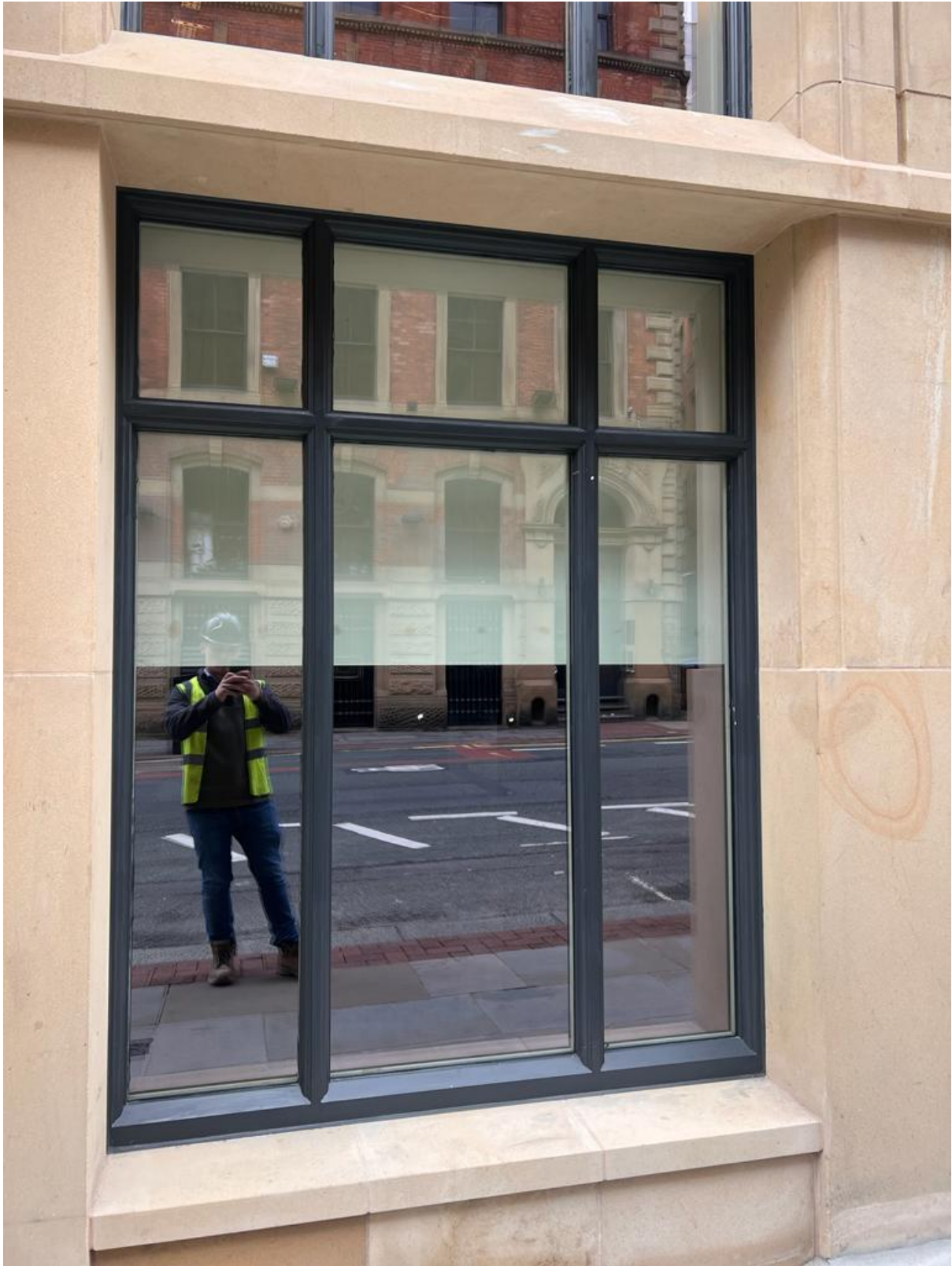
Figure 84: WP.-2.01 External (Credit CubicWorks 2023)
