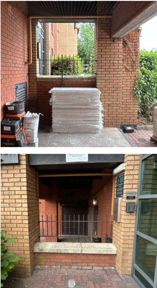
Photos showing the existing wall and railing which prevents direct pedestrian access to the ground floor commercial space from the eastern accommodation blocks. There is a finished floor level difference of approximately 1 metre.
