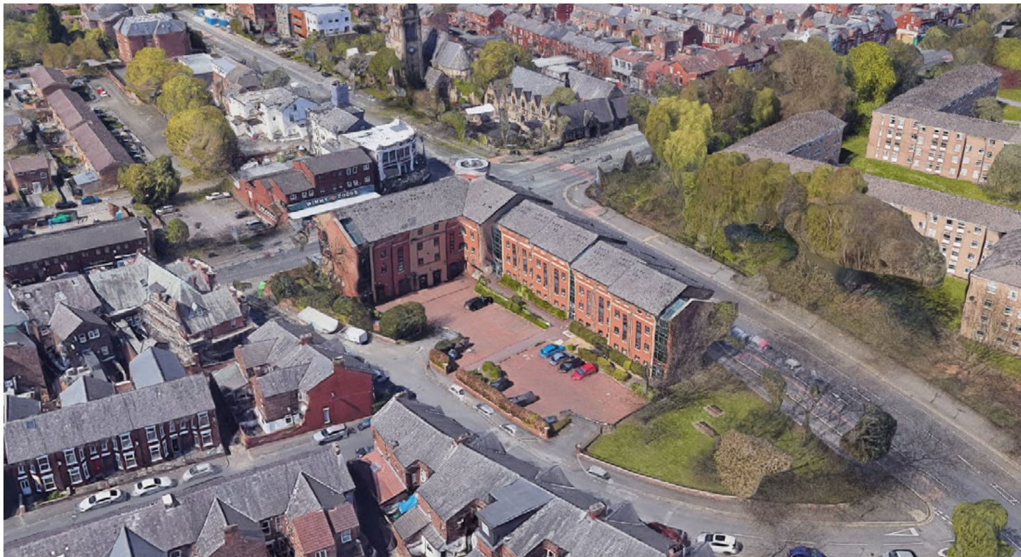
Existing aerial view from the south east
