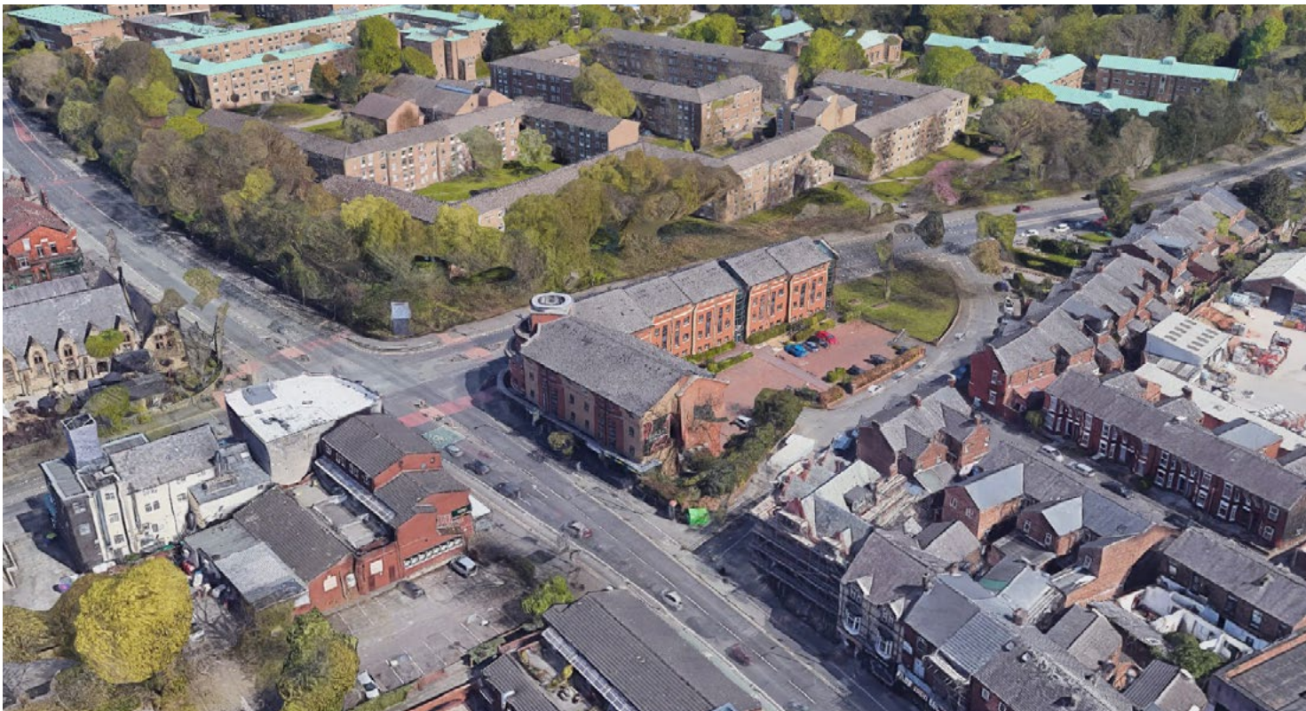
Existing aerial view from the south west
