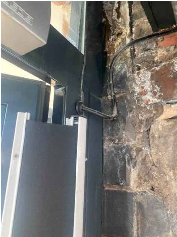
Additional work 1 of 1
