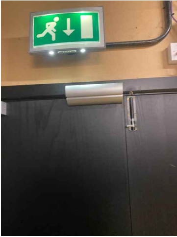
Additional work 1 of 1
