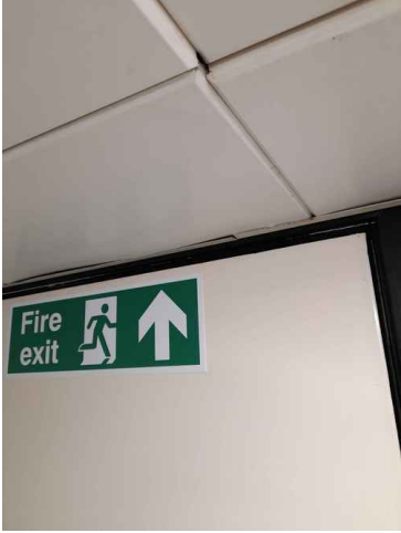
Additional work 1 of 1
