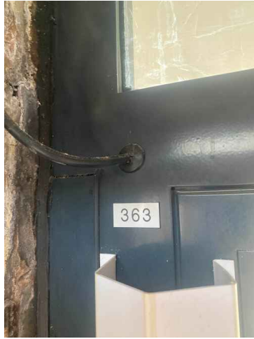
Additional work 1 of 1
