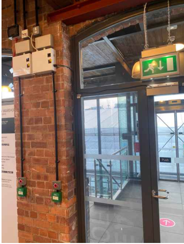
Additional work 1 of 1
