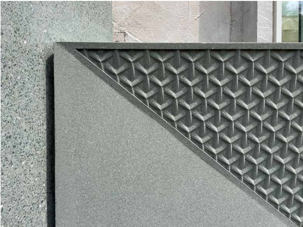
A detail of the junction between the polished pier and the acid etched horizontal panel.
