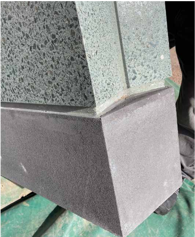
Base detail of the precast concrete columns
