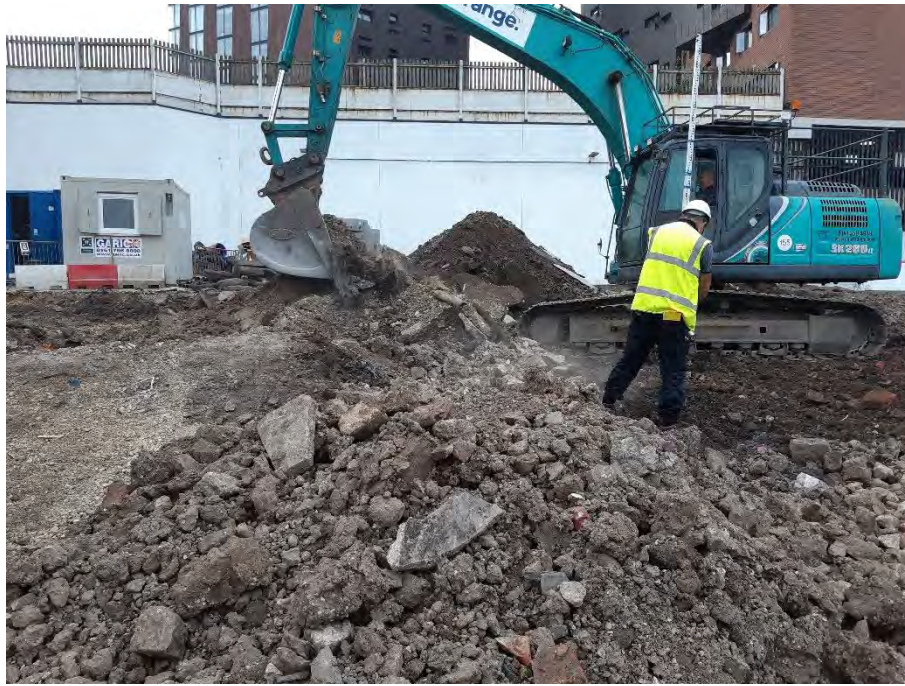
Photograph 7: reduced level dig continues in the east of the site.
