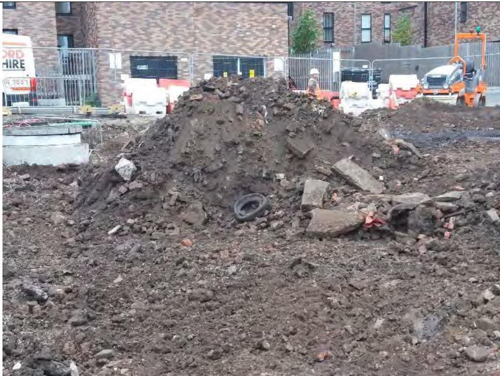
Photograph 6: Stockpiled soils containing oversize from the reduced level dig.
