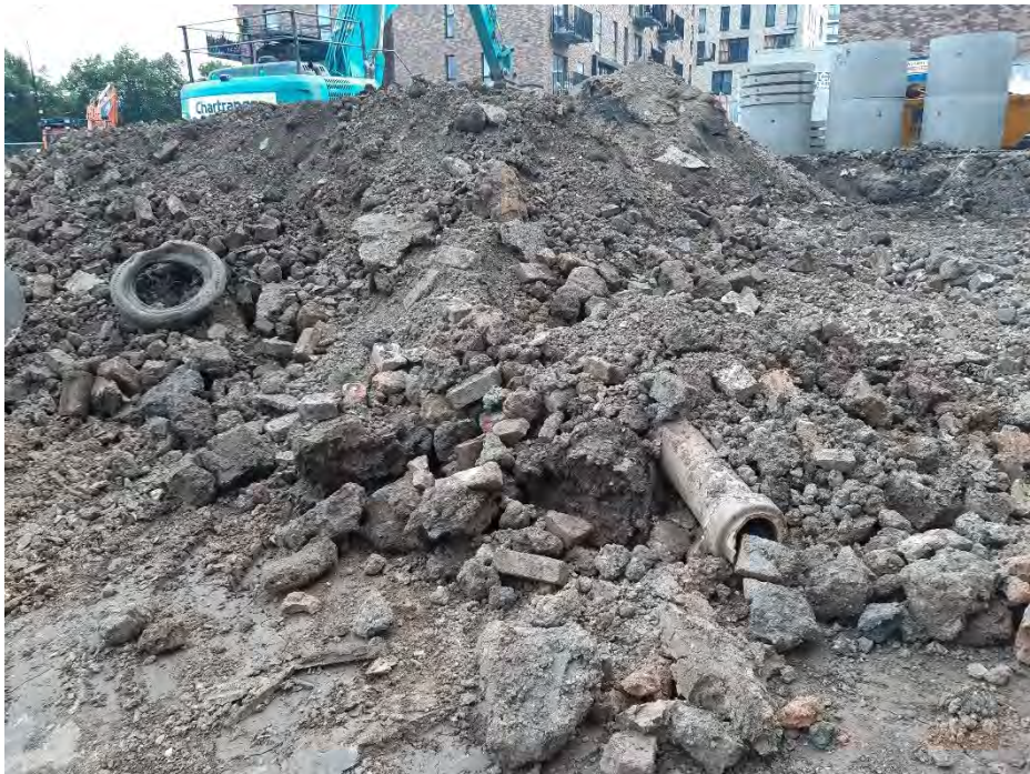
Photograph 5: Made Ground excavated from reduced level dig.
