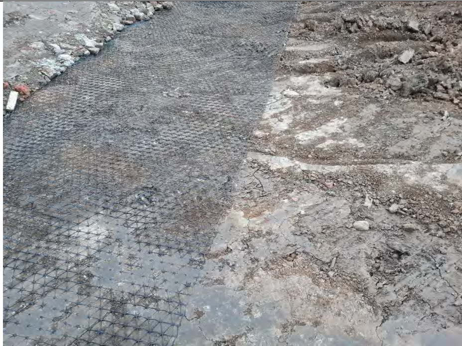
Photograph 4: Geogrid onto Glacial Till.
