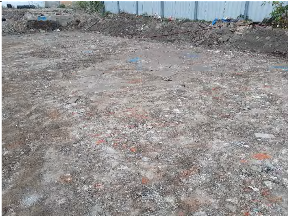
Photograph 1: Reduced level dig complete in the west of the site. Compacted 6F2 and Geogrid placed over the Glacial Till.
