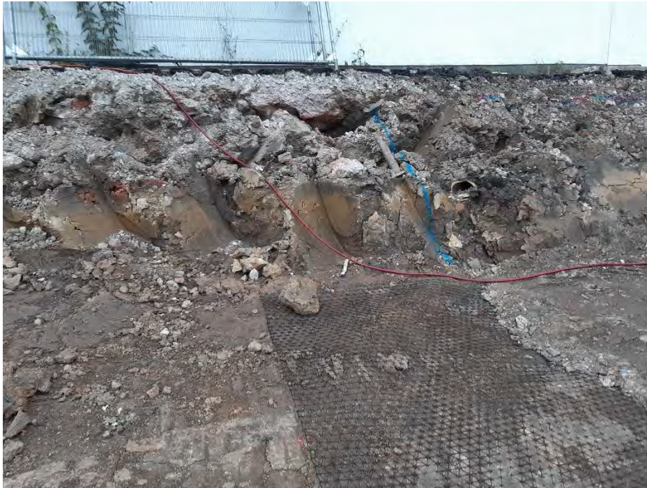
Photograph 3: Excavation side of reduced level dig and Geogrid in the west of the site
