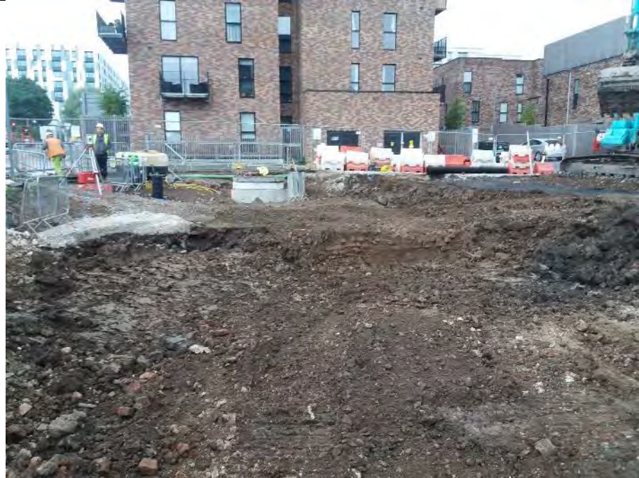
Photograph 1: Reduced level dig being undertaken in the north east of the site.
