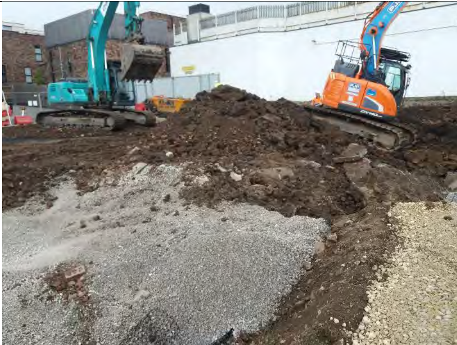
Photograph 2: Remaining soils from the final hotspot excavation.
