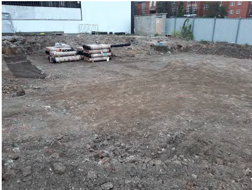
Photograph 1: Reduced level dig complete in the west of the site. Compacted 6F2 and Geogrid placed over the Glacial Till.
