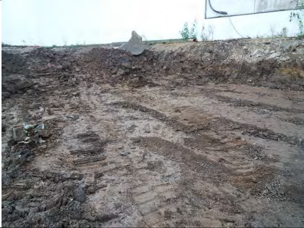
Photograph 3: Natural clay proven at formation level adjacent to the eastern boundary.
