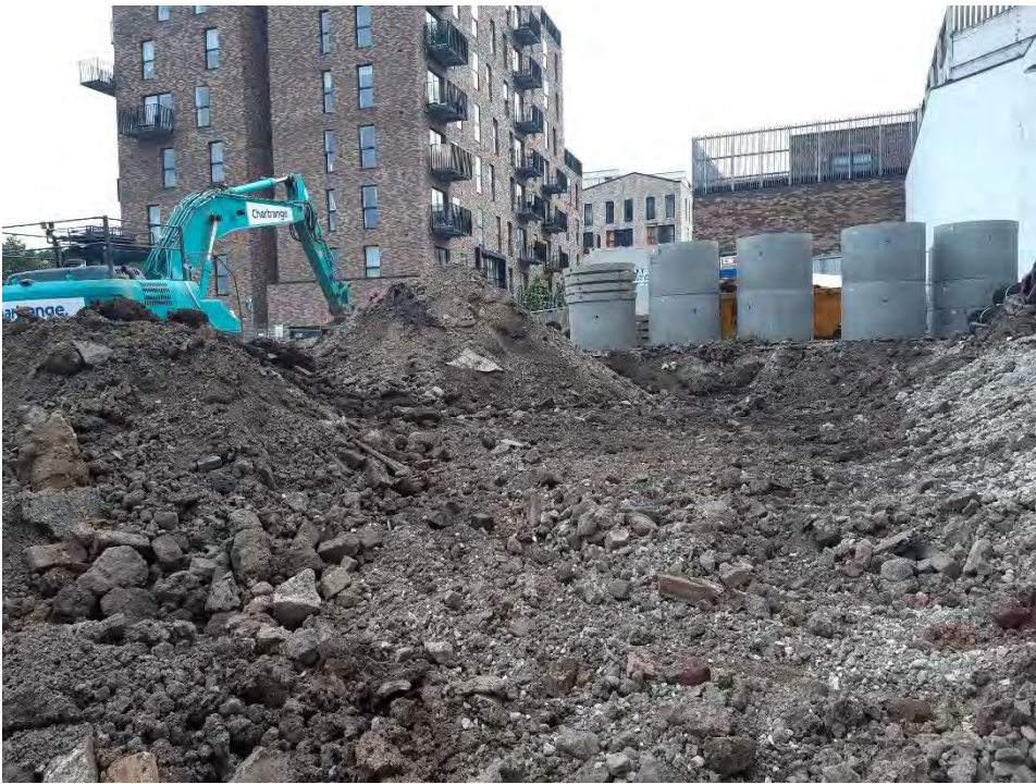
Photograph 6: Stockpiled Made Ground from the reduced level dig.
