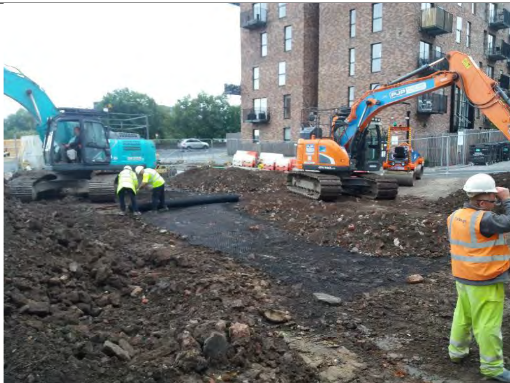
Photograph 4: Placing geogrid in the north east of the site.
