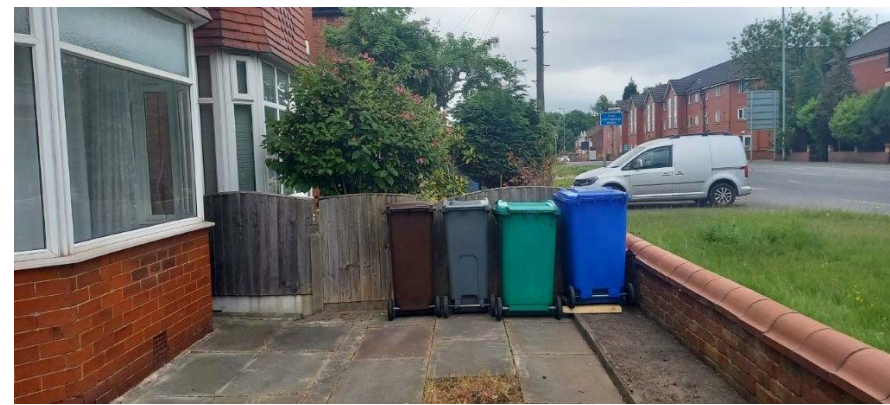
Existing Bin storage area retained
