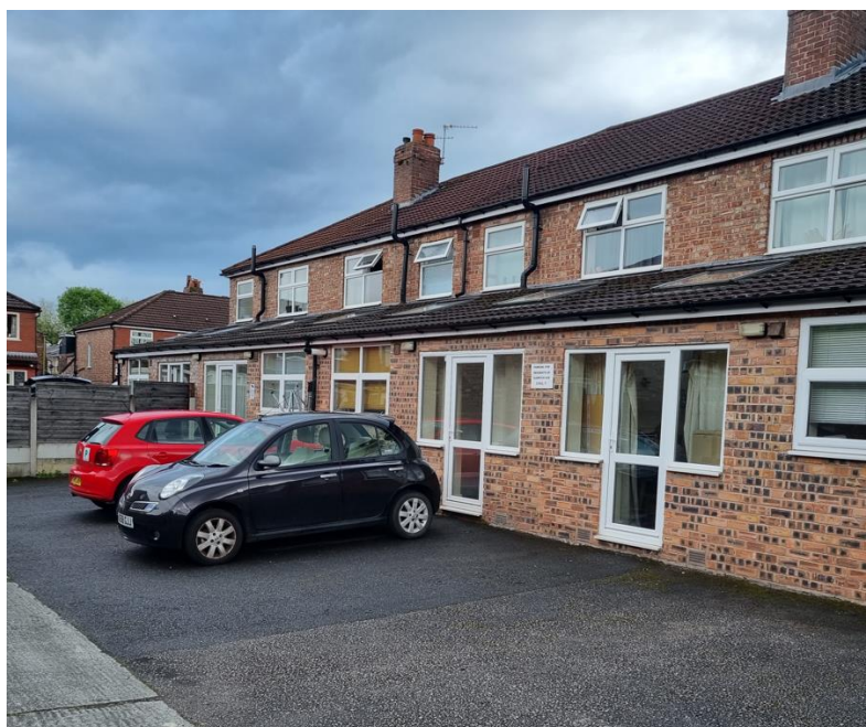
Photo 01 (Taken on site dated 10/05/2023)
