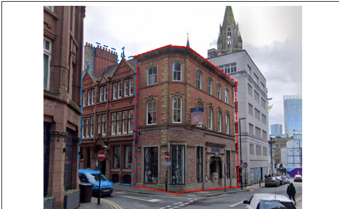
Figure 1 – The Site, looking south-west from the junction of Pall Mall and Clarence Street. No.1 Clarence Street is outlined in red and No.10 Kennedy Street is outlined in blue.
