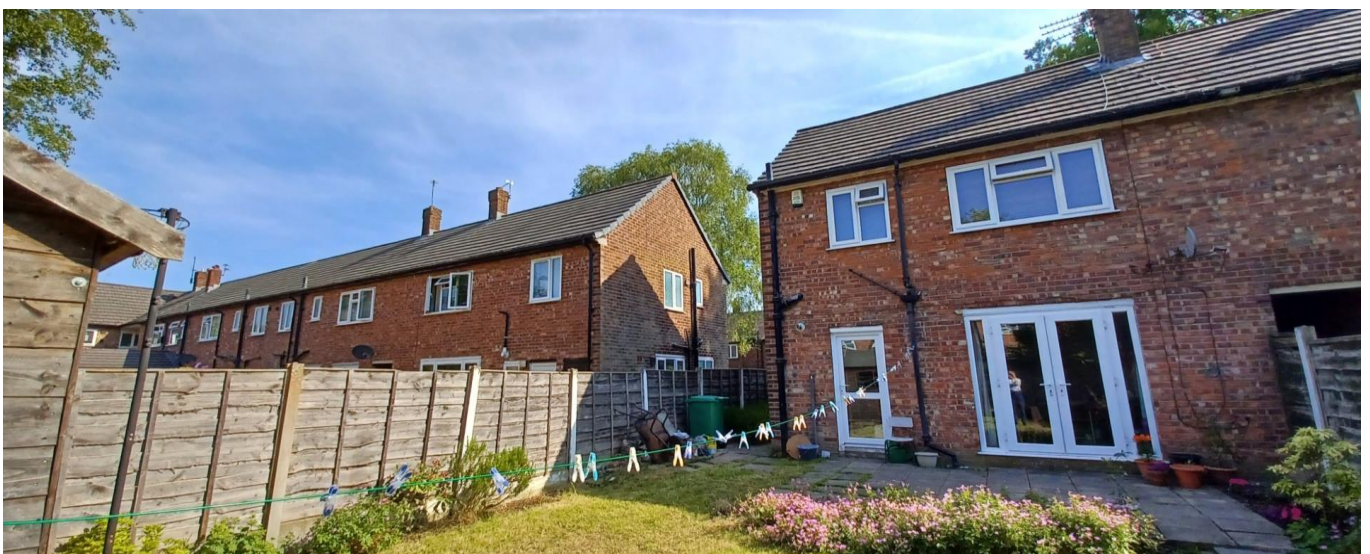
Figure 4. Boundary shared with No.10 Danbury Walk.
