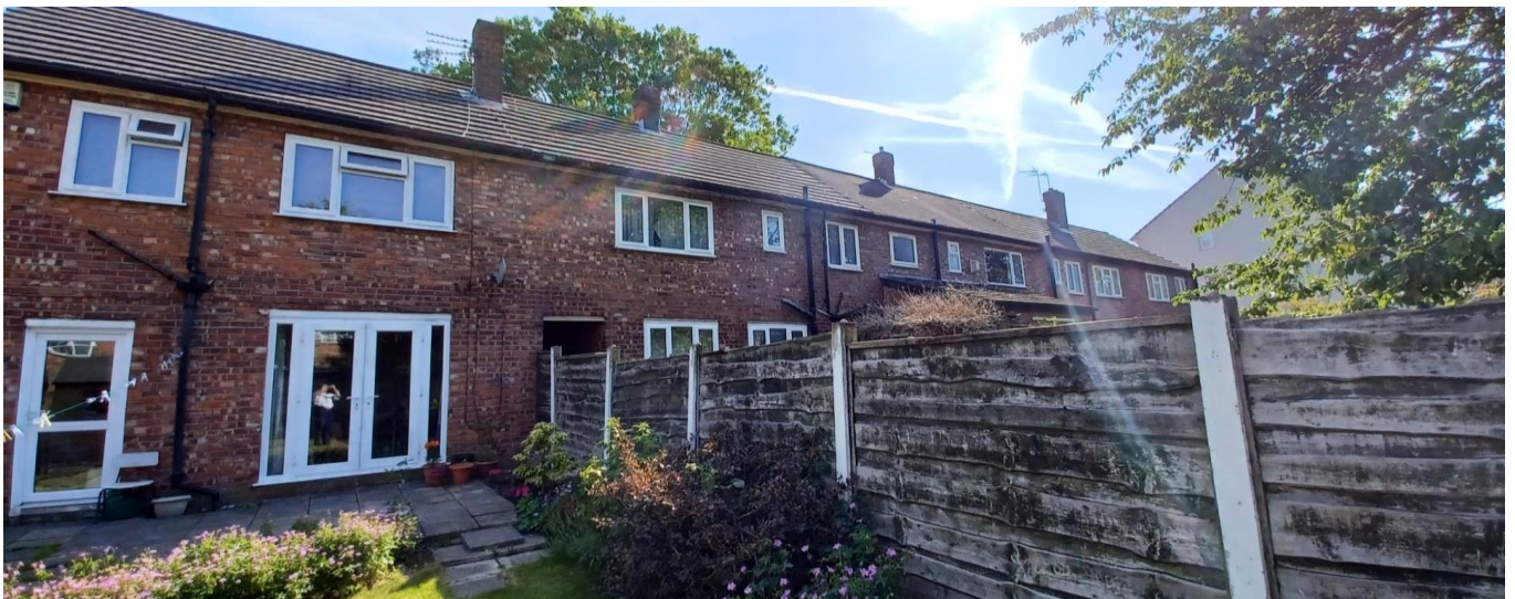
Figure 3. Boundary shared with No.14 Danbury Walk.
