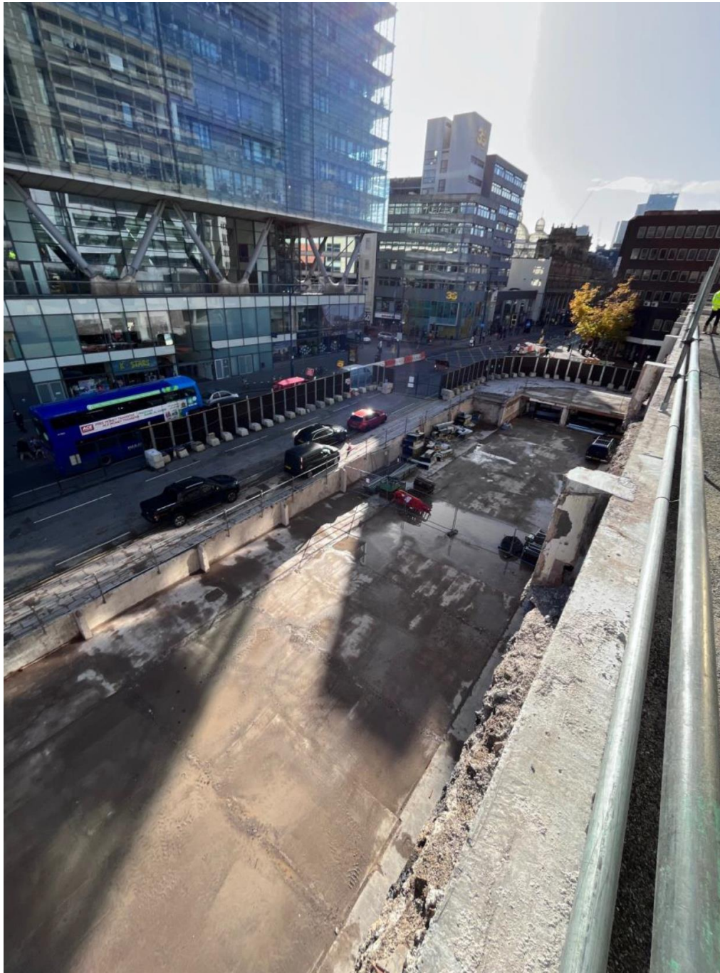
Arial View of Premier House Post Demolition, Looking South Towards Deansgate / Blackfriars
