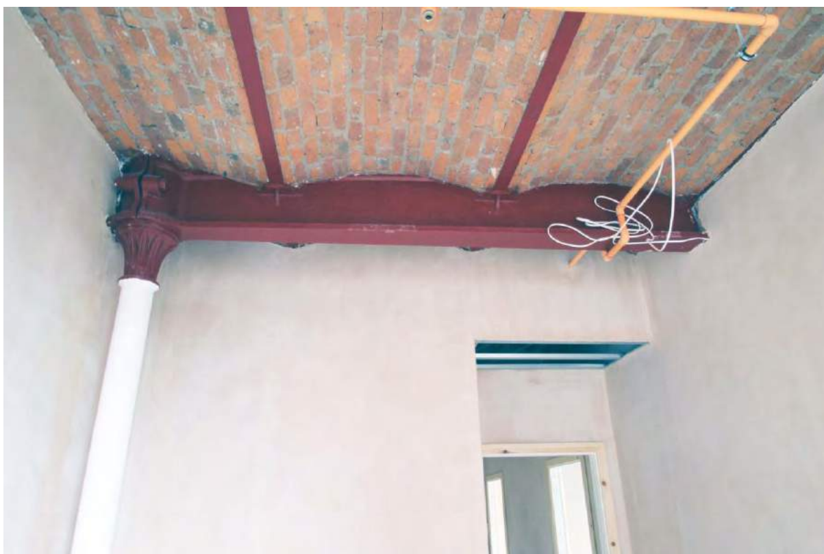
Plate 40. 'A' Mill, fourth floor, column and beam arrangement.
