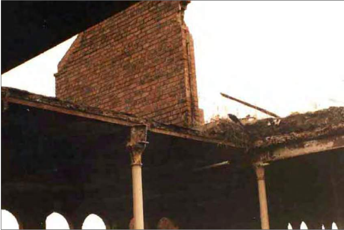
Figure 26: North-east mill ('A' Mill), fifth floor ceiling and gable of humidifying shed, c 1980s (AHP 2006).
