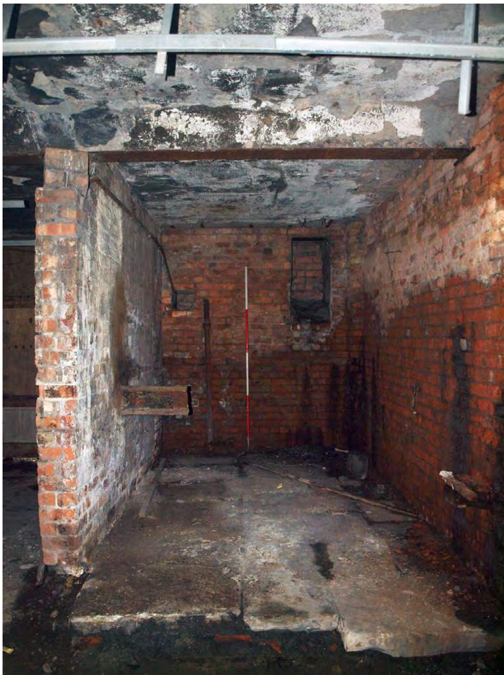
Plate 28. 'B' Mill, basement, small room in north-east corner, viewed from south-east (by S. Price).
