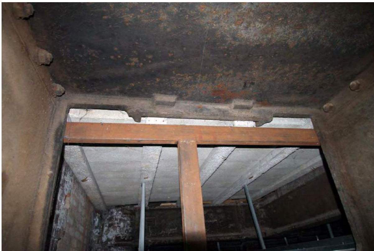
Plate 38. 'A' Mill, first floor, interior of upper part of large cast-iron wallbox, viewed from north-west.
