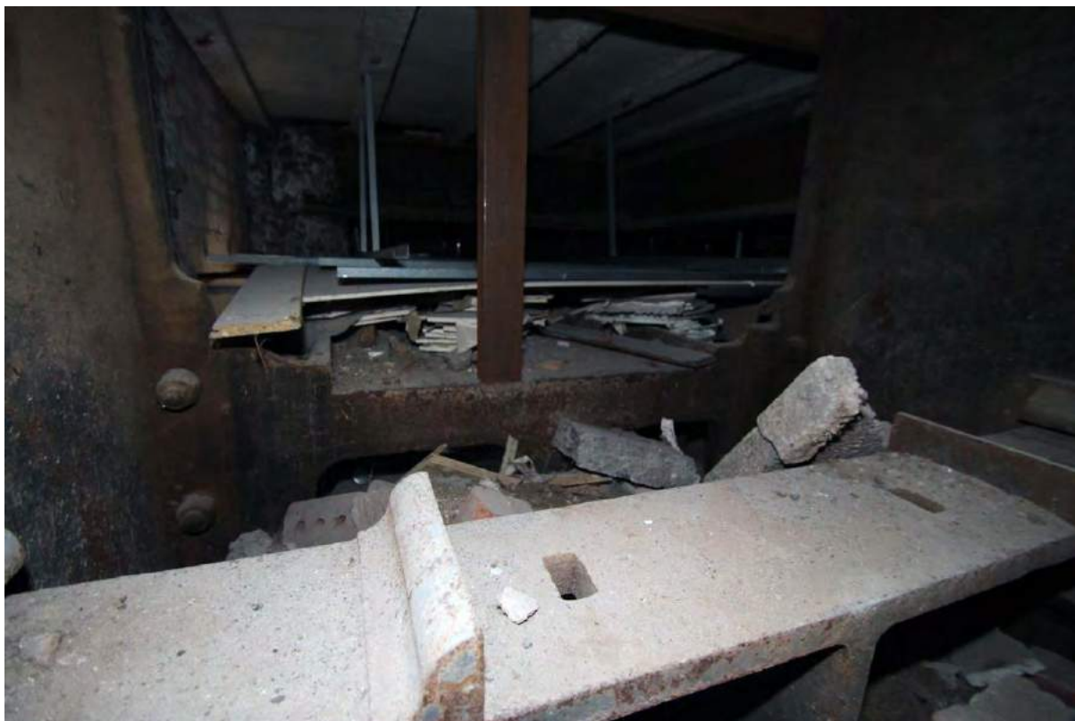
Plate 37. 'A' Mill, first floor, interior of lower part of large cast-iron wallbox, viewed from north-west.
