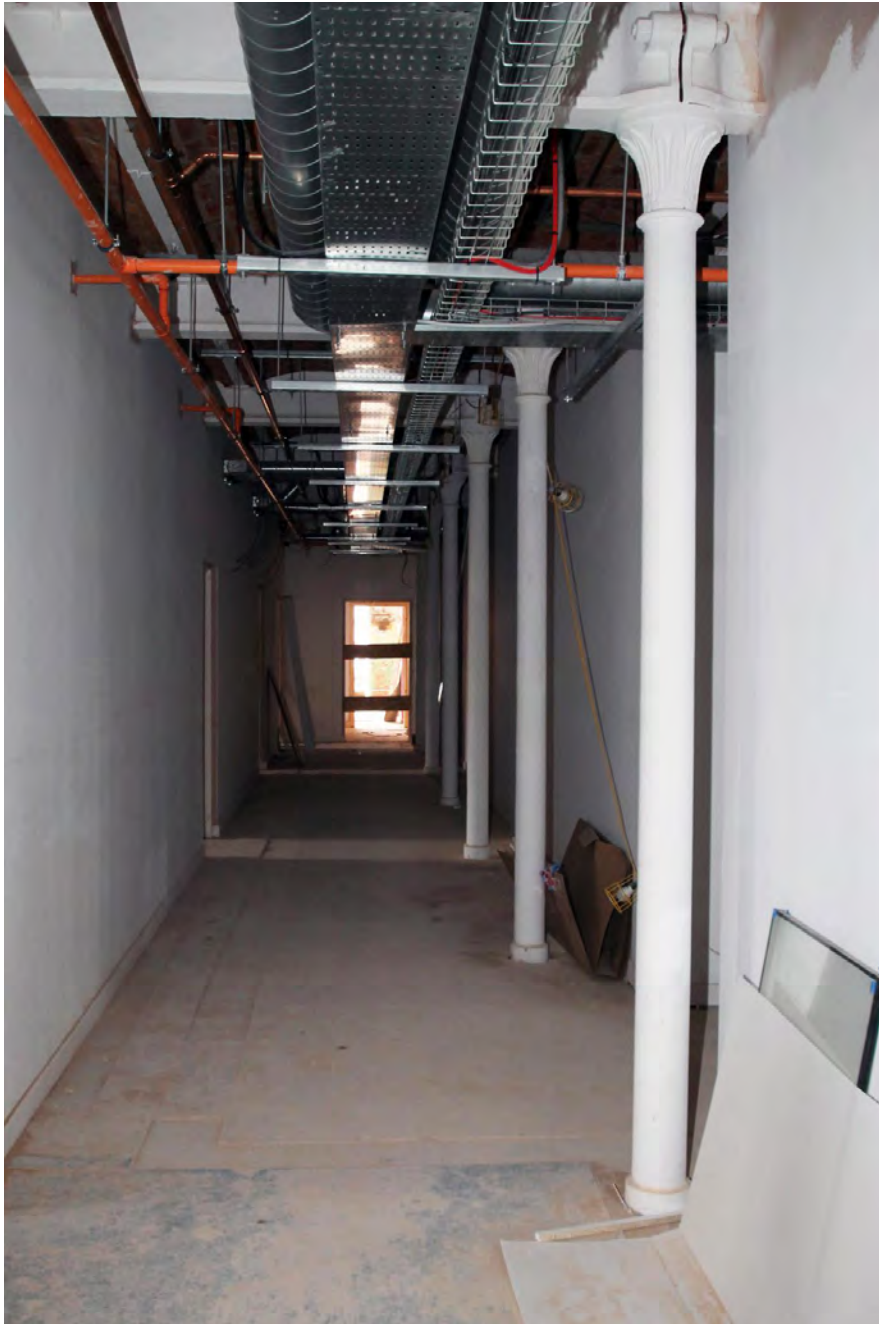
Plate 44. 'A' Mill, fourth floor, second run of columns counting from south-east.
