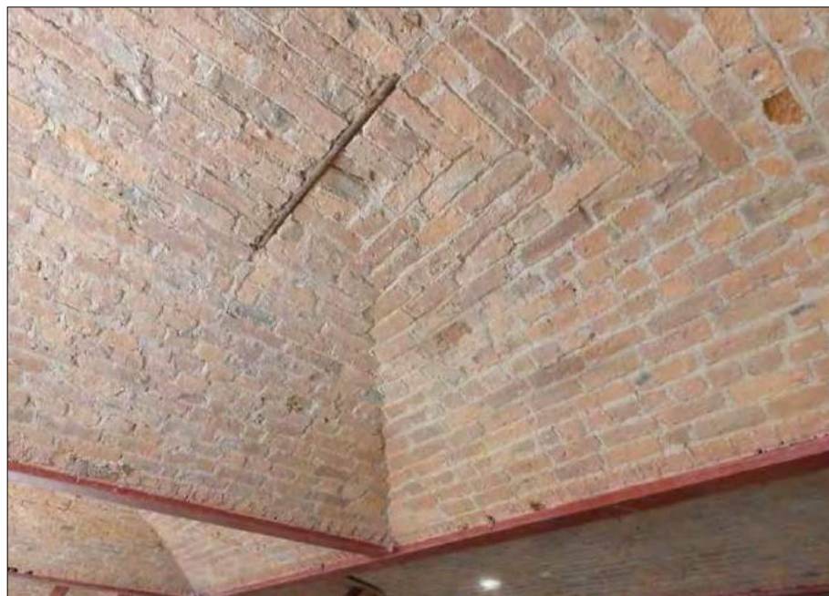
Figure 28: North-east mill ('A' Mill), detail of basement ceiling, 2016 (ARS).
