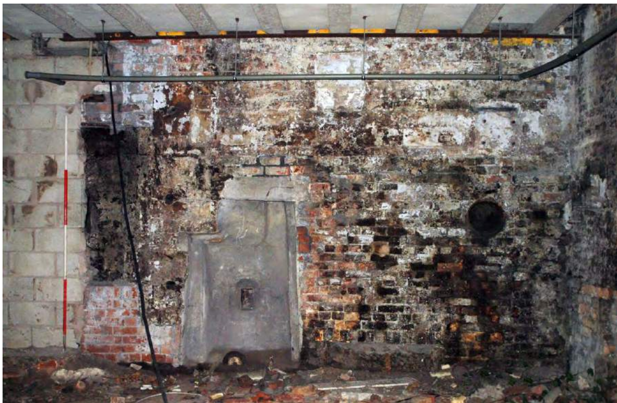
Plate 29. Central block, basement, probable south-west face of 'A' Mill beam engine bed, viewed from south-west (by S. Price).
