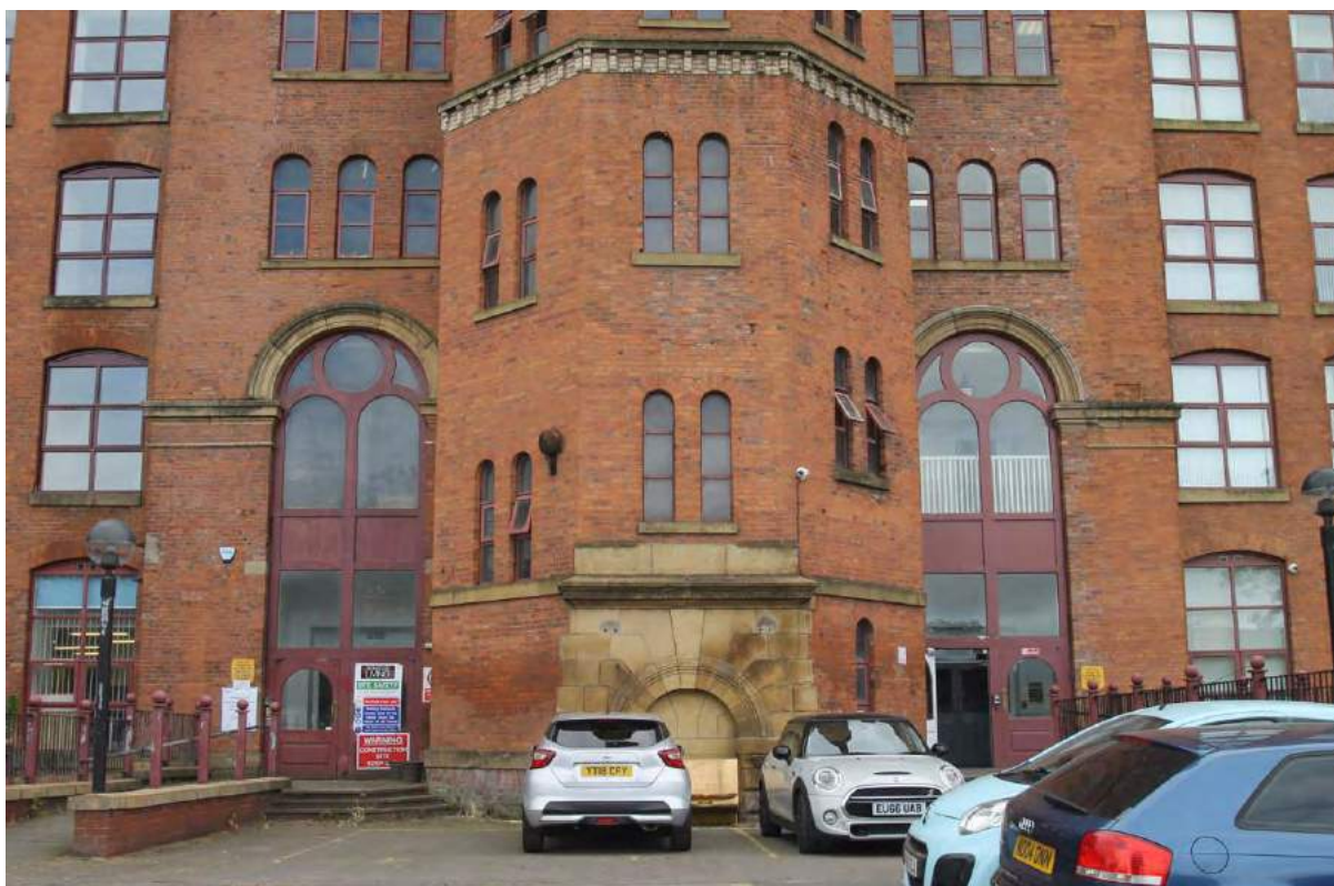
Plate 2. Base of stair tower, viewed from north-west.
