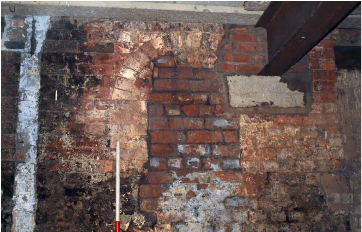
Plate 31. Central block, basement, south-east internal wall of original beam engine house, later within 1902 economiser chamber. Blocked arch is suggested as a flue from the 1902 boiler house, drawing hot flue gases into 1902 economiser chamber. Viewed from north-west (by S. Price).
