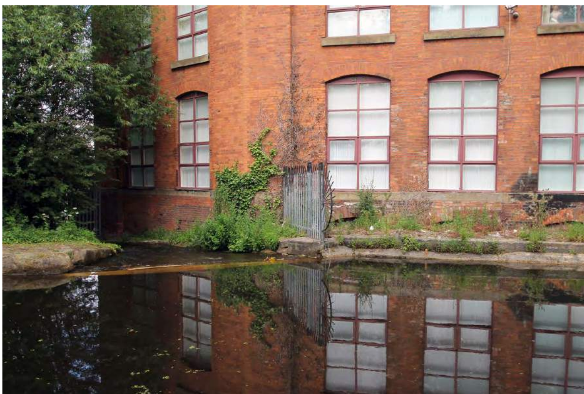
Plate 22. 'B' Mill at ground floor level, by canal byewash, note blocked arch windows which formerly illuminated the basement level. Viewed from east.
