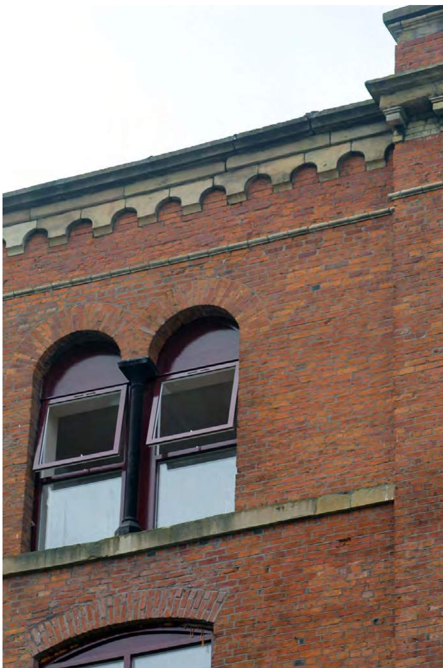
Plate 10. 'A' Mill, fifth floor windows with cast-iron column, viewed from north.
