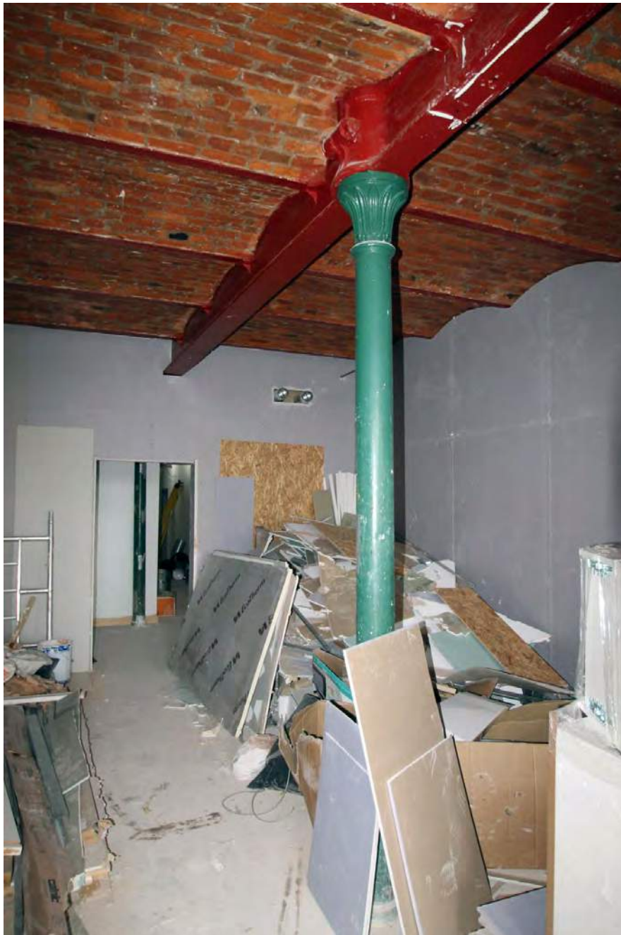
Plate 39. 'A' Mill, third floor, column and beam arrangement on north-west side.
