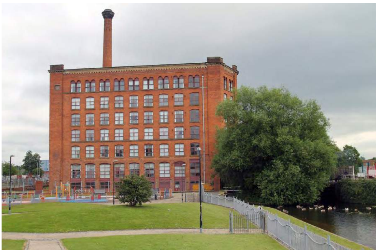
Plate 24. 'B' Mill, viewed from south-west.
