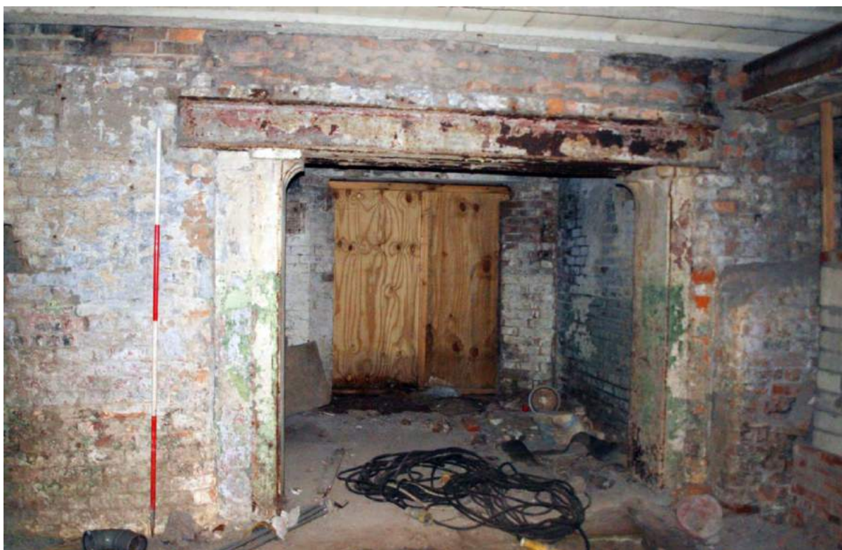
Plate 34. Central block, basement, possible original doorway between stair tower and 'B' Mill, viewed from south (by S. Price).
