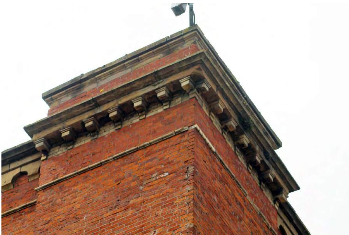
Plate 8. 'A' Mill, north-east corner tower, viewed from north.
