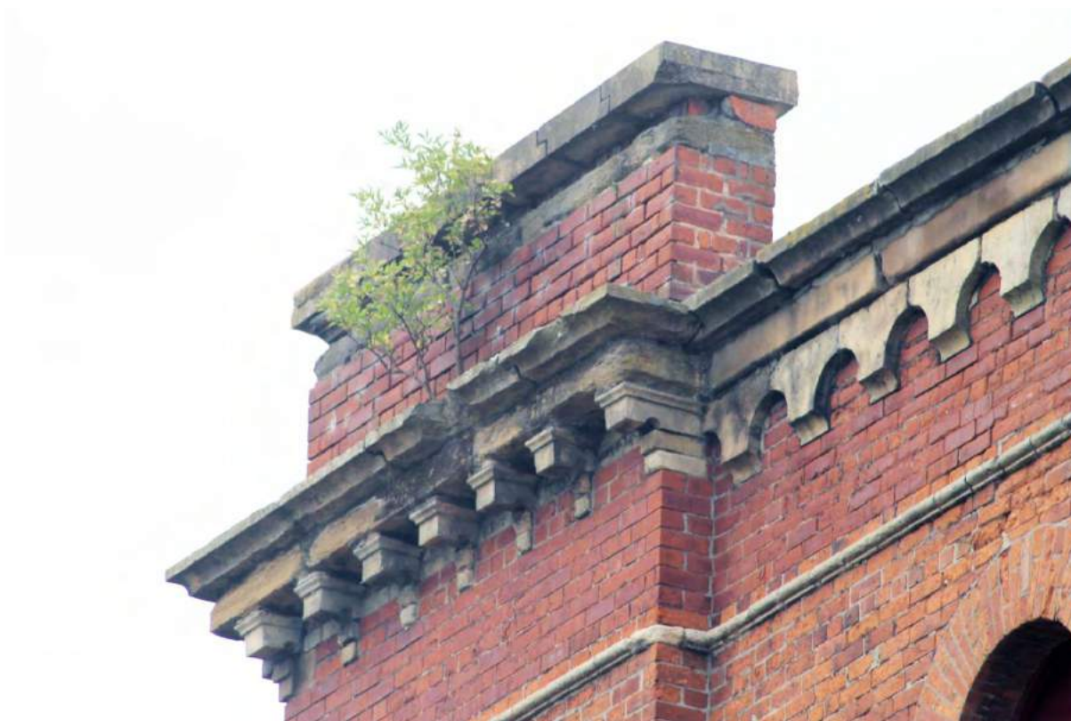
Plate 9. 'A' Mill, south-east corner turret, viewed from north.
