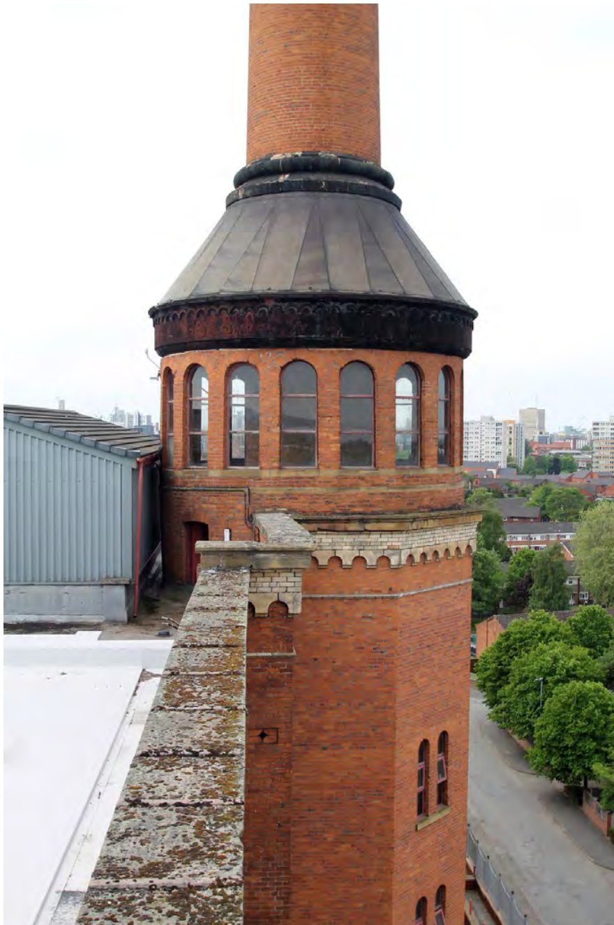
Plate 5. Gallery and water tank at top of stair tower, viewed from roof.
