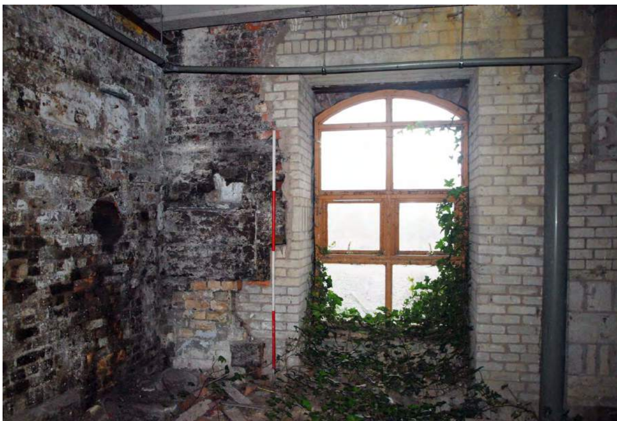
Plate 30. Central block, basement, probable south-west face of 'A' Mill beam engine bed visible to left; and external window inserted through original engine house wall, viewed from north-west (by S. Price).
