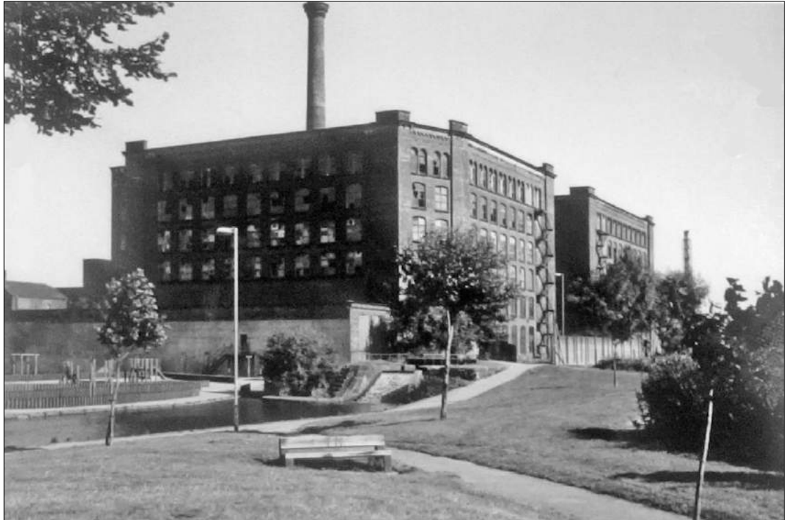
Figure 19: Victoria Mill, looking north, 1980s (Greater Manchester Textile Mill Survey).
