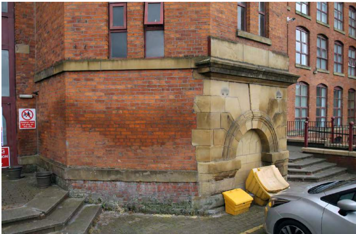
Plate 3. Close-up view of stair tower base, viewed from north.
