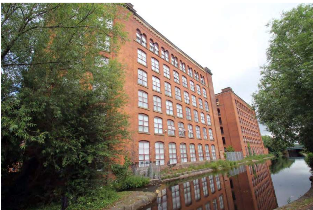
Plate 21. Mill south-east elevation, viewed from south. Note canted section of wall on 'B' Mill, to left.
