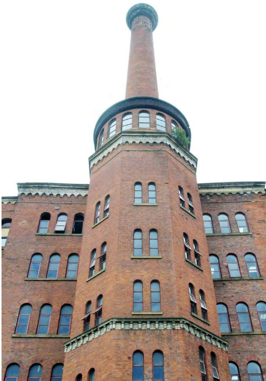
Plate 4. Upper part of stair tower and chimney stack, viewed from north-west.
