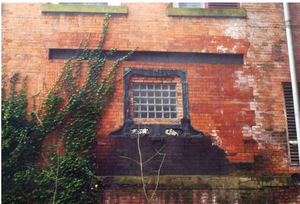
Plate 18. Courtyard, cast-iron wallbox for engine crankshaft, viewed from north-east.
