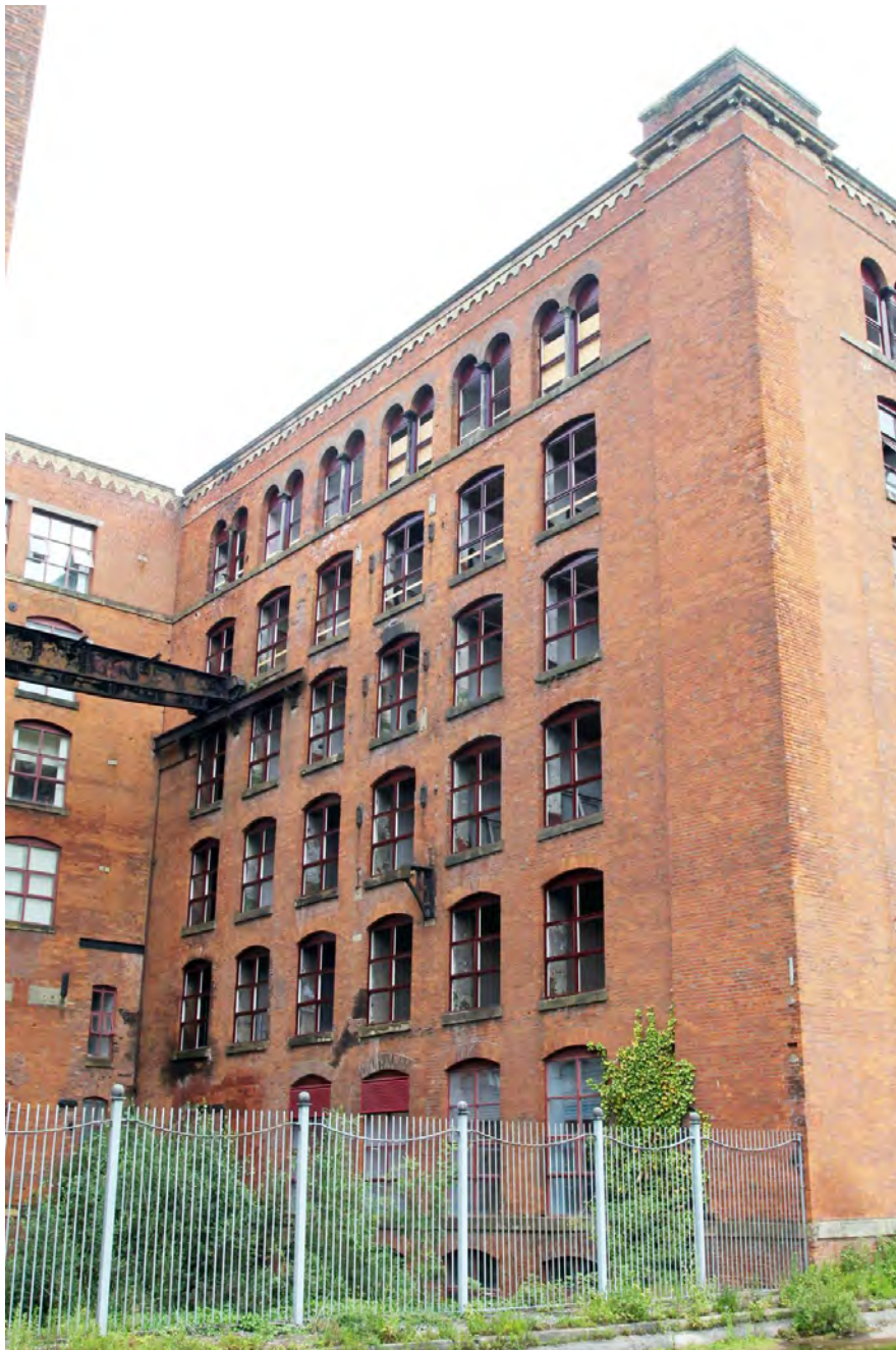
Plate 13. Courtyard, showing south-west elevation of 'A' Mill, viewed from south.
