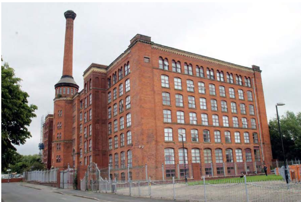
Plate 25. Mill viewed from west.
