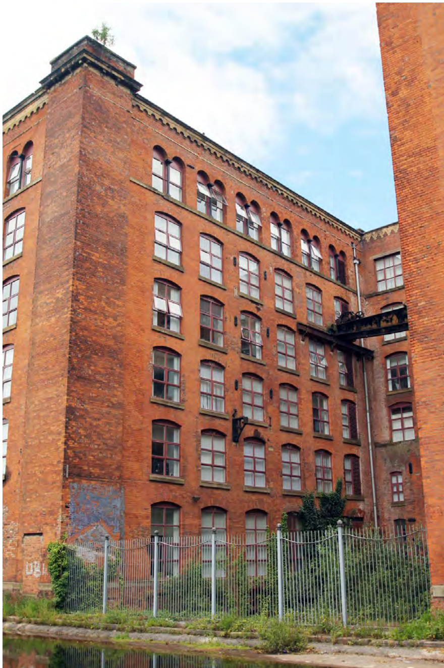
Plate 14. Courtyard, showing north-east elevation of 'B' Mill, viewed from east.
