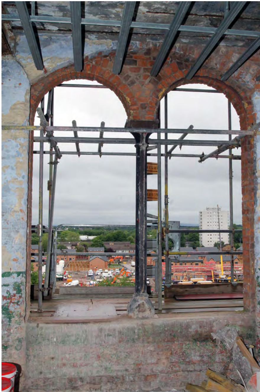
Plate 48. 'A' Mill, fifth floor, window with ornamental cast-iron post.
