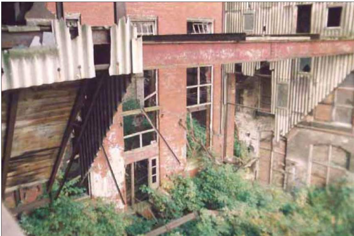
Figure 23: Detail of rope race enclosures, c 1980s (AHP 2006).
