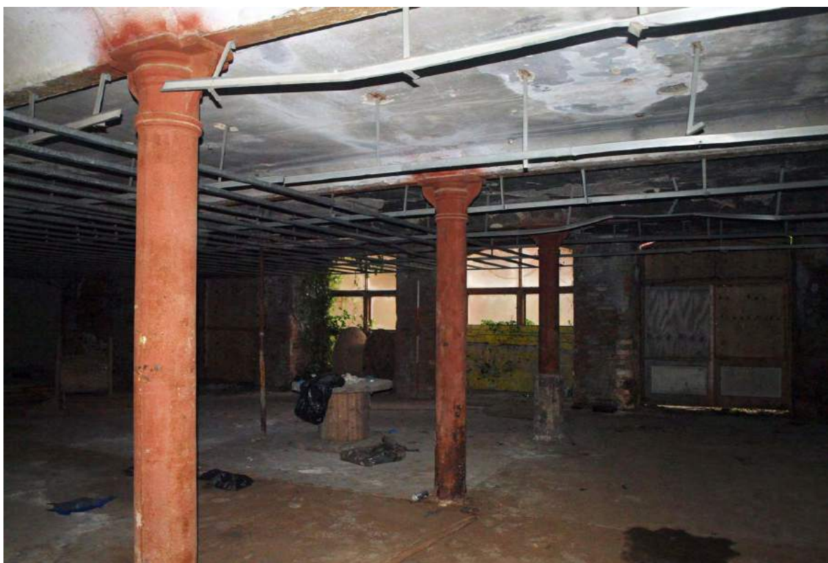
Plate 26. 'B' Mill, basement, viewed from south-west (by S. Price).
