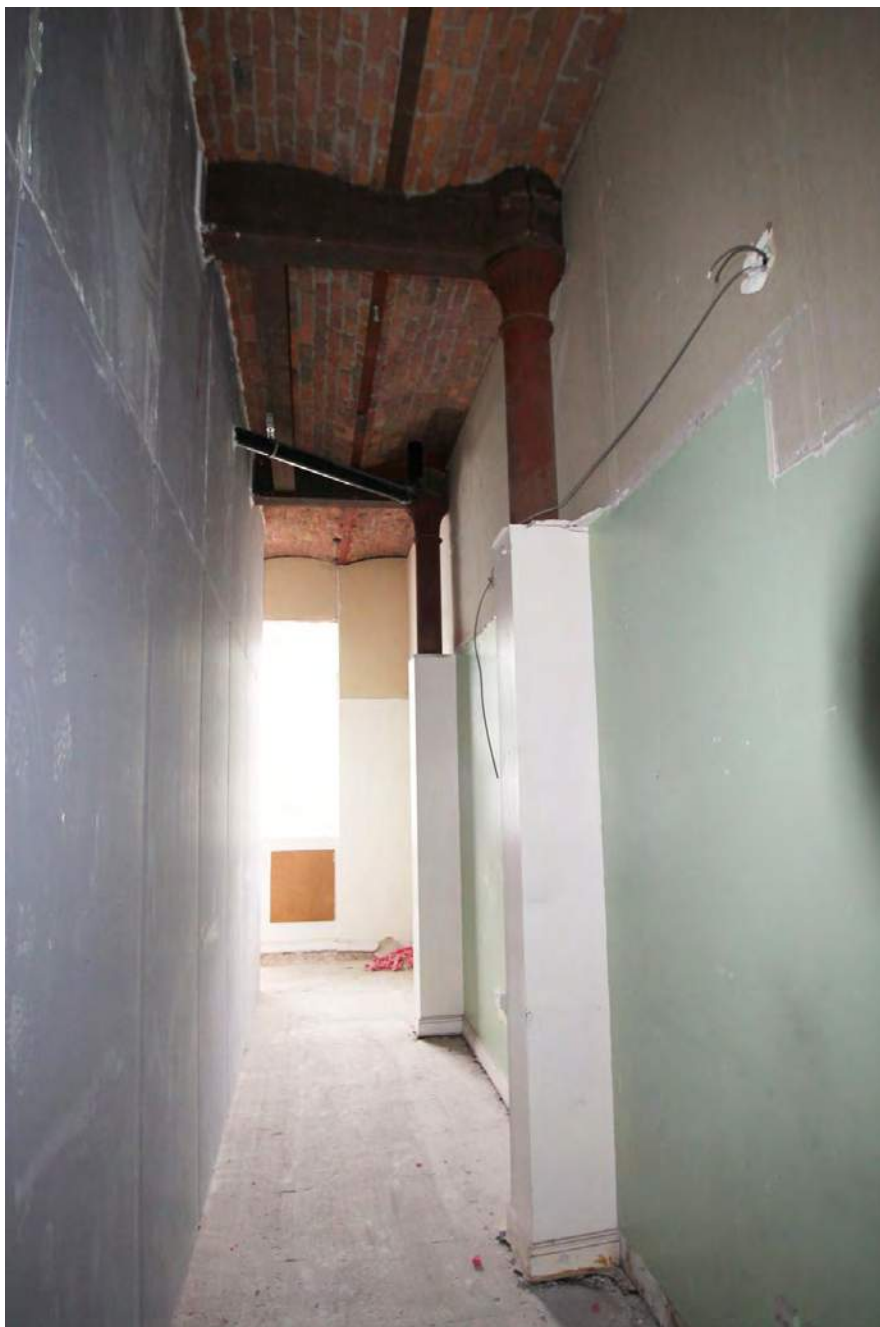
Plate 35. 'A' Mill, ground floor, cast-iron columns and beams, viewed from south-east.
