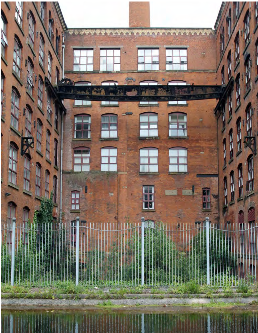
Plate 12. Central courtyard, viewed from south-east, from canal towpath.
