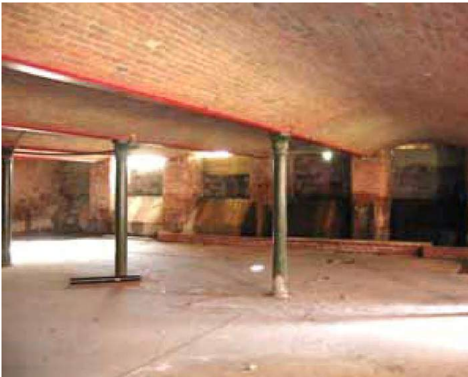
Figure 26: North-east mill ('A' Mill), basement, 2015 (AHP).
