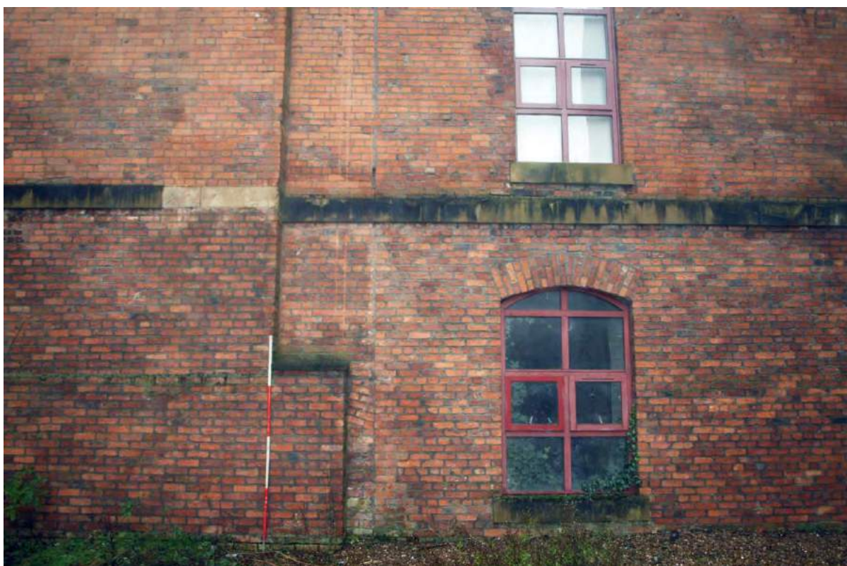
Plate 17. Courtyard, north-west wall, close-up of straight joint and offset, viewed from south-east.
