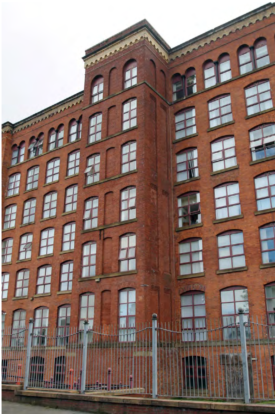
Plate 7. 'B' Mill flue tower, viewed from north-west.
