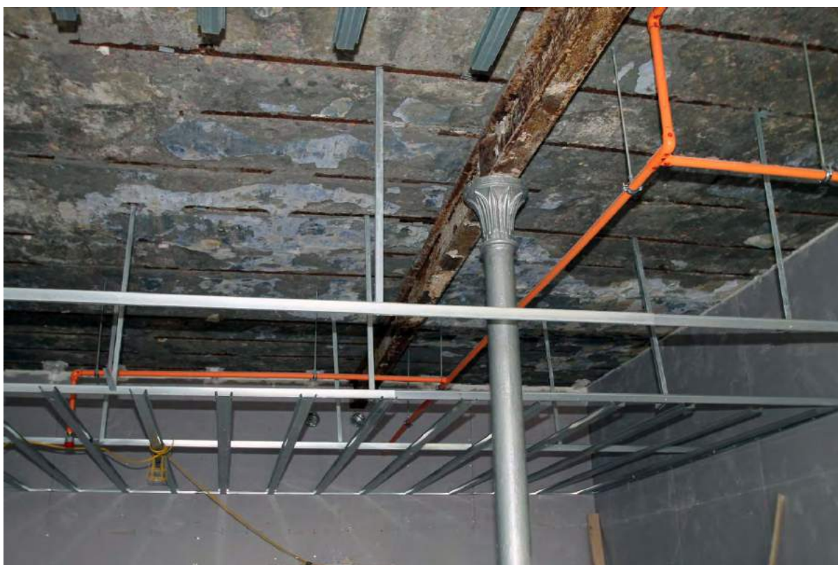
Plate 47. 'A' Mill, fifth floor, showing replacement concrete ceiling.
