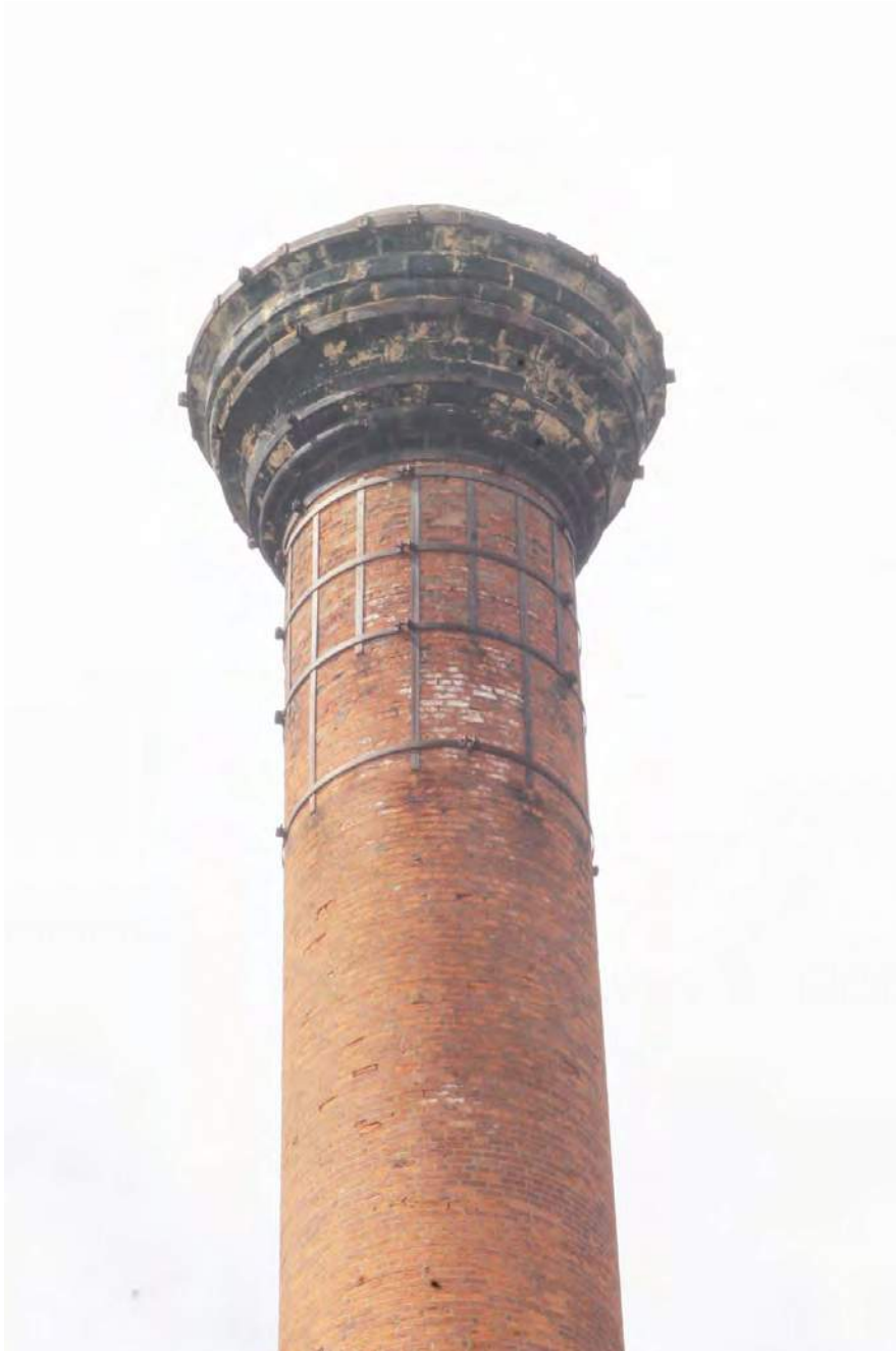
Plate 6. Top of chimney stack, showing sandstone oversailer and wrought-iron bands and straps.
