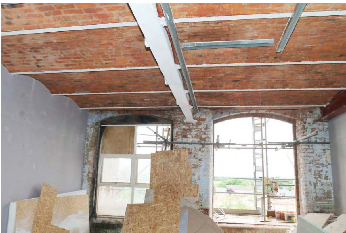
Plate 43. 'A' Mill, fourth floor, north-west side, beam arrangement and windows.
