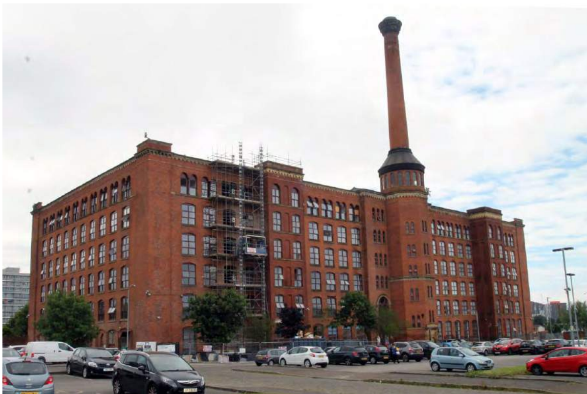
Plate 1. Mill viewed from north, from James Street.
