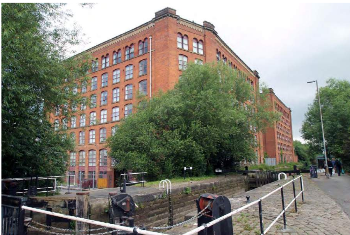
Plate 23. 'B' Mill, viewed from canal lock, from south.
