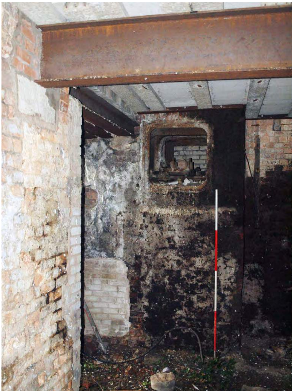
Plate 32. Central block, basement, south-east corner, showing cast iron wallbox extending into 'B' Mill, possibly taking drive from beam engine house. Viewed from north-east (by S. Price).
