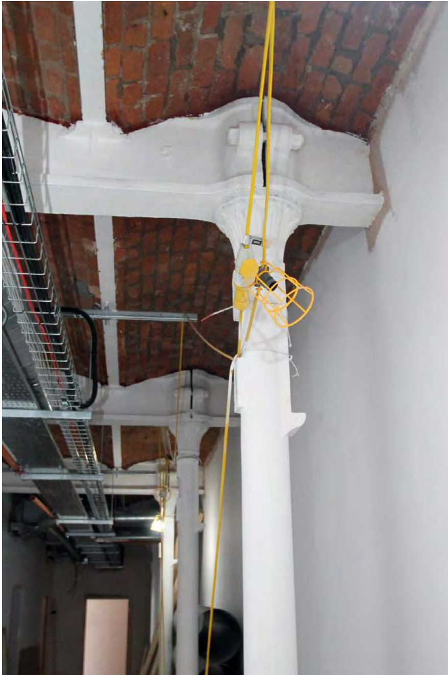
Plate 45. 'A' Mill, fourth floor, fourth run of columns counting from south-east, with integral castings for bearing boxes on right.
