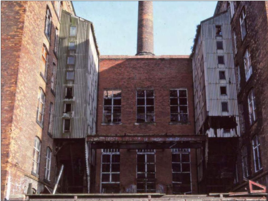
Figure 22: Victoria Mill, 1955 rope race enclosures and south-east wall of 1902 engine house, c 1980s (Greater Manchester Archaeological Advisory Service).
