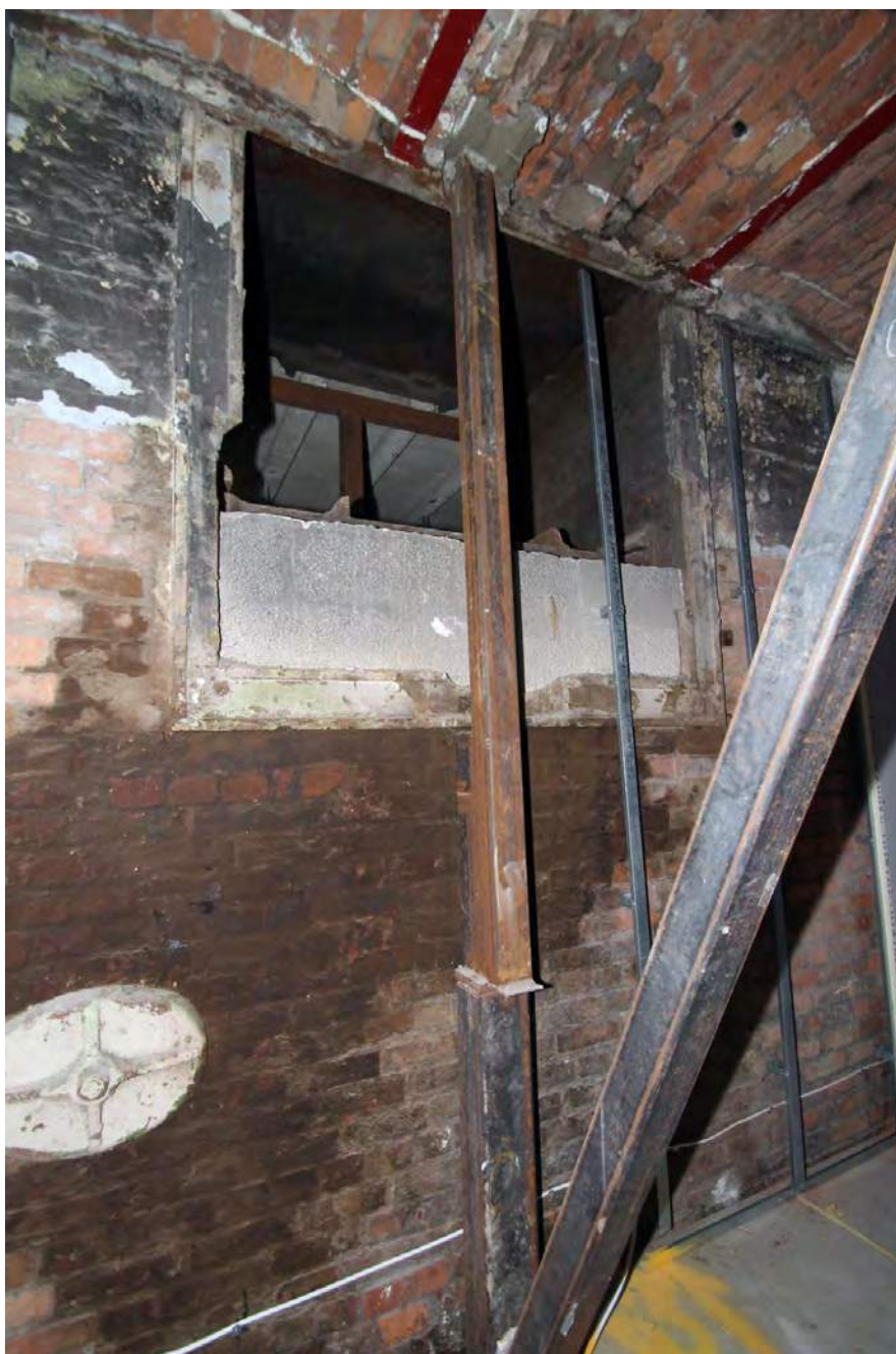
Plate 36. 'A' Mill, first floor, large cast-iron wallbox which connects through to central block.
