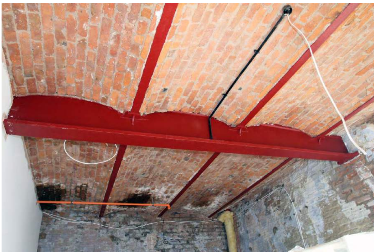
Plate 42. 'A' Mill, fourth floor, beam arrangement.
