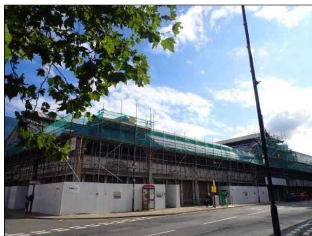
Photo 6: Lower Campfield, southern elevation, western end
