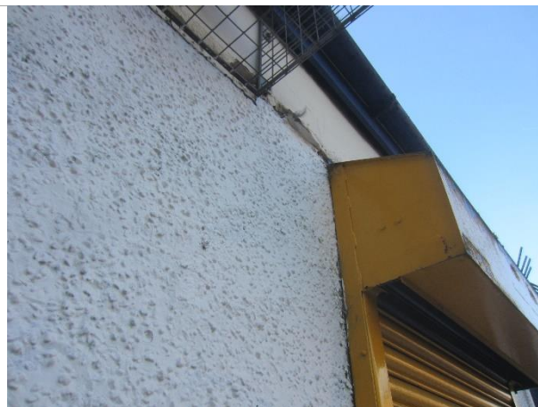
Photo 8: Sealed at fascia and doorways
