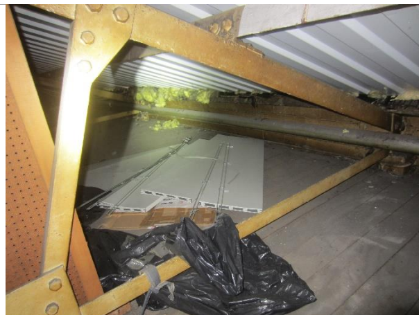
Photo 14: Under eaves storage areas – well-sealed
