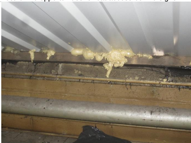
Photo 11: Expandable foam used to seal eaves
