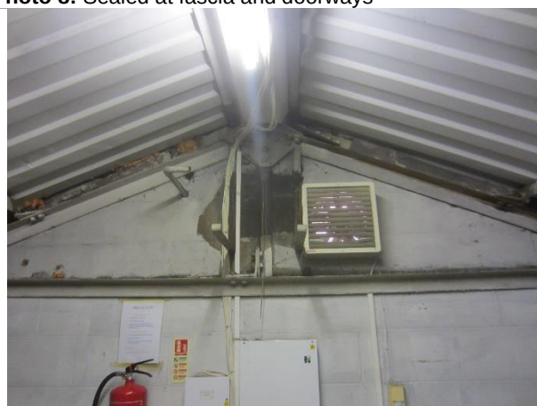
Photo 10: View of internal side of upper level
