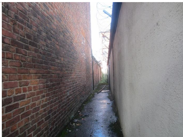
Photo 5: Southern elevation (right) and adjacent building (left)
