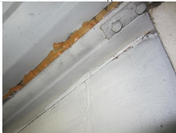
Photo 12: Expandable foam used to seal eaves
