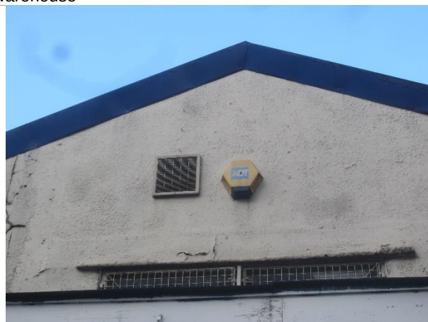
Photo 6: Sealed metal fascia at western elevation
