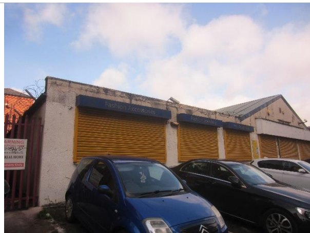
Photo 2: Eastern elevation of the warehouse taken from Cheetham Hill Road
