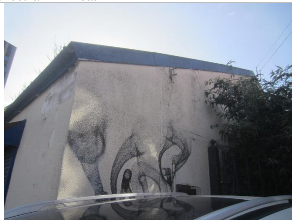
Photo 4: Western elevation of the pitched roof section of the warehouse
