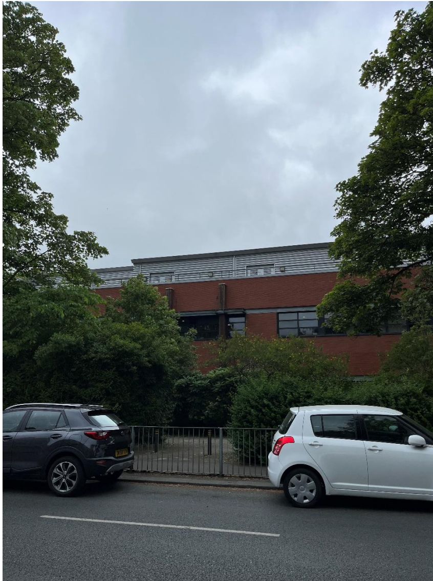
Figure 5.2: View of existing Withington Community Hospital from Burton Road
