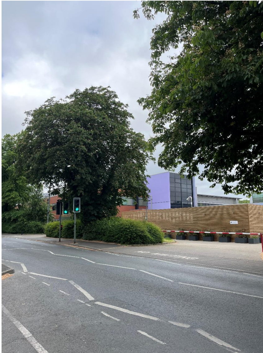
Figure 5.1: View of existing Withington Community Hospital from Burton Road
