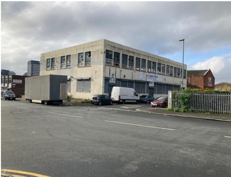
View from Redbank
