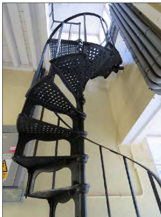
Figure 16: Painted steel spiral access stair to lift overrun tower and glazed access lobby.
