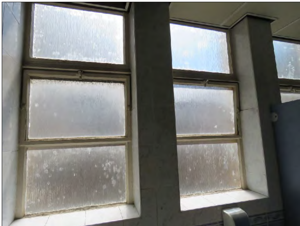
Figure 22: Typical original metal framed opening casement window to lavatories. (Considerable Significance)
