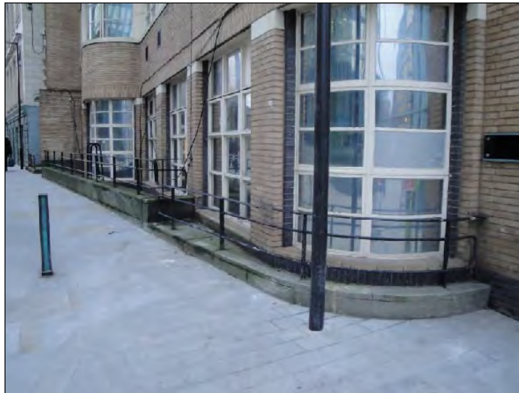
Figure 5: Retaining wall and railings to Dantzic street elevation, 27.11.2015. Below is a lightwell serving the basement areas. Recessed window reveals of buff blue engineering brick are also prominent here around the curved glass, a motif which appears throughout the building. (High Significance)
