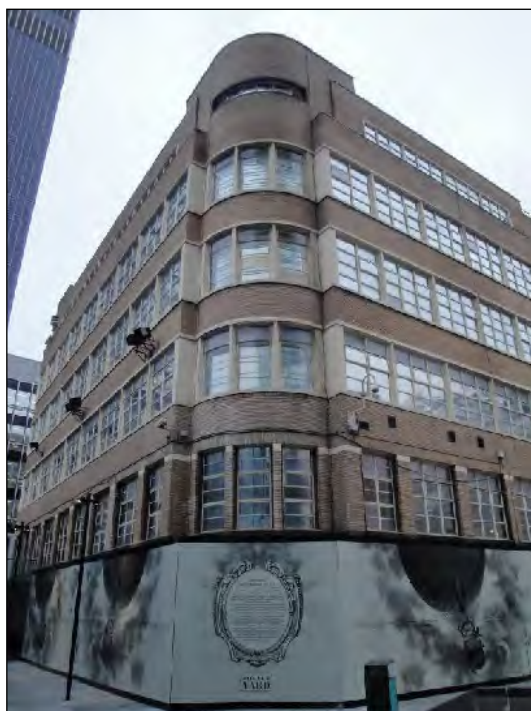
Figure 7: North and west elevations from Sadler's Yard, 27.11.2015. The two elevations are joined by an elegant section of original curved glazing terminated with brickwork and reconstituted Portland stone returns. (High Significance)
