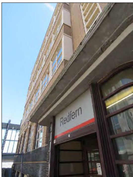
Figure 9: Main entrance doors with original timber and curved glazing screen, and concrete roof above. (High Significance) Recent signage can also be seen.
