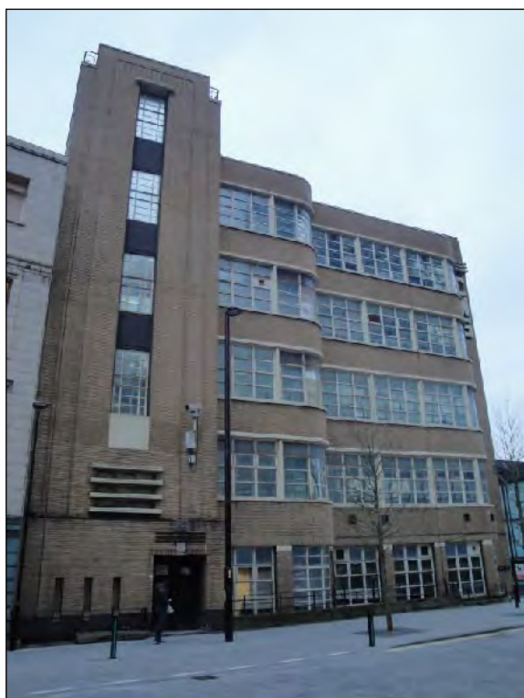
Figure 3: Principal east elevation facing Dantzic Street, 27.11.2015. The ancillary stair tower dominates the left (south) side of the composition, with recessed brickwork and large metal framed windows with side bars typical of the period. (High Significance)
