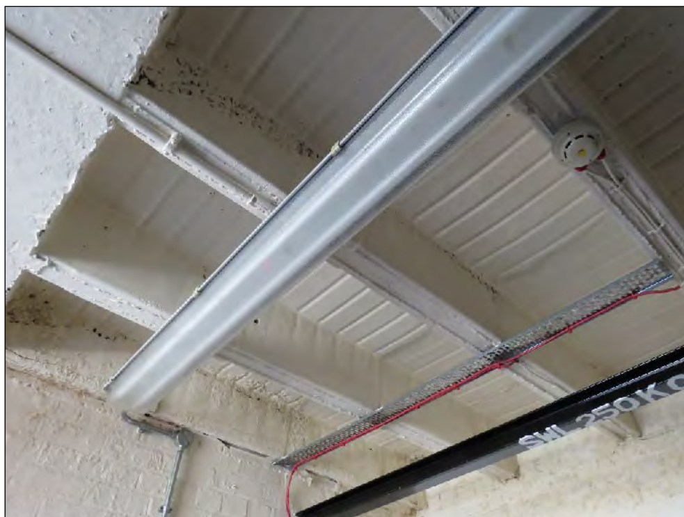
Figure 30: Concrete beam and block structure visible above passenger lift overrun to fifth floor, revealing structure of original build. (Considerable Significance)
