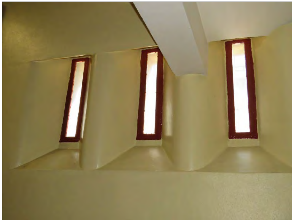
Figure 36: Secondary staircase (Core B) vertical slit windows deeply recessed into masonry wall thickness. (High Significance)
