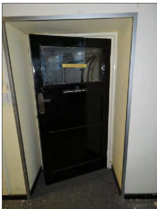
Figure 17: Original plant room door to basement, of typical 1930s form with three panels, the uppermost glazed. (Considerable Significance)
