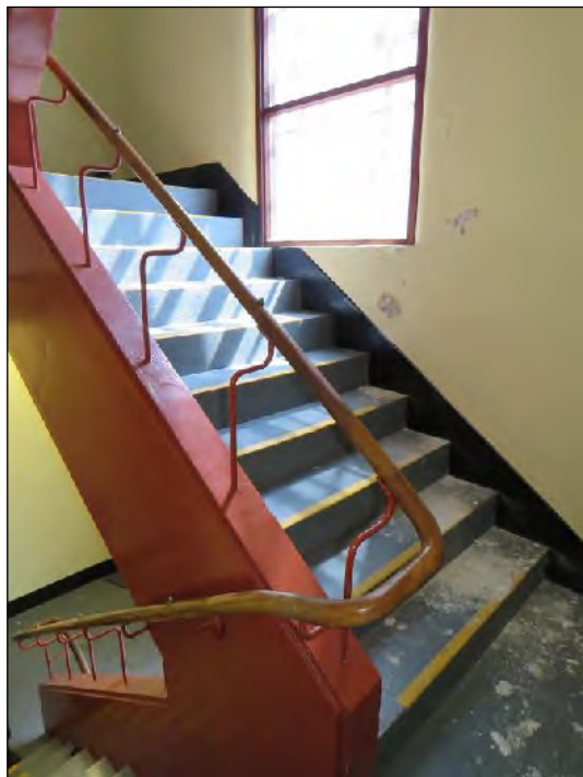
Figure 34: Secondary staircase (Core B) balustrade of timber with elegant steel fixings and brass caps on balustrade above. (High Significance)
