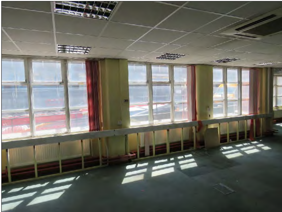
Figure 21: Typical view of ground floor interior. (Disposition of windows, columns and open plan space dating to original build and of Considerable Significance, but all partitions, fixtures and finishes of Low Significance)
