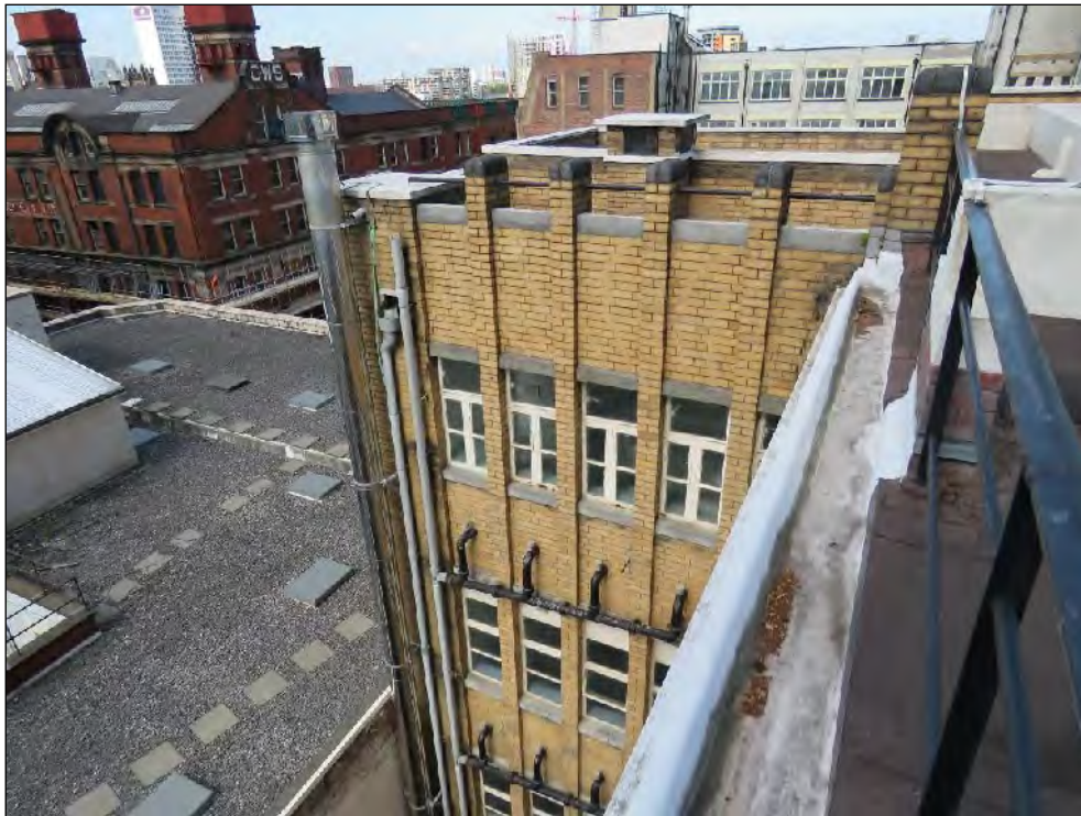
Figure 13: South elevation lightwell adjoining the Holyoake building. The CWS New Drapery Warehouse or E Block can be seen in the background, to the south-west of the site. The façade of the south elevation of the Redfern Building, although not designed to be seen, is marked by elegant recessed brickwork and original metal framed casement windows. (High Significance)
