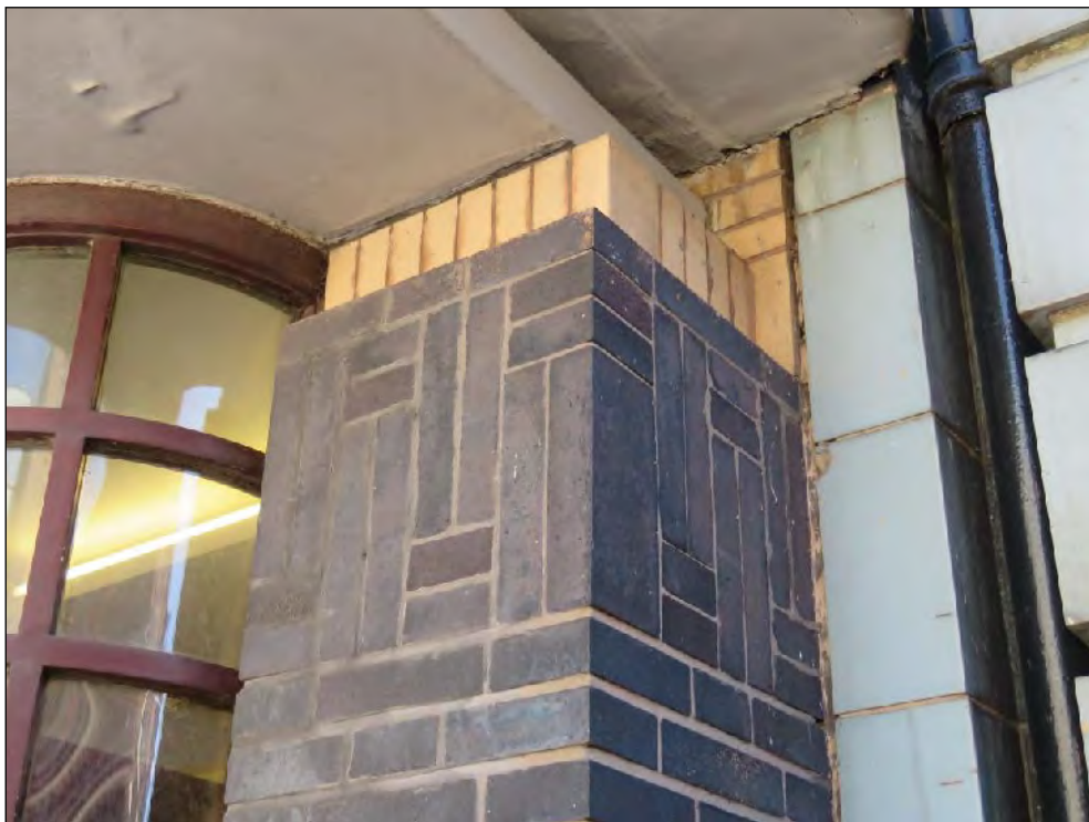
Figure 12: Capital of column adjacent to principal entrance formed of blue engineering brick with buff brick capping above.
