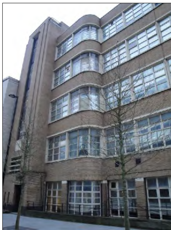
Figure 4: Principal east elevation facing Dantzic Street, 27.11.2015. This view shows the surviving original curved glazing and the more robust brick pilasters dividing the glazing sections at ground floor level, with reconstituted Portland stone pilasters. (High Significance) Later ventilation bricks can also be seen.
