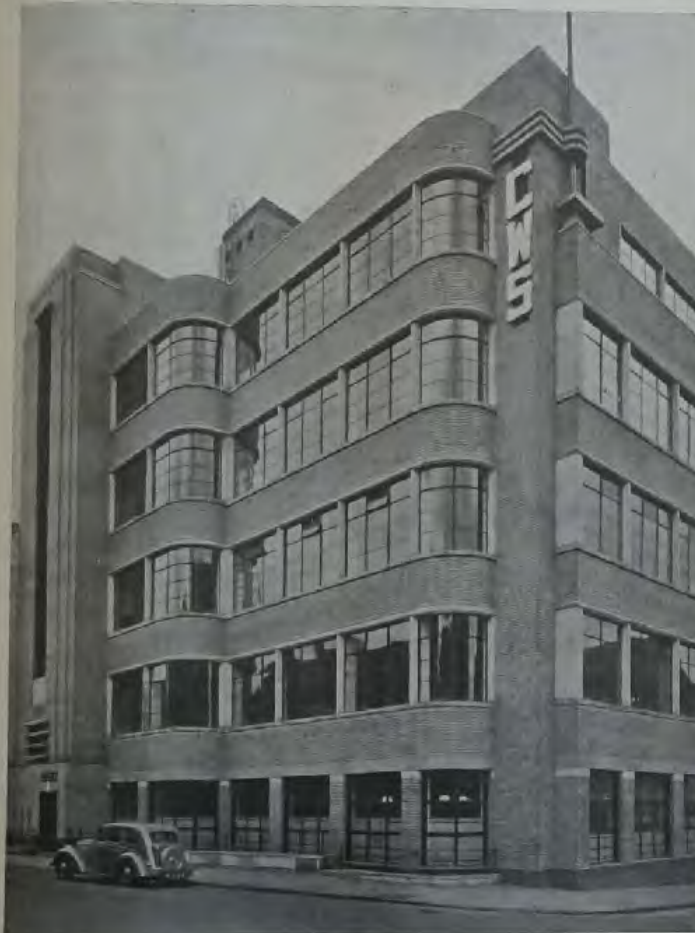
The exterior is finished in buff facing bricks, with 1/2-in. recessed joints.
