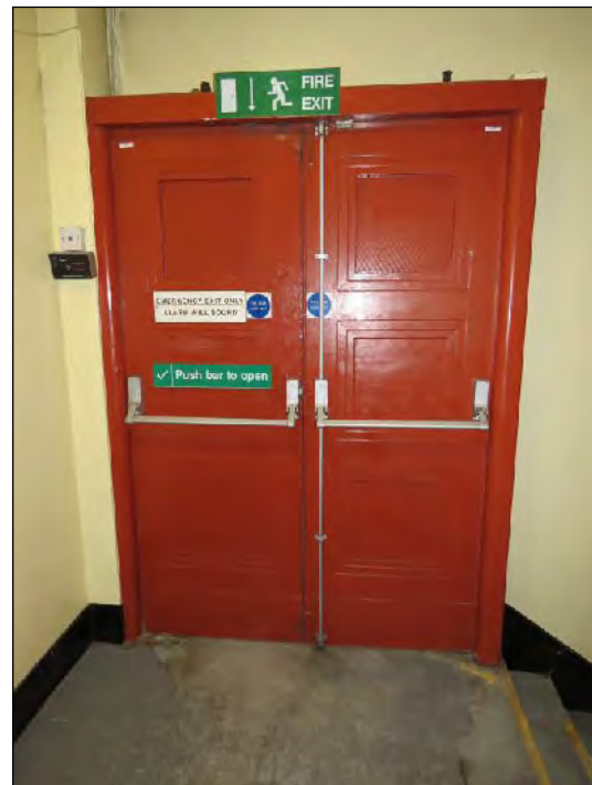
Figure 35: Secondary staircase (Core B) timber exit doors to Dantzic Street of typical 1930s form with recessed panels. (High Significance)
