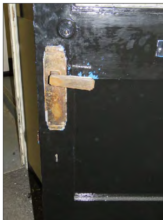
Figure 18: Plant room door with original brass door handle of typical 1930s form. (Considerable Significance)
