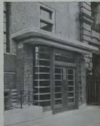
A detail of the main entrance, with blue brick piers.
