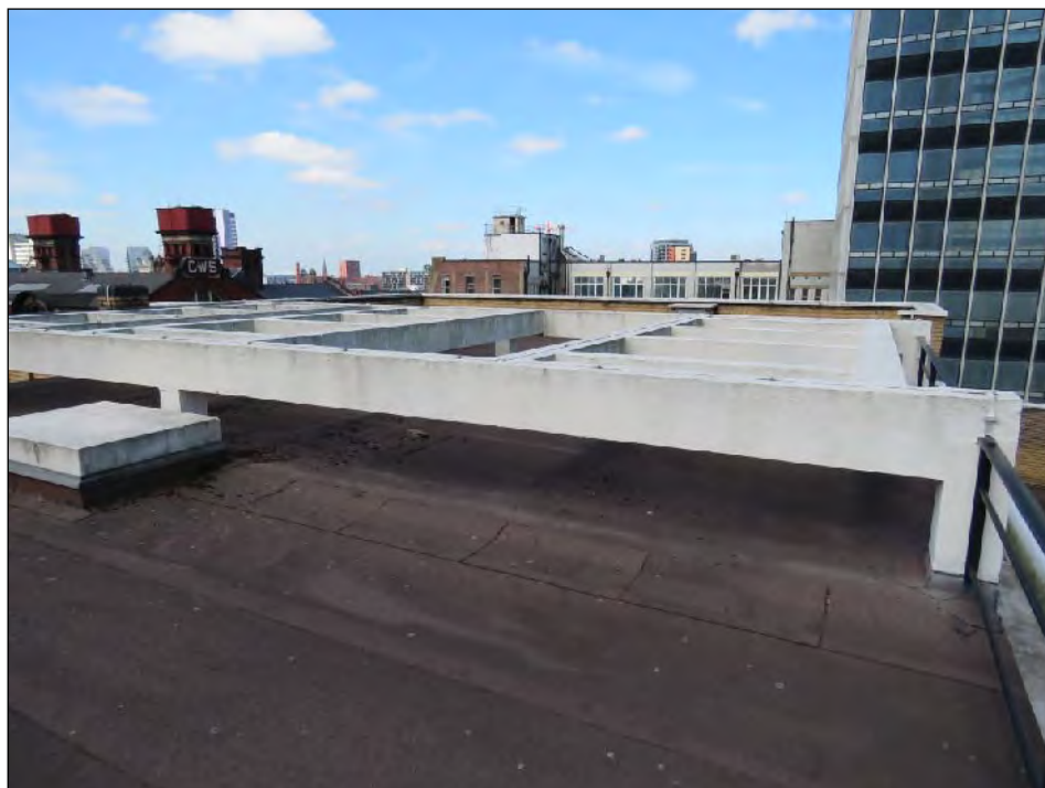
Figure 14: Fifth floor roof level with original brick parapets (High Significance) and later felt roof coverings and concrete web structure (Low Significance)
