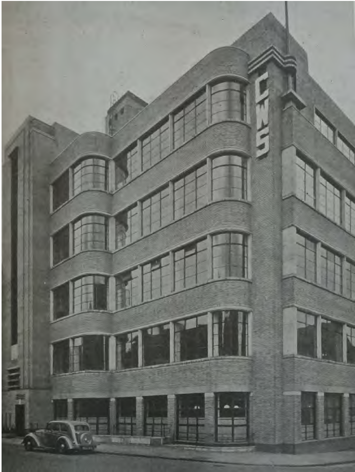
1937: The Redfern building, as completed, from Dantzic Street. The structure appears largely unchanged from its appearance in 2018, however the original windows with dark painted frames can be clearly seen. (The Architect and Building News).
