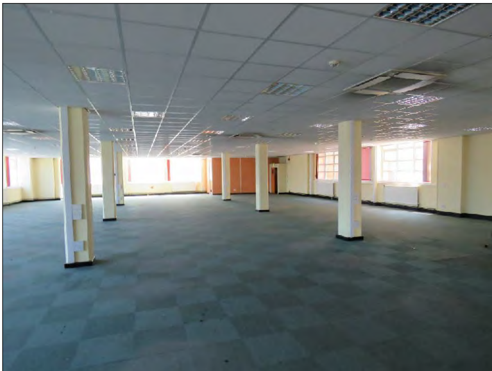
Figure 24: Typical view of second floor interior. (Disposition of windows, columns and open plan space dating to original build and of Considerable Significance, but all partitions, fixtures and finishes of Low Significance)
