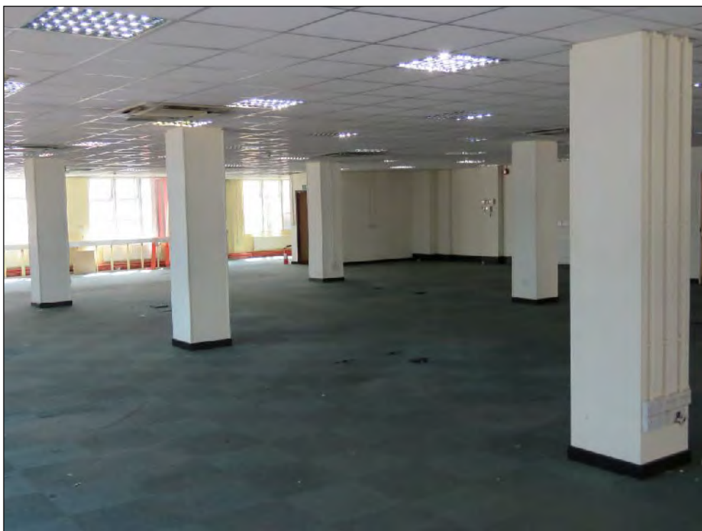
Figure 20: Typical view of ground floor interior (Disposition of windows, columns and open plan space dating to original build and of Considerable Significance, but all partitions, fixtures and finishes of Low Significance)
