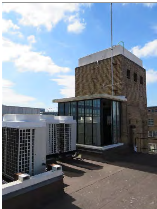
Figure 15: Brick lift overrun tower and glazed access lobby at roof level.
