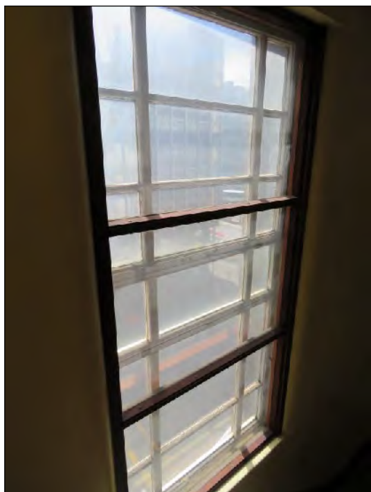
Figure 37: Secondary staircase (Core B) typical metal framed upper level window with side bars and later secondary glazing. (High Significance)
