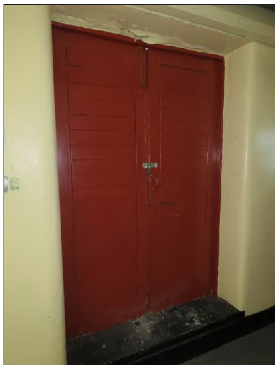
Figure 28: Timber double doors to fifth floor external roof area. (Considerable Significance)
