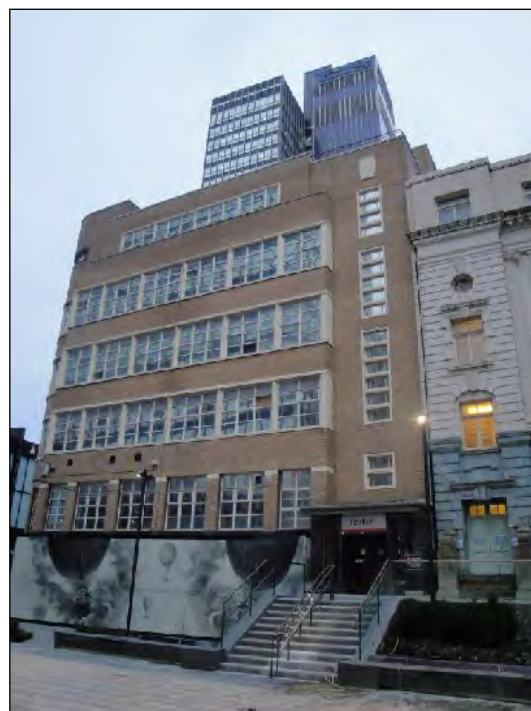
Figure 8: West elevation from Sadler's Yard, 27.11.2015. The CIS Tower may be seen in the background. The newly completed Sadler's Yard landscaping scheme has set the elevation considerably higher above ground level. (High Significance)
