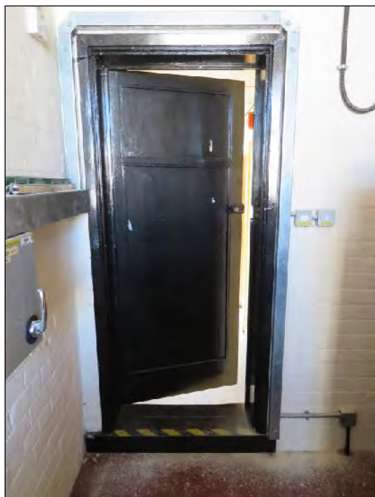
Figure 31: Timber door and frame to ancillary areas above passenger lift at fifth floor level. (Considerable Significance)
