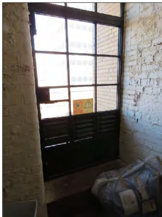
Figure 32: Partially glazed timber door at fifth floor level giving access to roof terrace areas. (High Significance)
