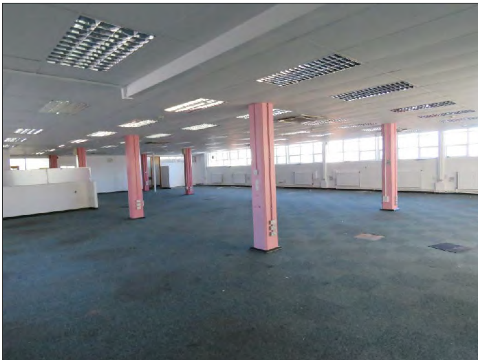
Figure 26: Typical view of fourth floor interior. (Disposition of windows, columns and open plan space dating to original build and of Considerable Significance, but all partitions, fixtures and finishes of Low Significance)
