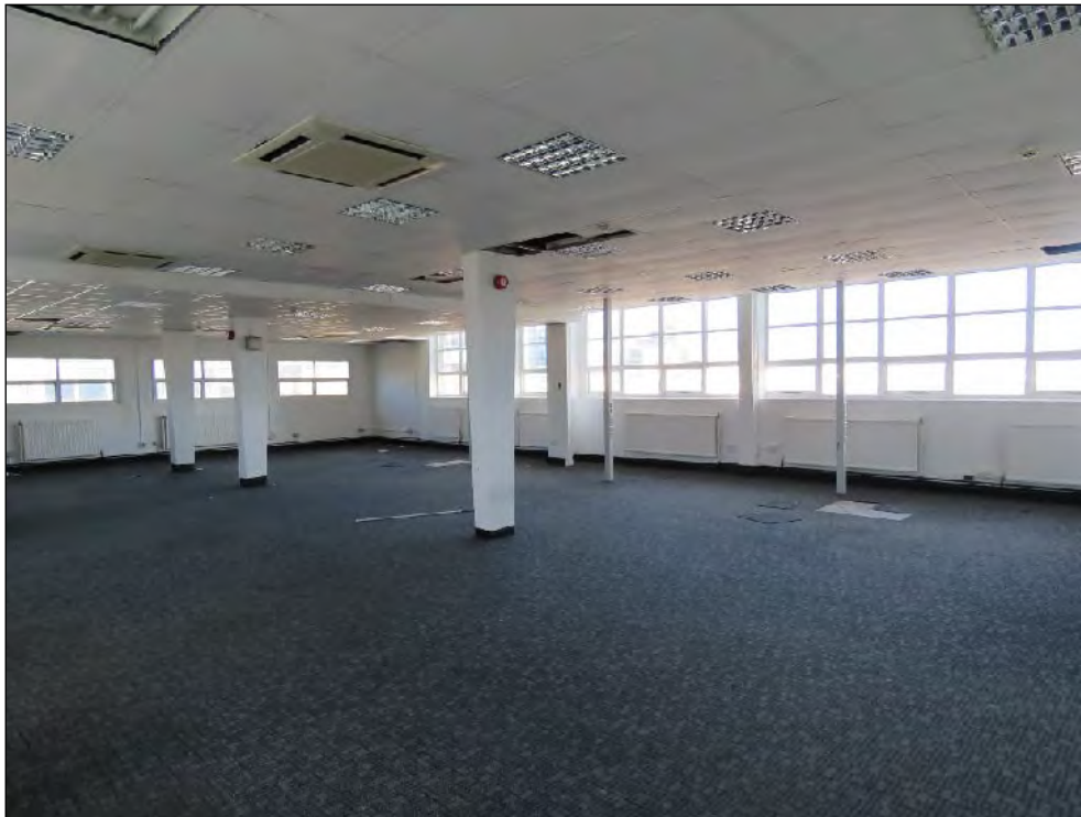
Figure 33: Typical view of fifth floor interior, note the widened columns. (Disposition of windows, columns and open plan space dating to original build and of Considerable Significance, but all partitions, fixtures and finishes of Low Significance)
