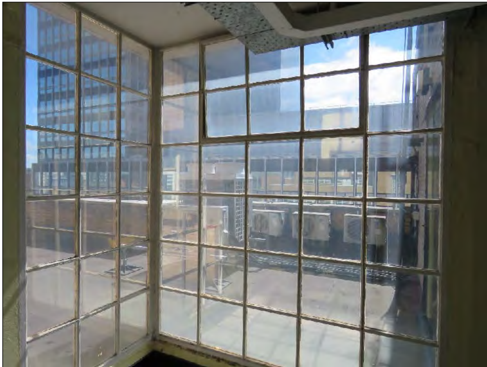
Figure 27: Steel framed glazing sections to fifth floor beneath lift overrun tower. (High Significance)
