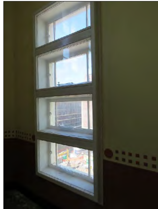
Figure 40: Principal staircase (Core A) side opening metal framed casement windows and later secondary glazing. (High Significance).
