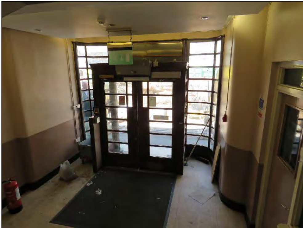
Figure 19: Ground floor entrance lobby with curved wall sections matching curved external glazed joinery screen.
