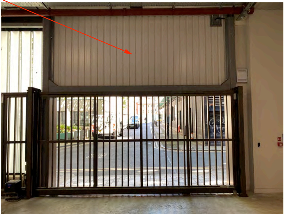
Rear view of Car Park entrance externally and internally
