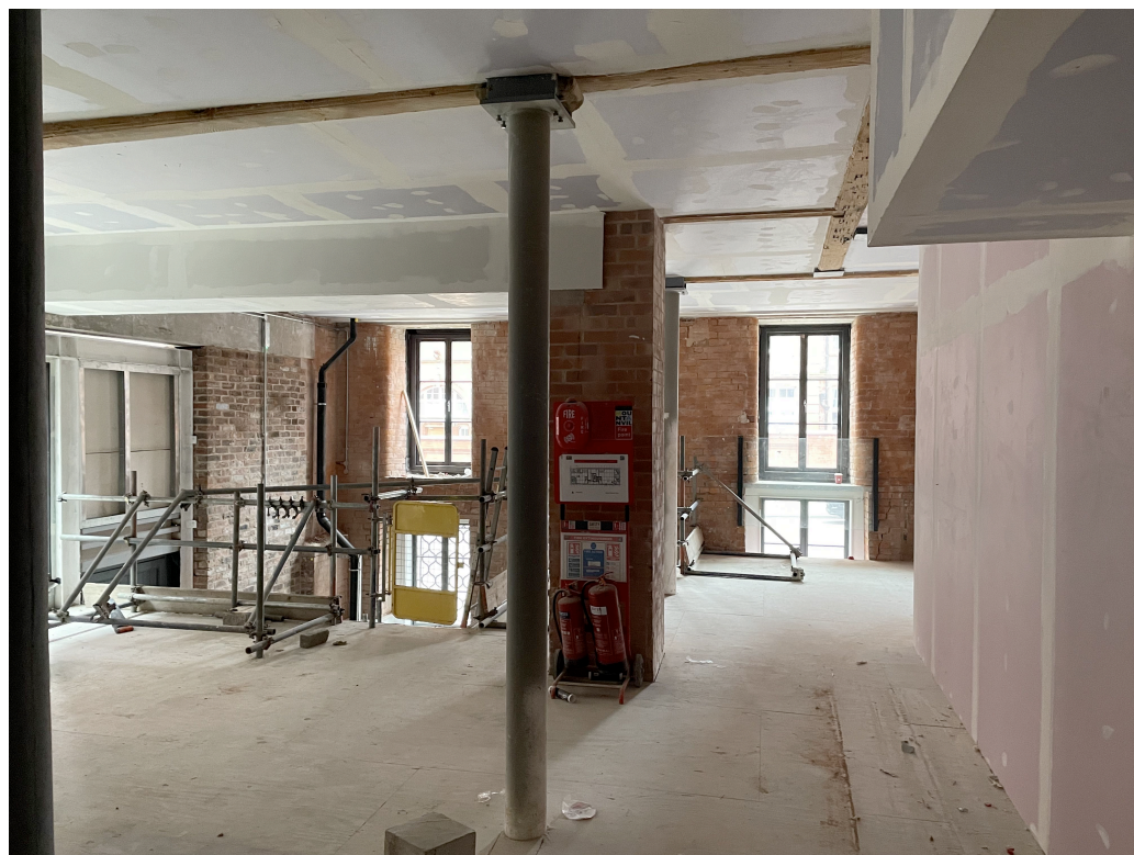
02 view of unit existing interior
