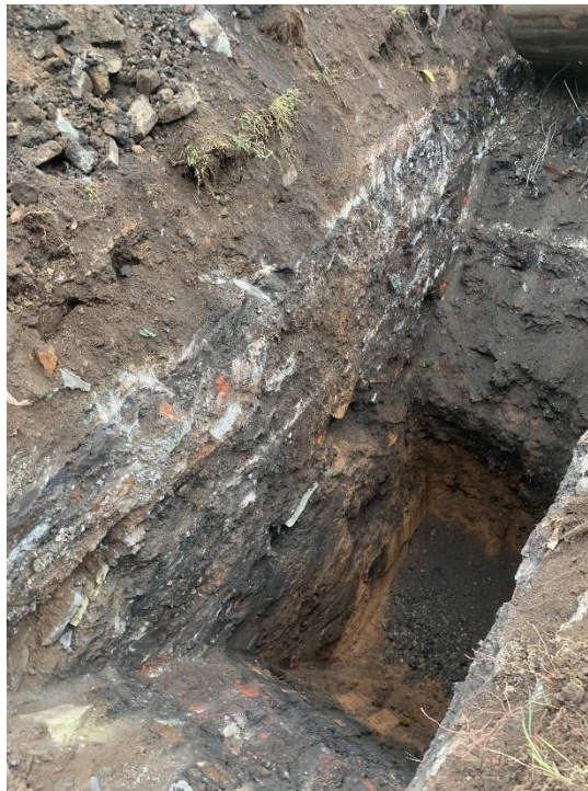
EXCAVATION FOR CULVERT TRENCH (EASTERN SECTOR)
