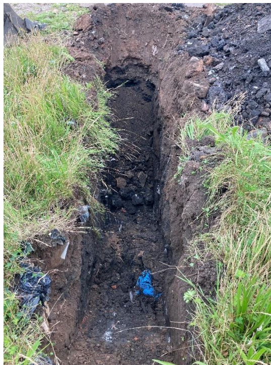
EXAMPLE OF SHALLOW GRANULAR MADE GROUND (TP106)
