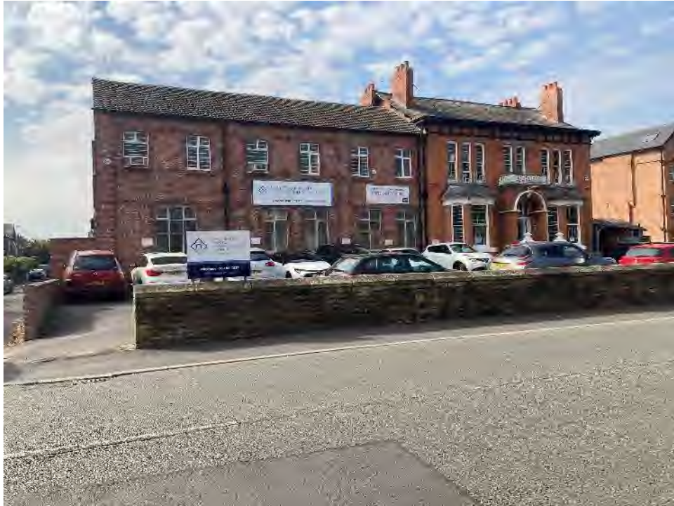
Plate 1: View south towards the northern façade of the school
