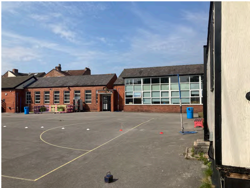
Plate 4: View west towards buildings along the western boundary of the study site
