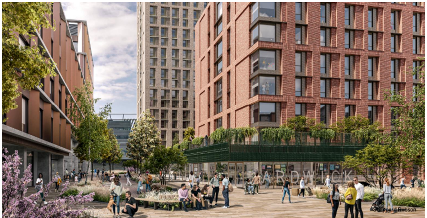
Figure 1-2: Site View- Upper Brook Street
