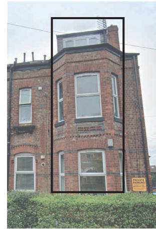
Existing semi's on Stockton Road
