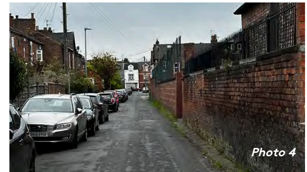
Existing wall fronting Acres Road.
