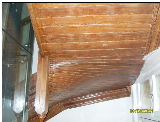
Underside of timber staircase
