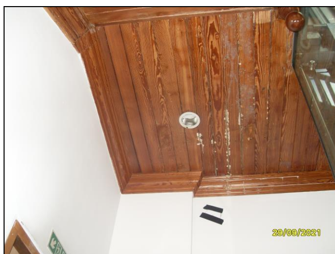
Underside of timber staircase
