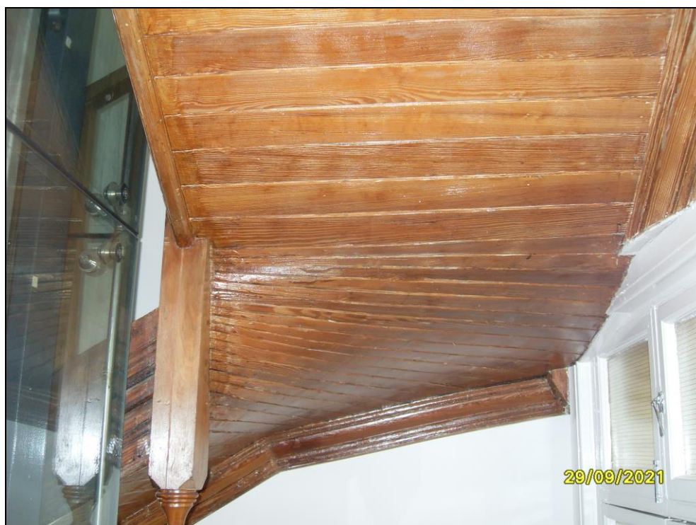
Underside of timber staircase
