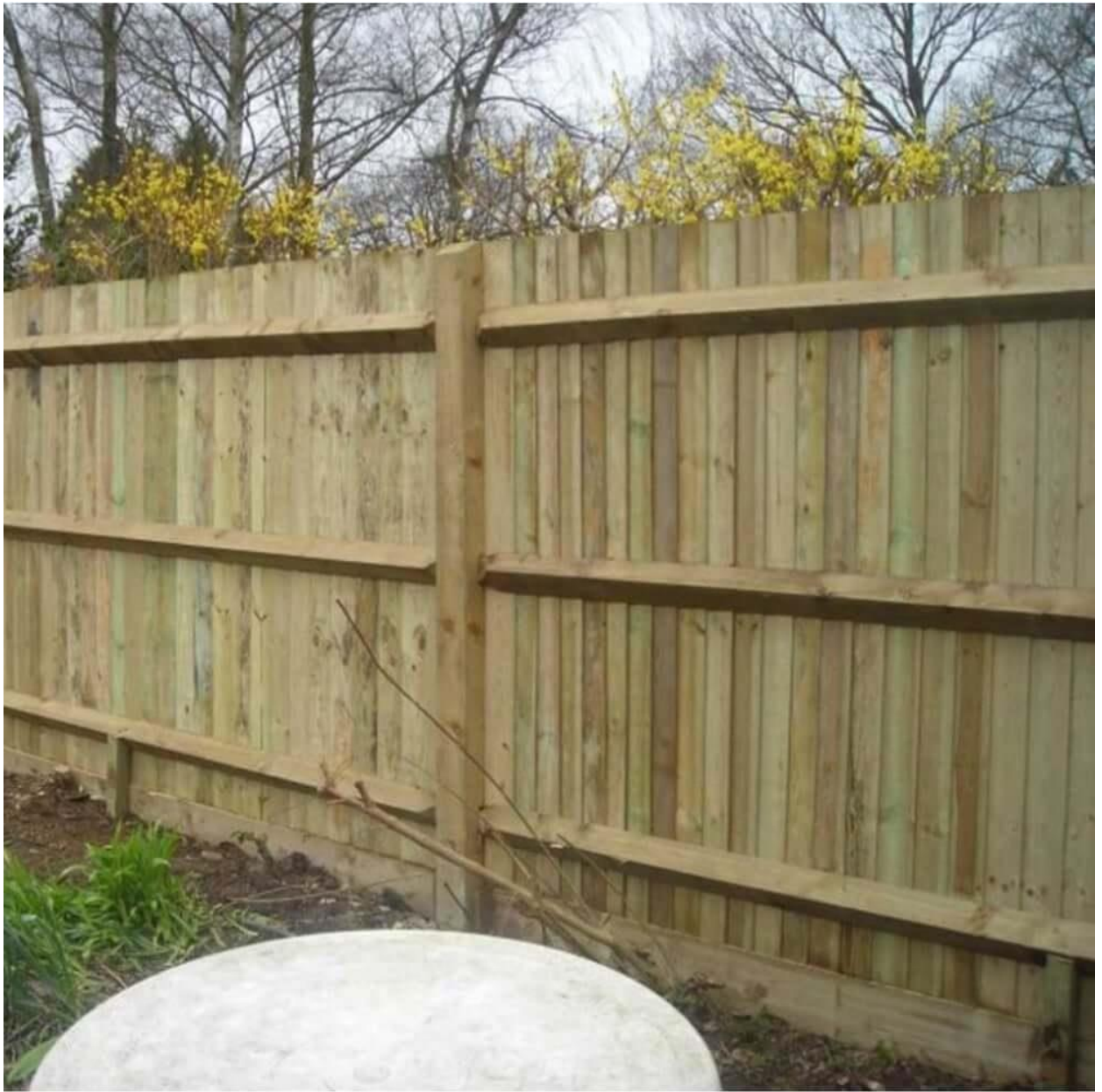
Figure 6, Similar fencing used
