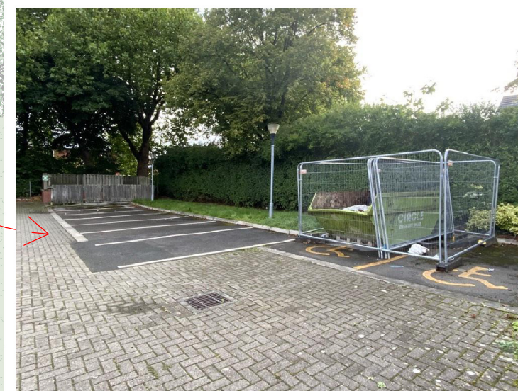
Existing disabled parking
