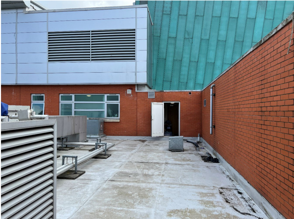
Photograph 2: The main plantroom is located within the main building next to the Air Handling Units, as noted by the white door.
