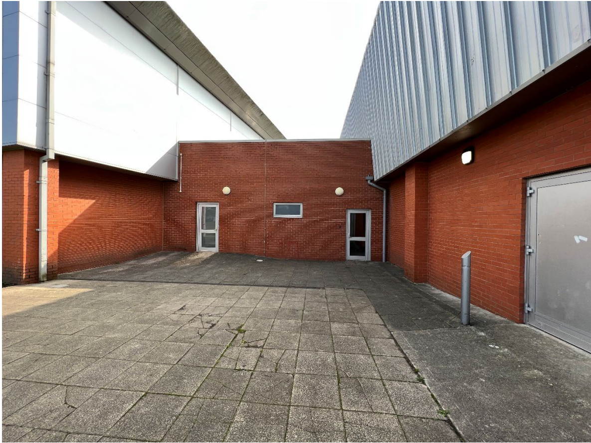
Photograph 3: Fire exits to be maintained during and after works completed
