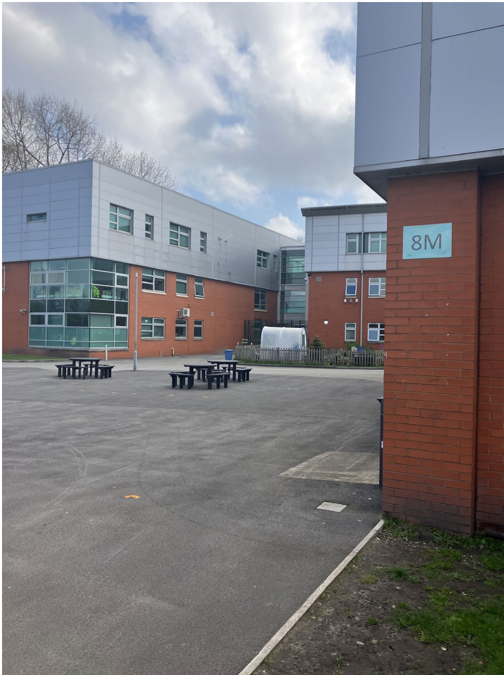
Photograph 4: The macadam area that will be trenched for pipework to the sixth form block on the west. The pipework to the main building will be above ground.
