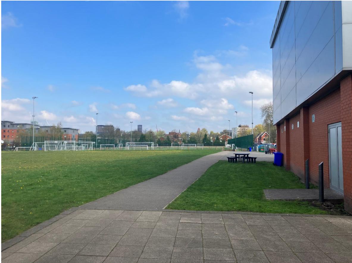
Photograph 1: Proposed area for new Air Source Heat Pump compound on green space where existing path is located.
