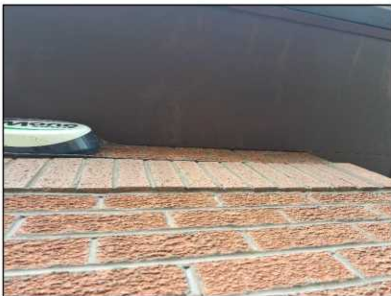
Figure 4 showing the wooden soffit
