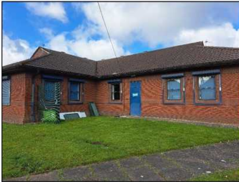
Figure 5 showing the ridge vents
