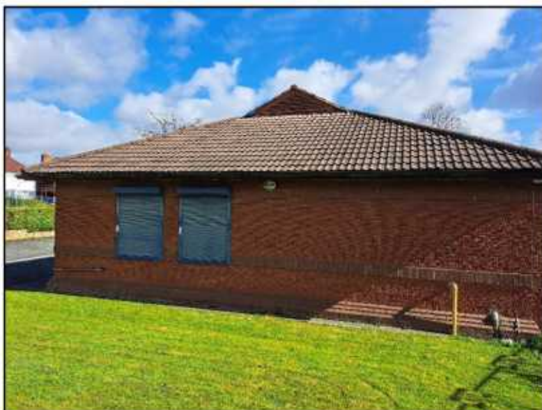
Figure 3 showing the rear of the site
