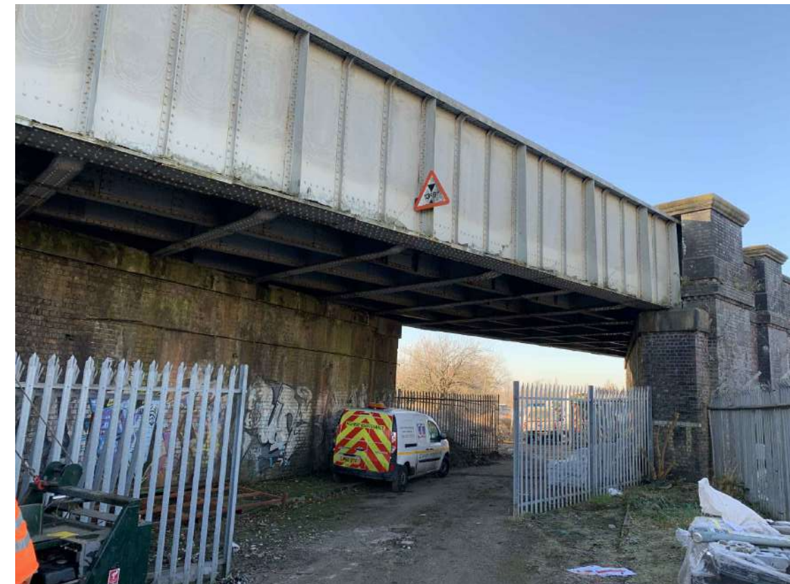
NORTH ELEVATION (PHOTO AS TAKEN IN 2022)
