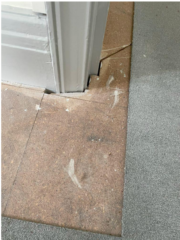
Raised access floor detail
