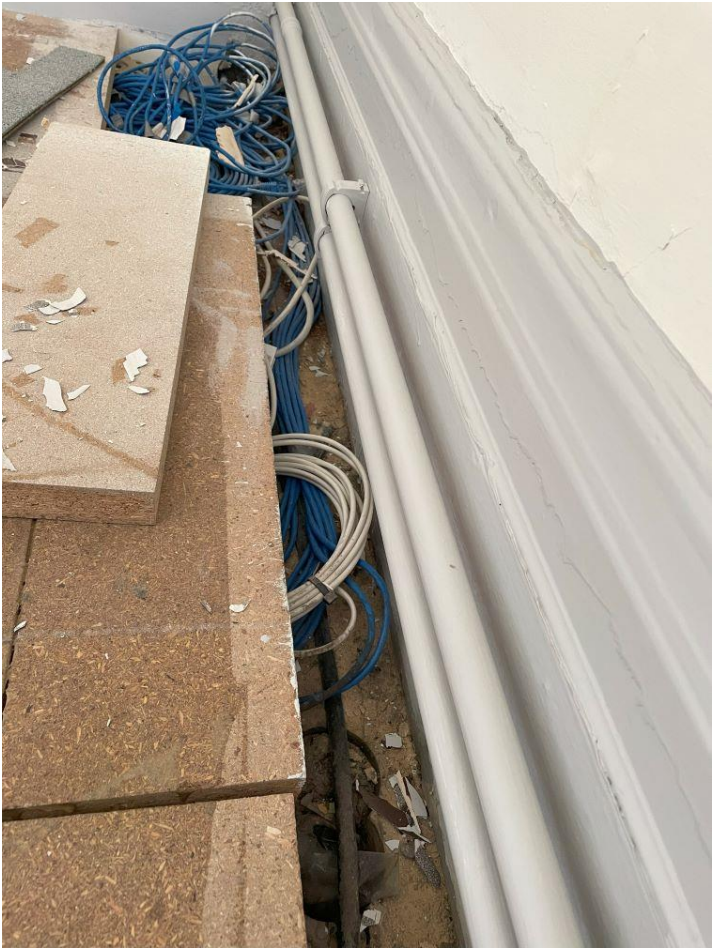
Raised access floor above base of skirting
