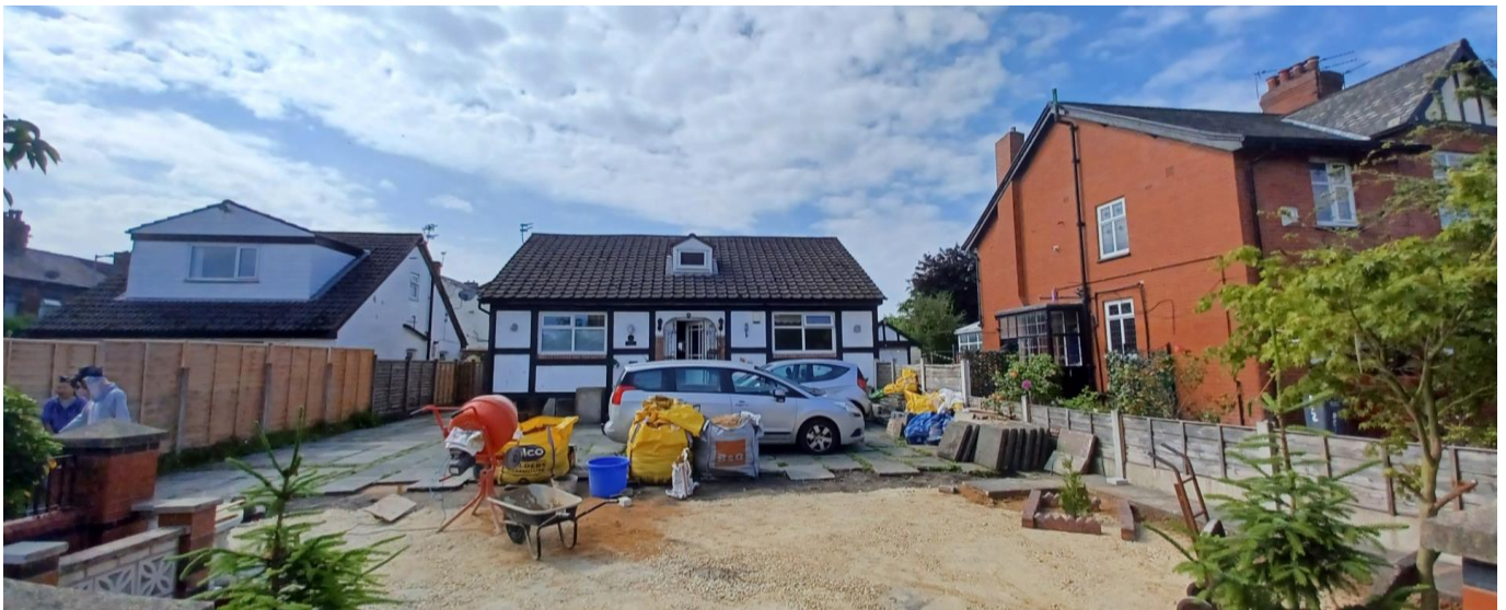
Figure 1. Principal elevation of property.
