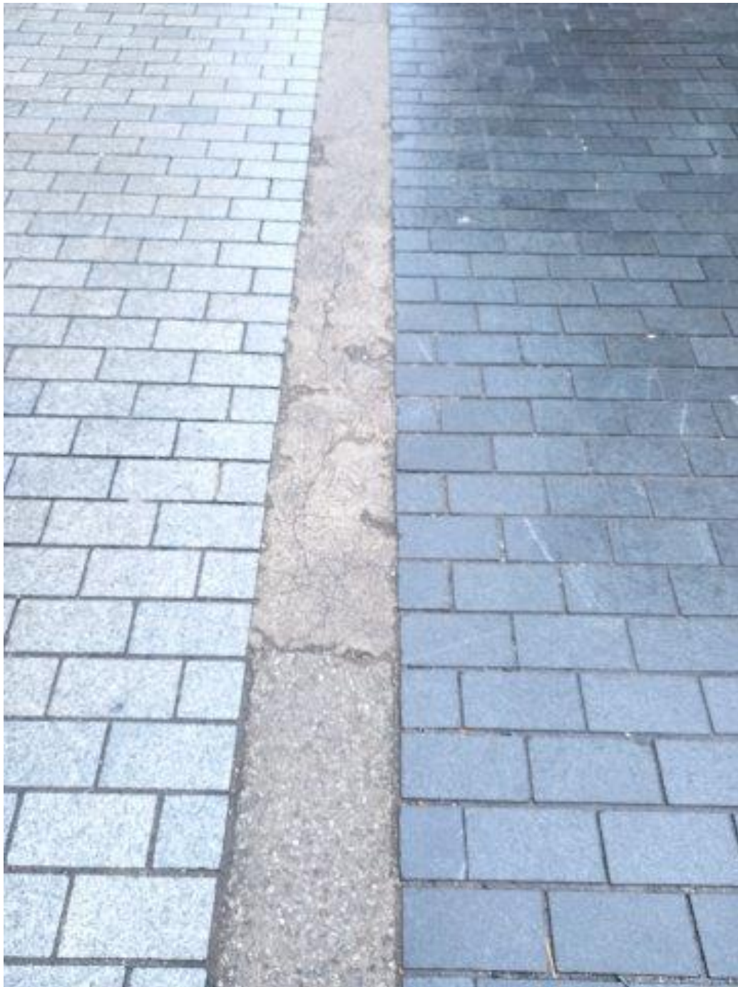
Junction of Bridgeford St and Higher Chatham Street
