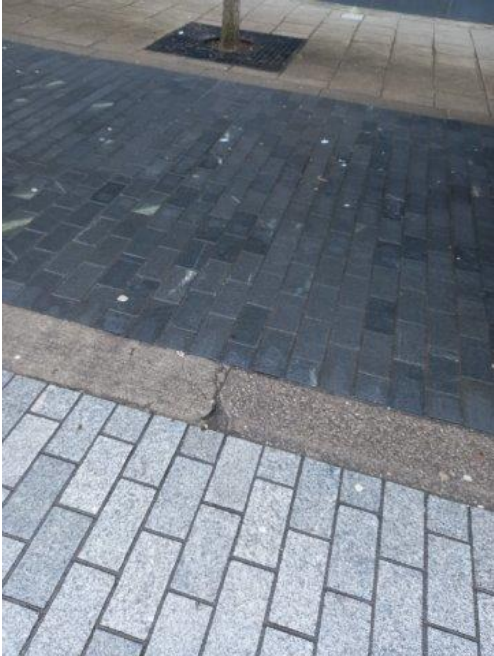
Between the dental hospital and third mesh panel to the high rise car park (left of car park entrance)
