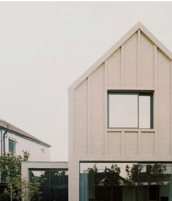
Projecting vertical header course To gables and ground floor
