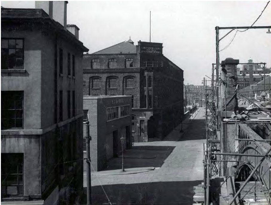
E - 1952 - View along Altrincham St
