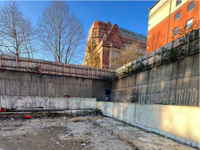
View 1: View of the retaining wall
