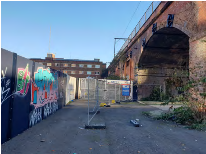
View 2: View of the Viaduct Arch access
