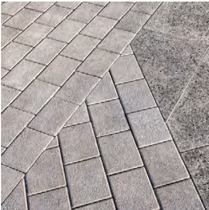
Concrete block paving
