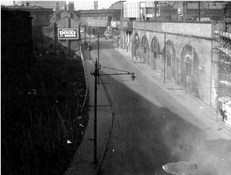
C - 1959 - View along Altrincham St
