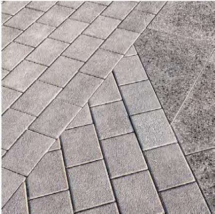
Concrete Block Paving
