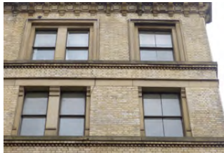
Conservation Area Brick
