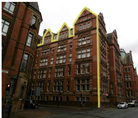
Distinctive roof-line separates bays
