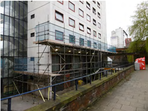
The west facade of Chandos Hall faced Vimto Park, and whilst it was connected in one location through the link bridge, the isolation of the block was a missed opportunity.
