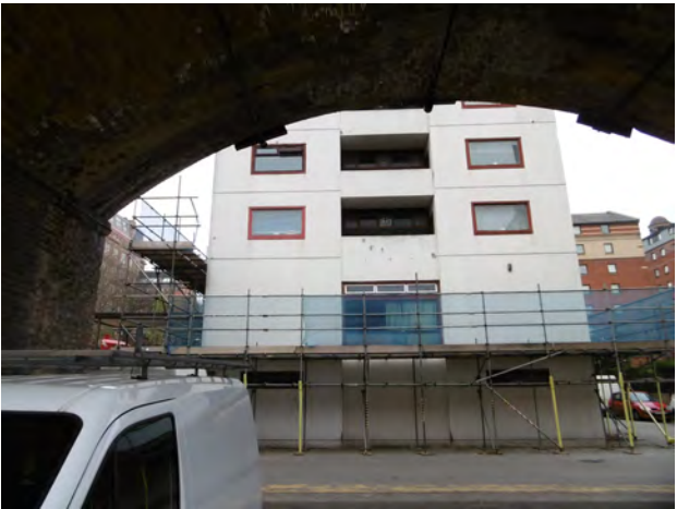
Service access to the building was provided through the light-well, allowed by the difference in level between Granby Row and Altrincham Street.
