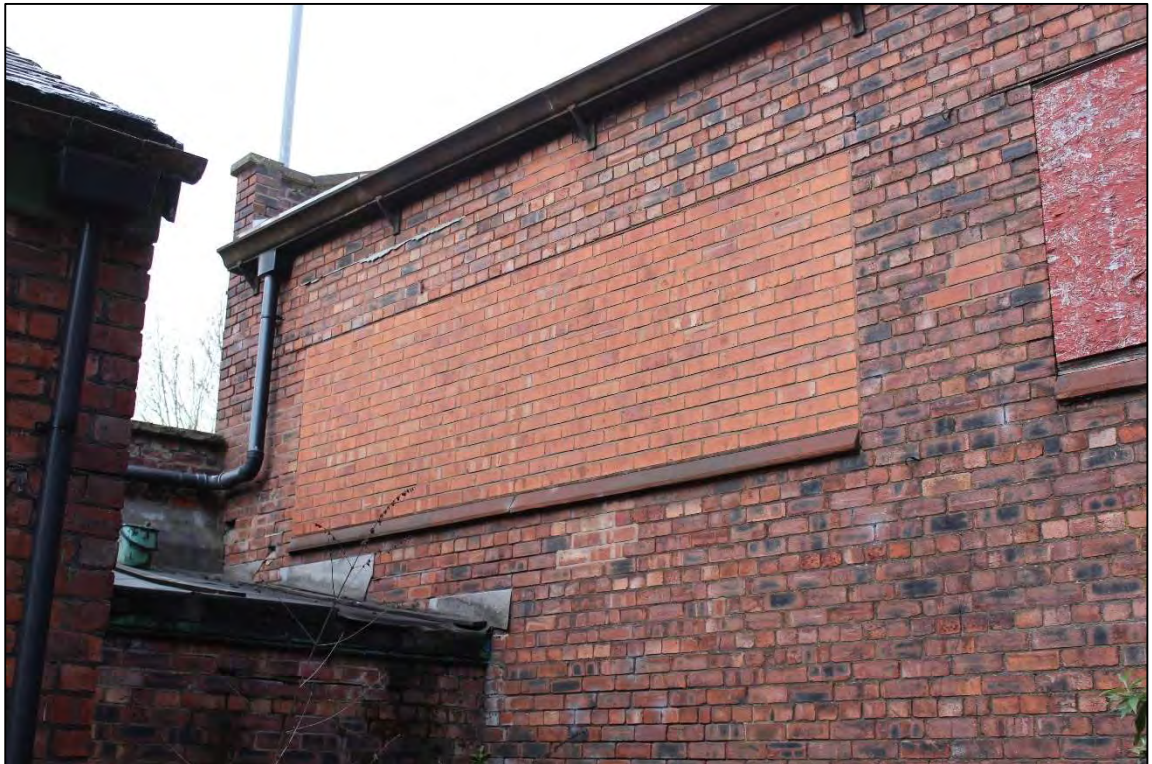
Plate 21: The infilled window to the southern end of the eastern elevation
