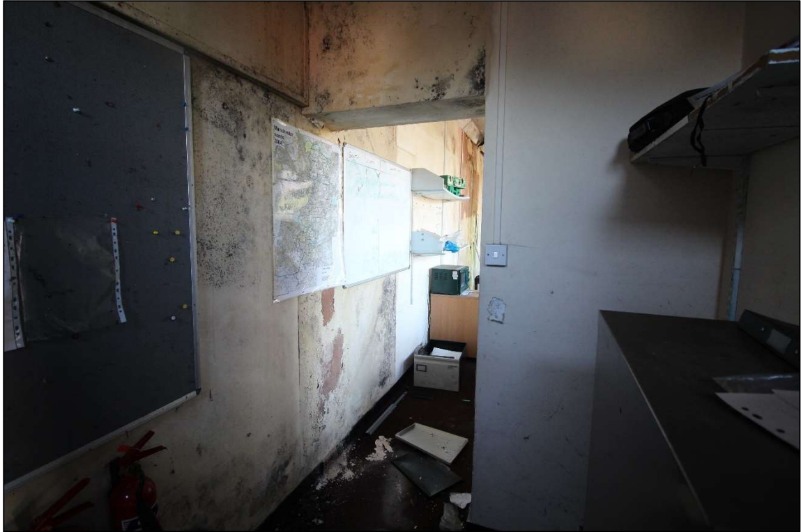
Plate 44: General view of Room 2 of the office block, facing south-east
