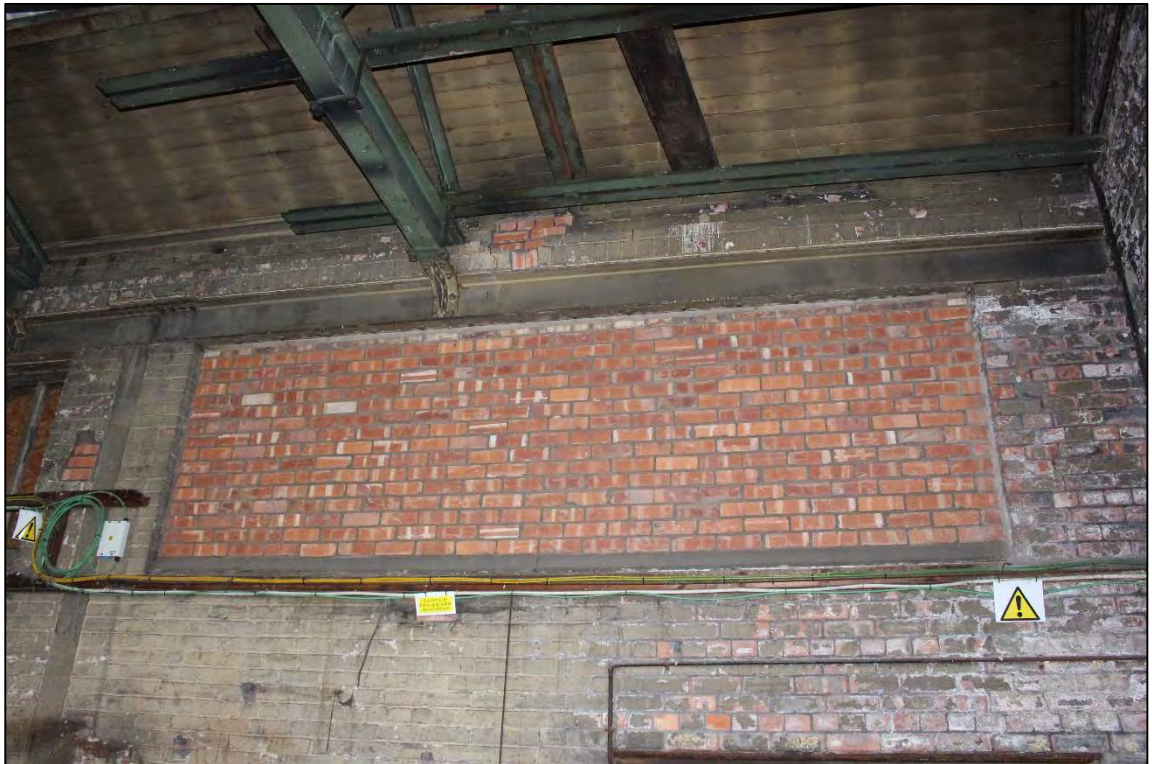
Plate 29: The infilled window to the southern end of the eastern wall of Room 1
