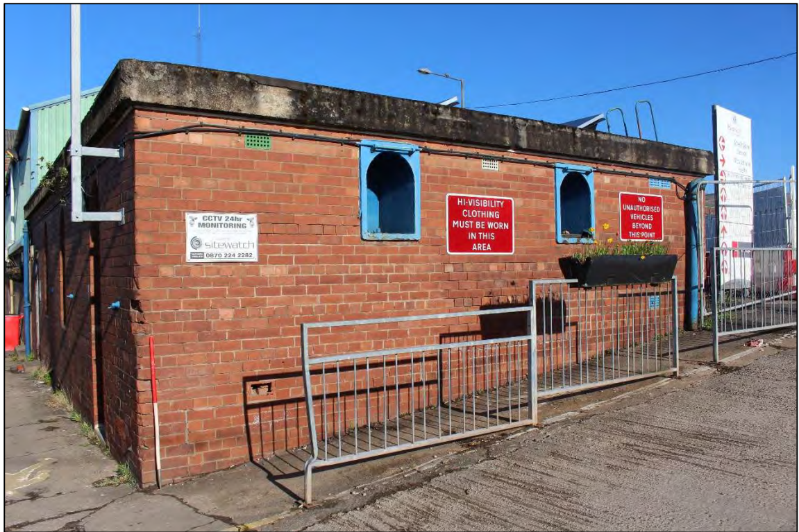
Plate 50: General view of the eastern elevation, looking north-west
