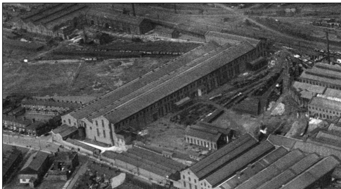
Plate 9: Aerial view of the new boiler shop taken in 1927
