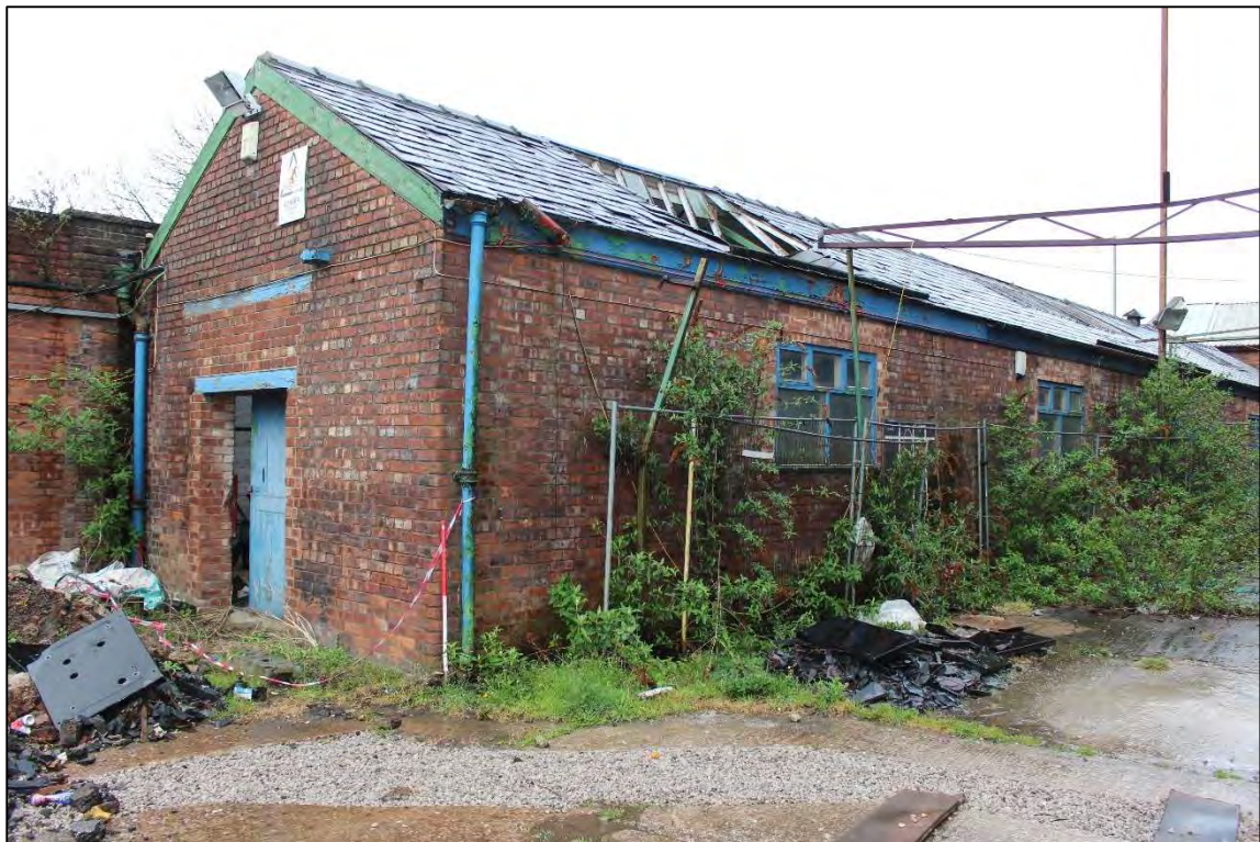
Plate 11: General view Shed 1 looking south-west
