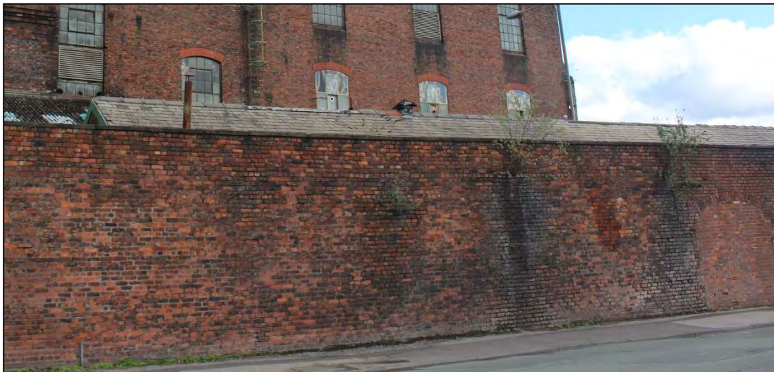
Plate 15: General view of the southern elevation Shed 1
