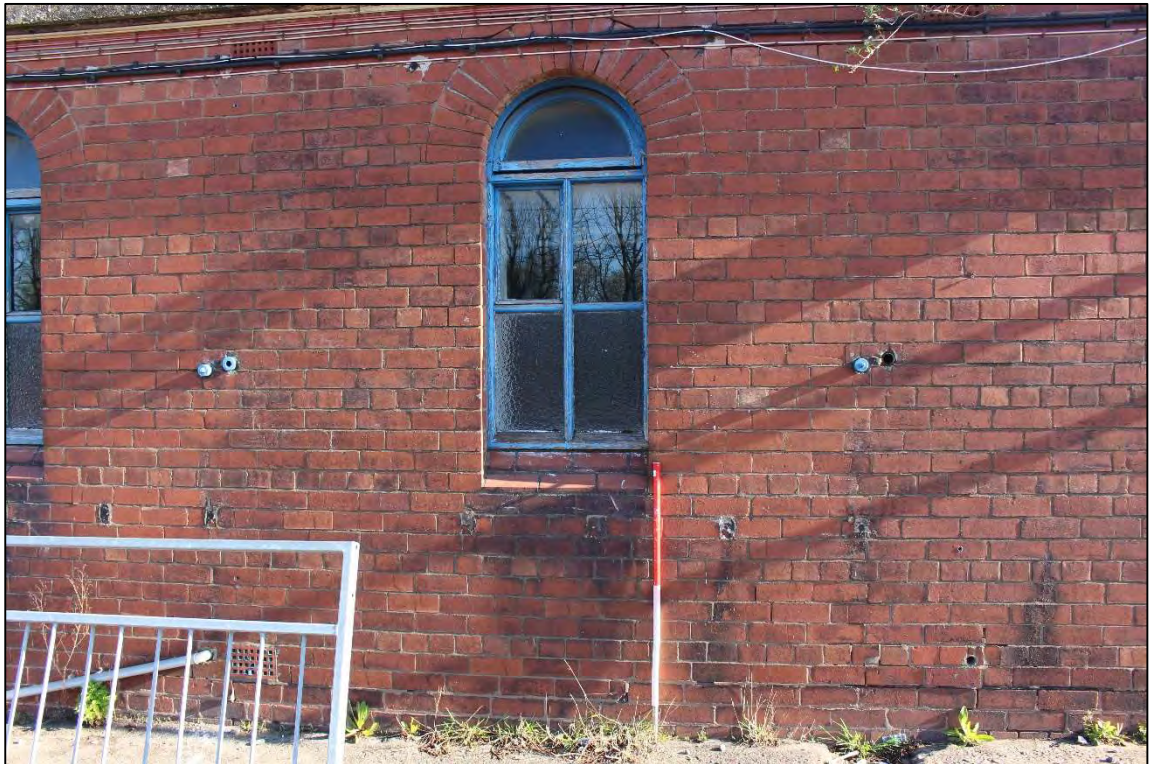
Plate 47: Detail of the central windows within the southern elevation, looking north
