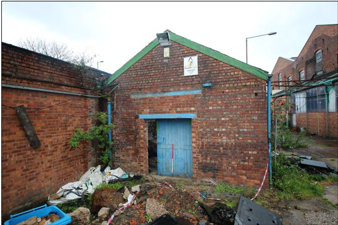
Plate 12: General view of the eastern elevation Shed 1
