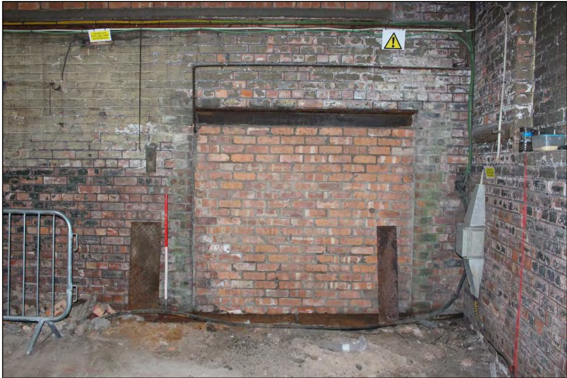
Plate 30: The blocked doorway within the eastern wall of Room 1
