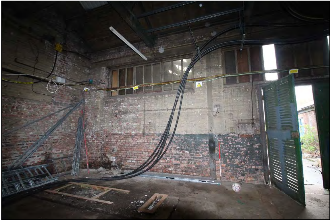
Plate 28: The window aperture to the northern end of the eastern wall of Room 1
