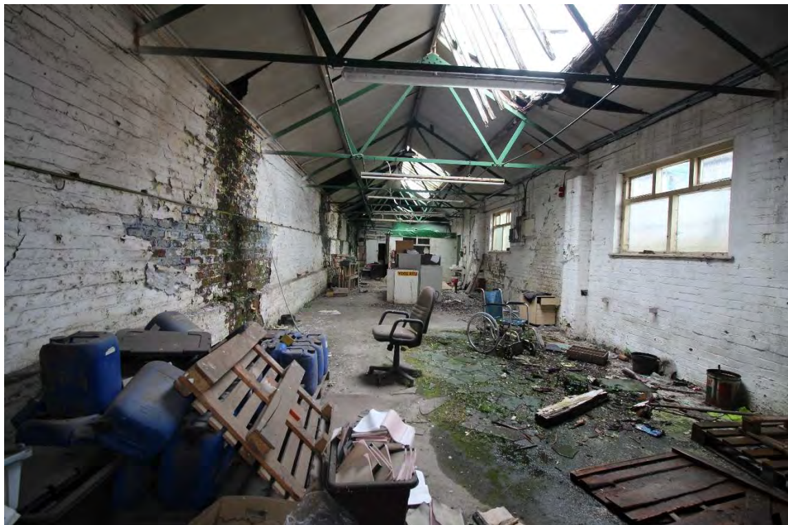
Plate 18: General internal view of Shed 1, looking west
