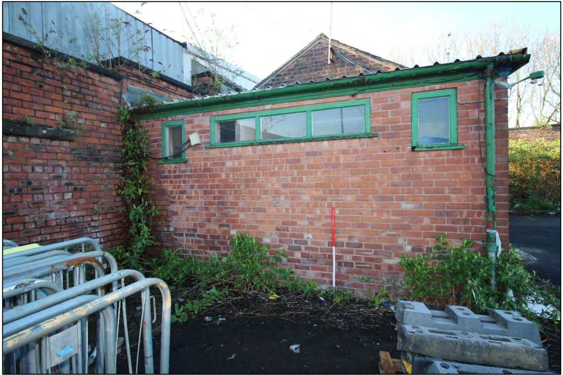
Plate 41: General view of the northern elevation of the office block
