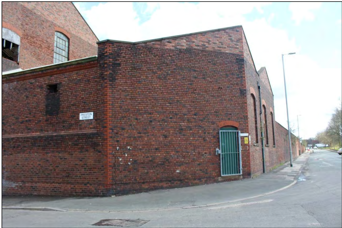
Plate 23: General view of the south-western elevation Shed 2
