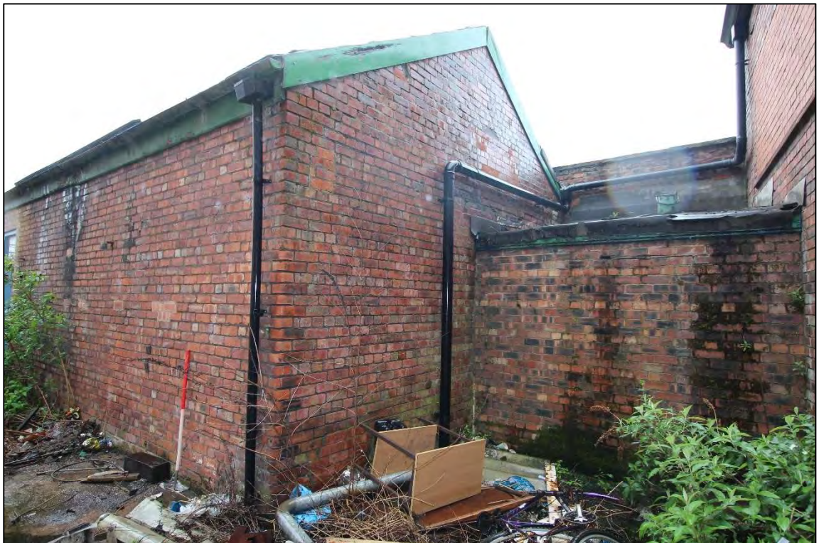
Plate 17: General view of the western elevation Shed 1
