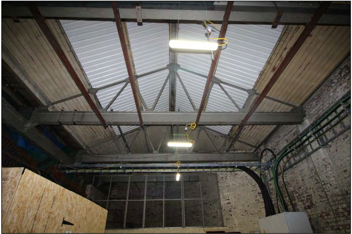
Plate 35: Detail of the fink trusses in Room 3
