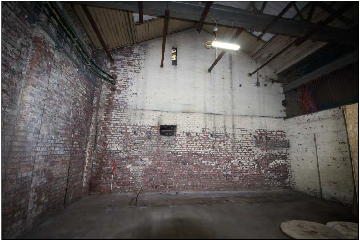
Plate 36: The northern wall of Room 3 with an exposed wall box to the left of the photograph
