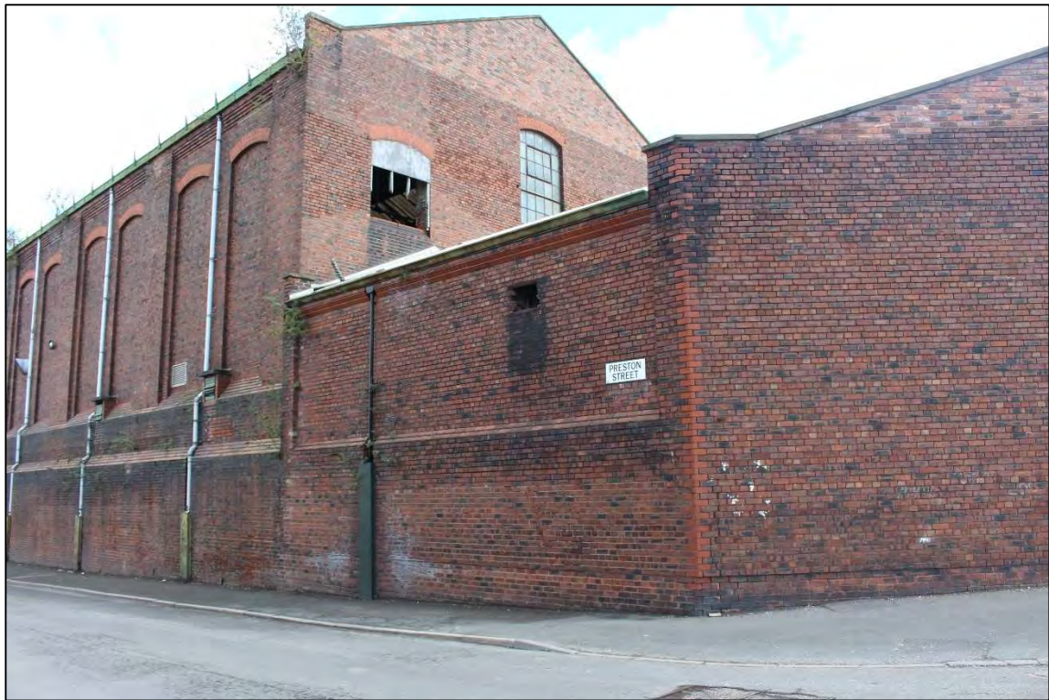
Plate 24: General view of the western elevation Shed 2
