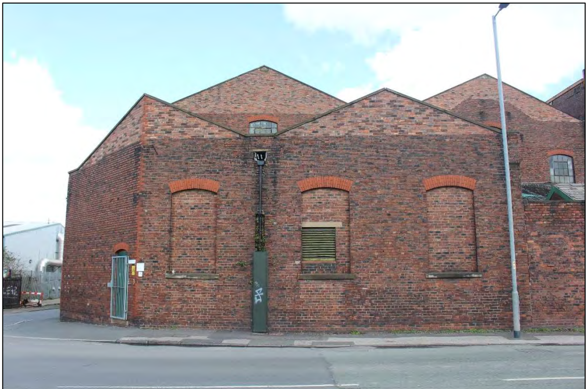
Plate 22: General view of the southern elevation Shed 2
