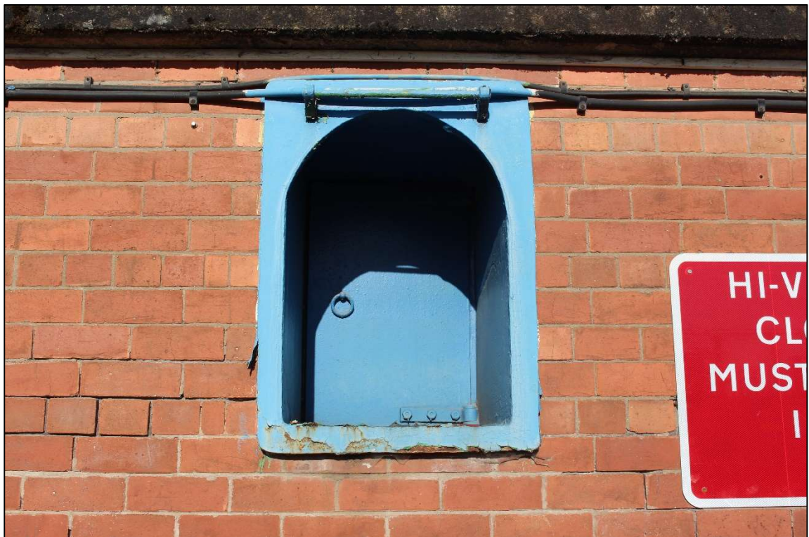
Plate 51: Detail of the cast-iron surround window to the eastern elevation, looking west
