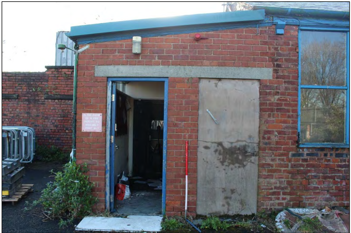
Plate 40: The two doorways within the western elevation of the lean-to
