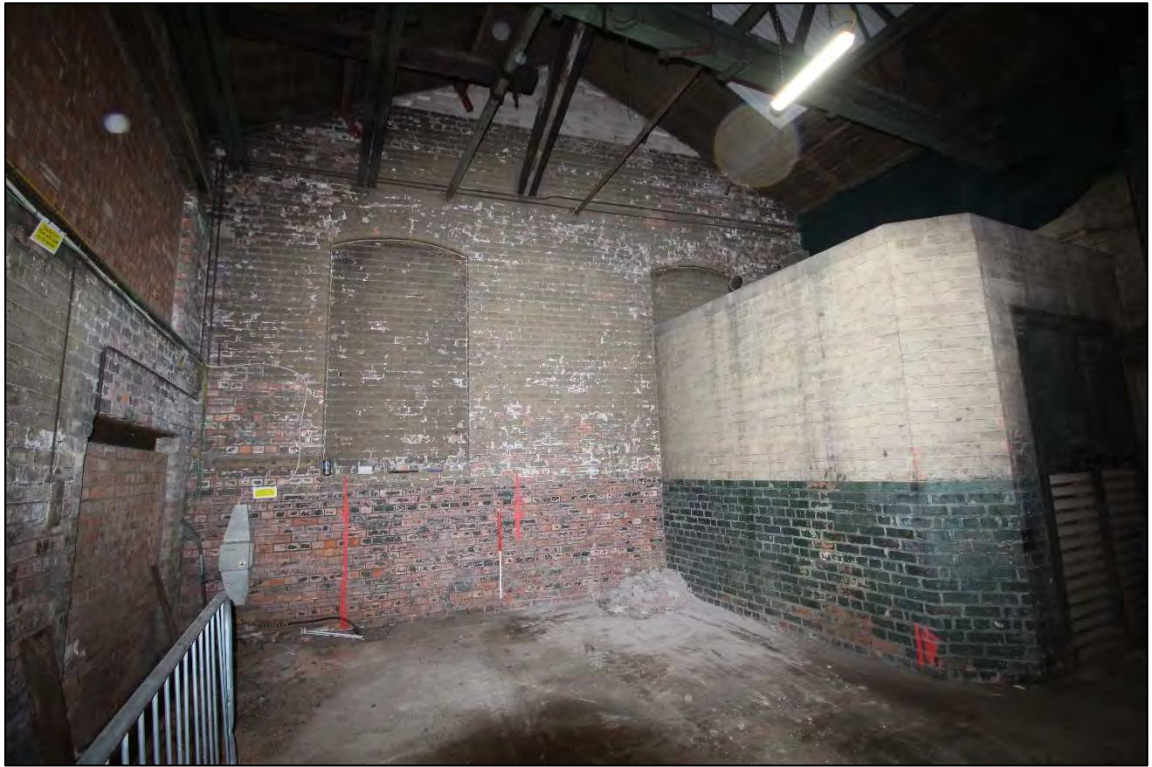
Plate 31: The blocked windows to the southern wall of Room 1
