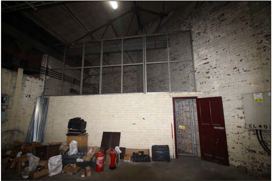
Plate 37: The brick and steel mesh partition wall between Rooms 3 and 4, looking south
