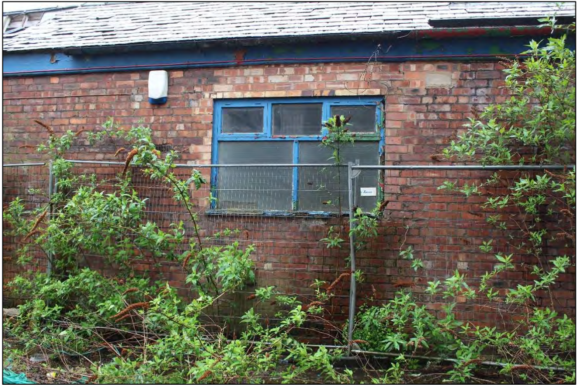
Plate 13: The central window within the norther elevation of Shed 1
