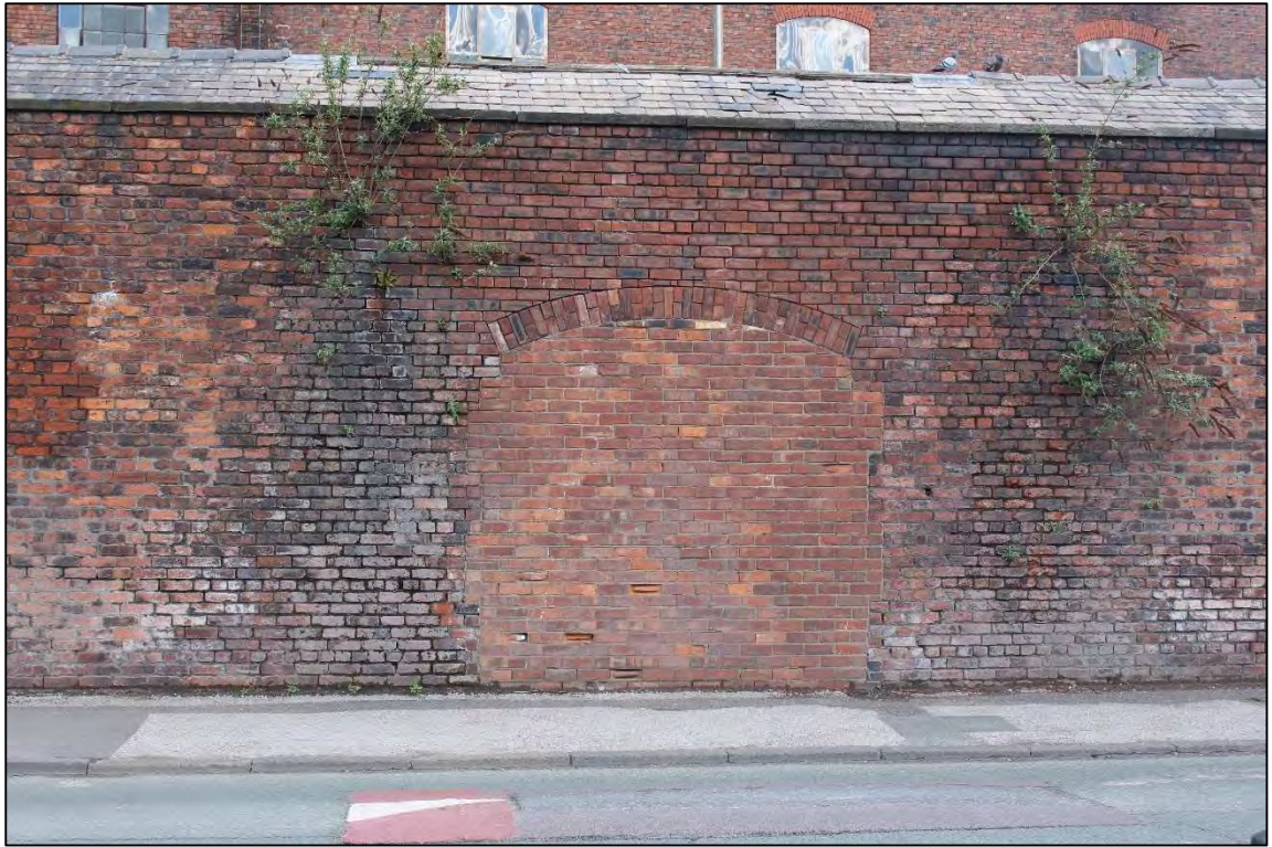
Plate 16: Detail of the infilled doorway within the southern elevation
