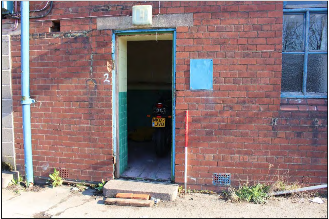
Plate 49: Detail of the western doorway within the southern elevation, looking north
