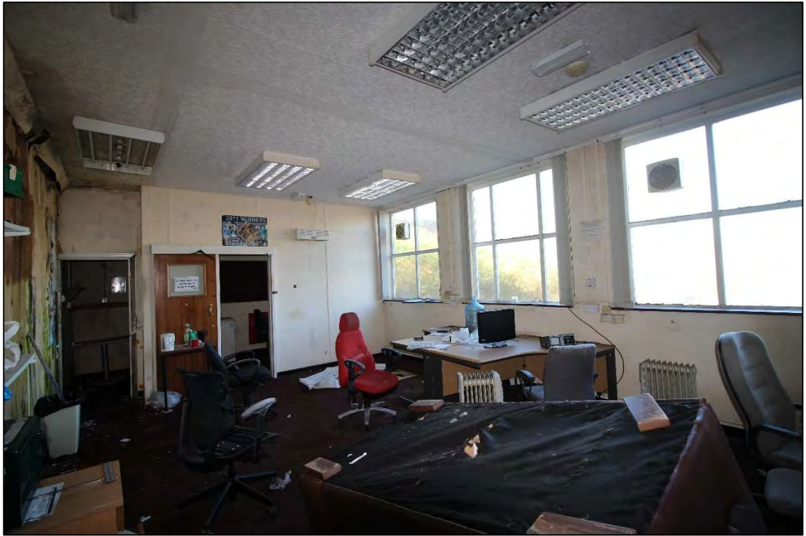
Plate 45: General view of Room 3 of the office block, facing south-west
