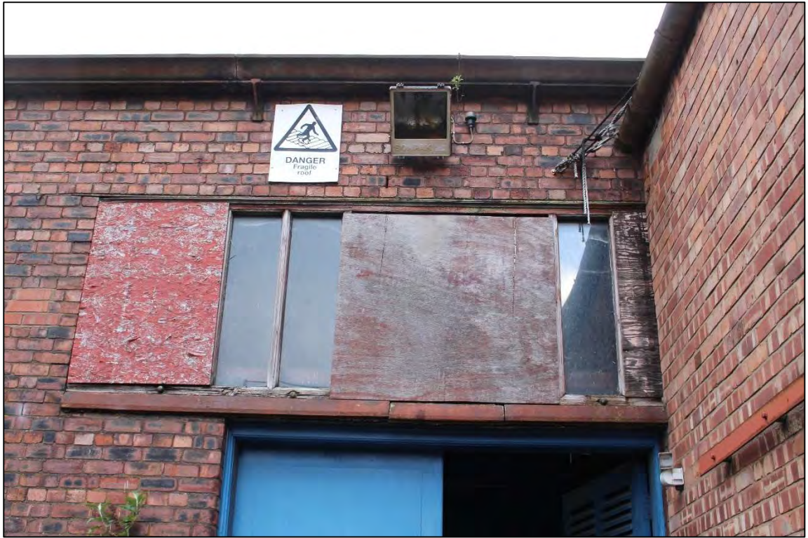
Plate 20: Detail of the window above the doorway within the eastern elevation
