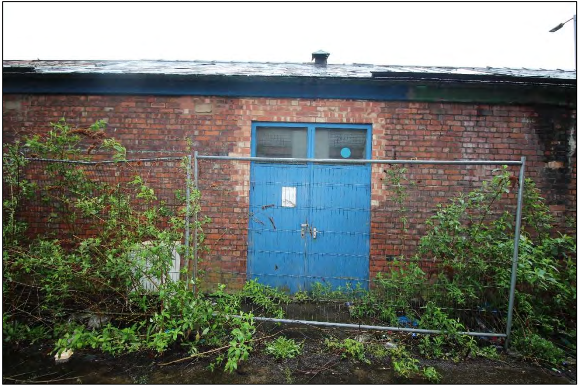
Plate 14: The western doorway within the norther elevation of Shed 1
