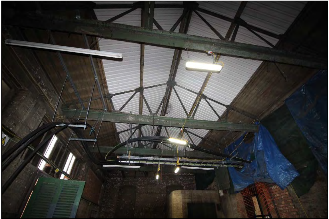
Plate 27: Detail of the fink trusses in Room 1
