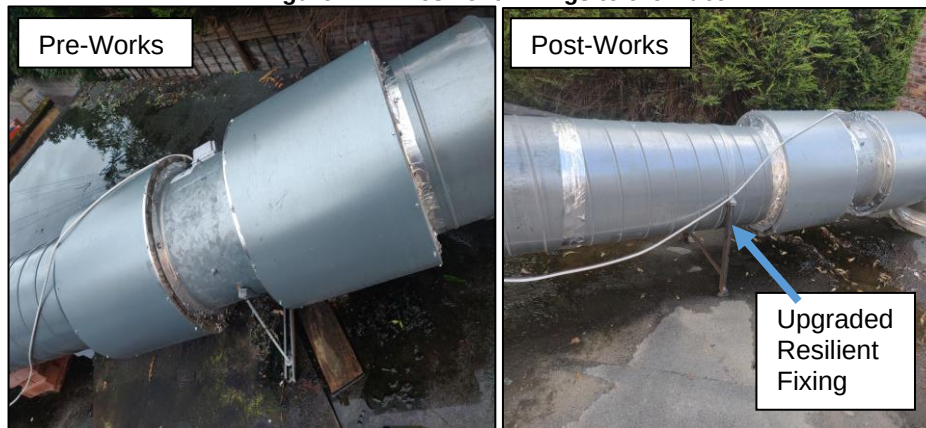
Figure 1.1 – Resilient Fixings to the Duct
