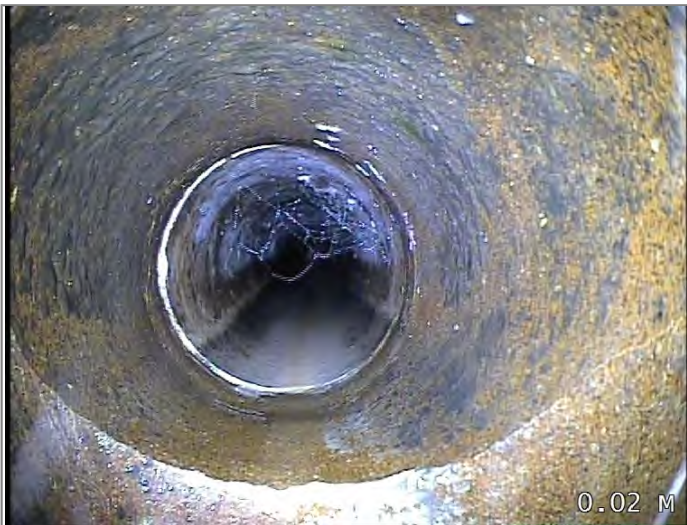
Start node type, manhole, reference MH12
