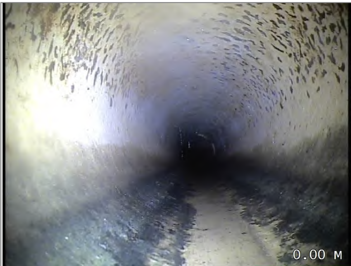
Start node type, manhole, reference MH4
