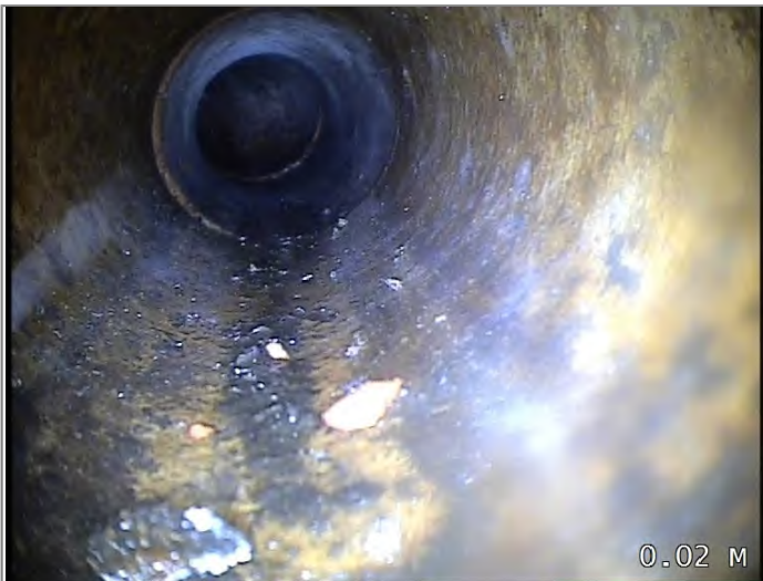
Start node type, manhole, reference MH13
