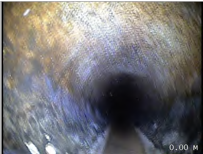
Start node type, manhole, reference MH13
