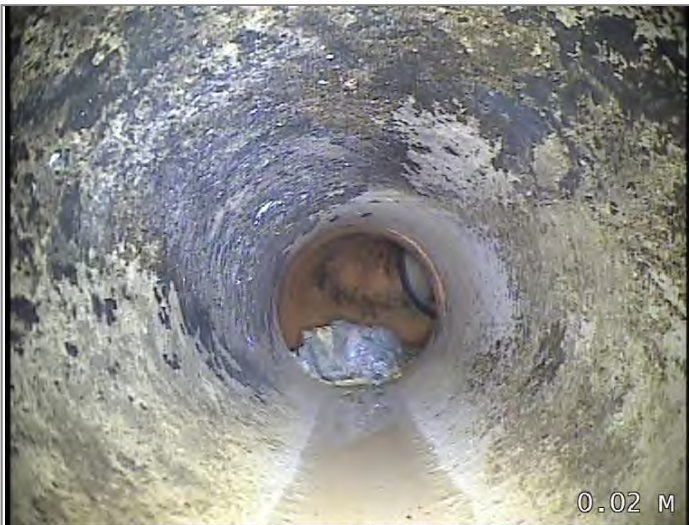
Start node type, manhole, reference MH6
