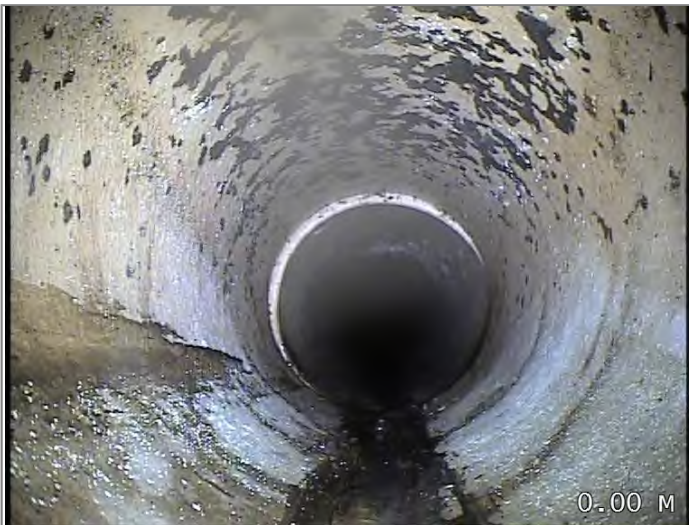
Start node type, manhole, reference MH11
