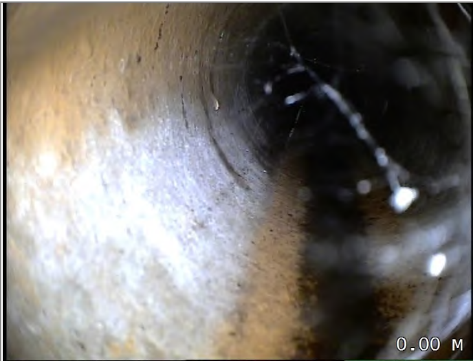
Start node type, manhole, reference MH11
