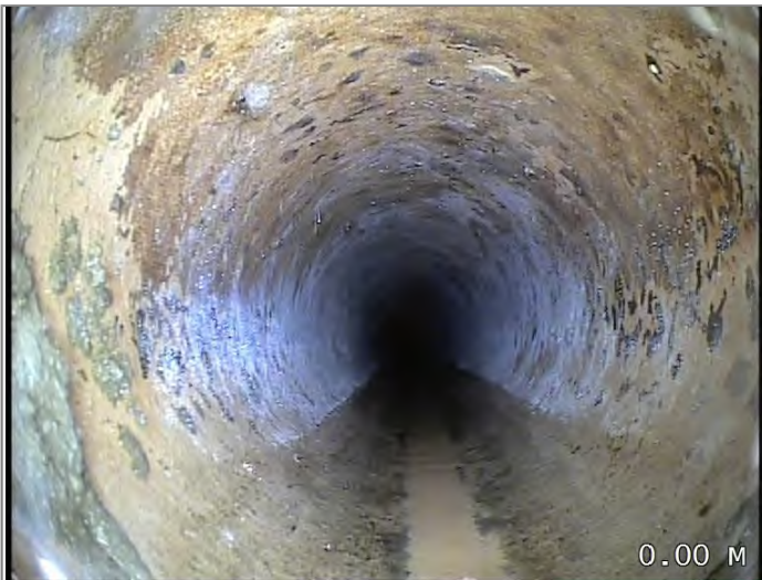
Start node type, manhole, reference MH18
