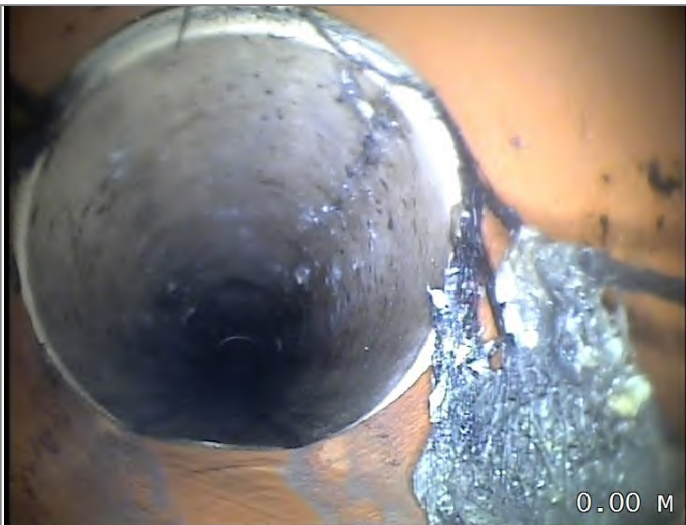
Start node type, manhole, reference MH7
