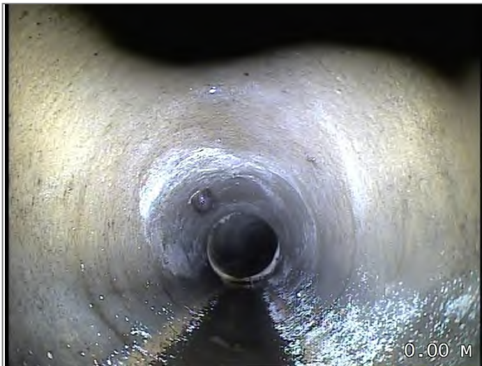
Start node type, manhole, reference MH17
