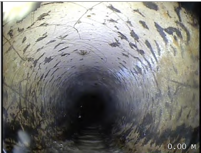
Start node type, manhole, reference MH19
