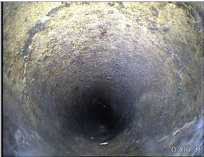
Start node type, manhole, reference MH13
