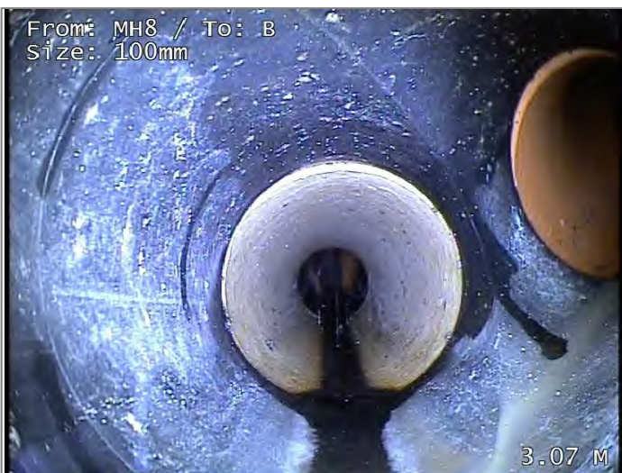
Junction at 3 o'clock, diameter 100mm
