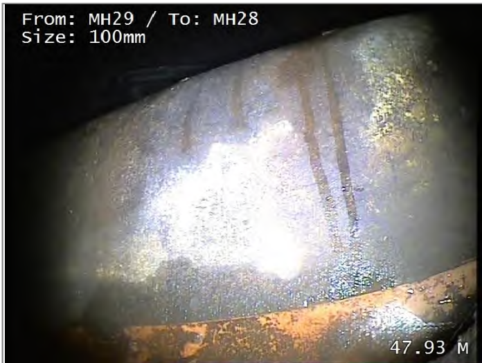
Finish node type, manhole, reference MH28
