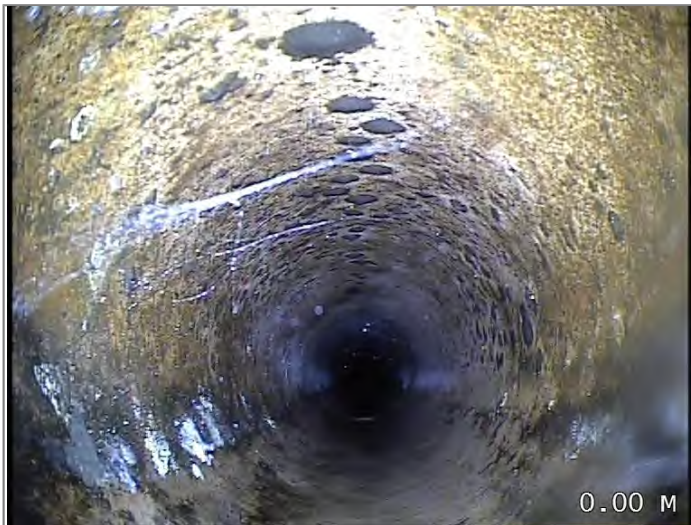
Start node type, manhole, reference MH13
