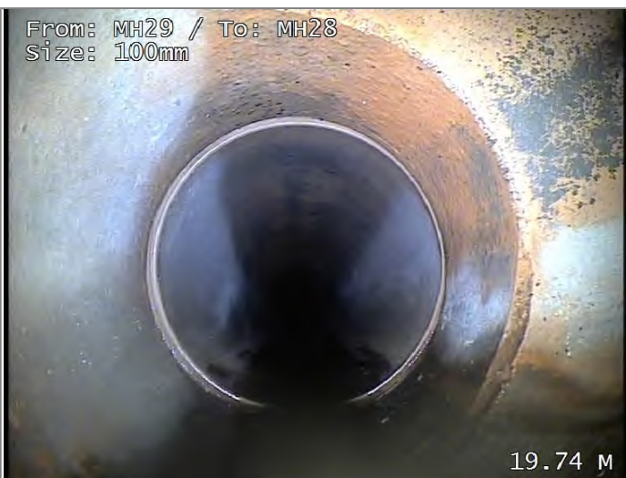
Junction at 3 o'clock, diameter 100mm
