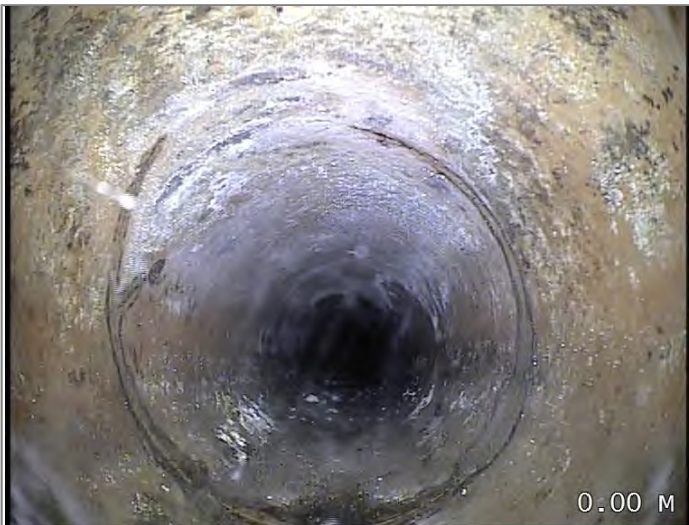
Start node type, manhole, reference MH18
