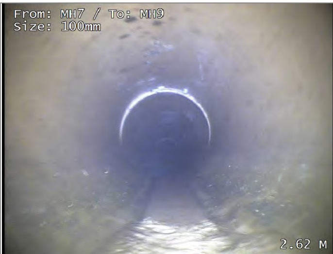
Dimensions of drain/sewer changes to 150mm
