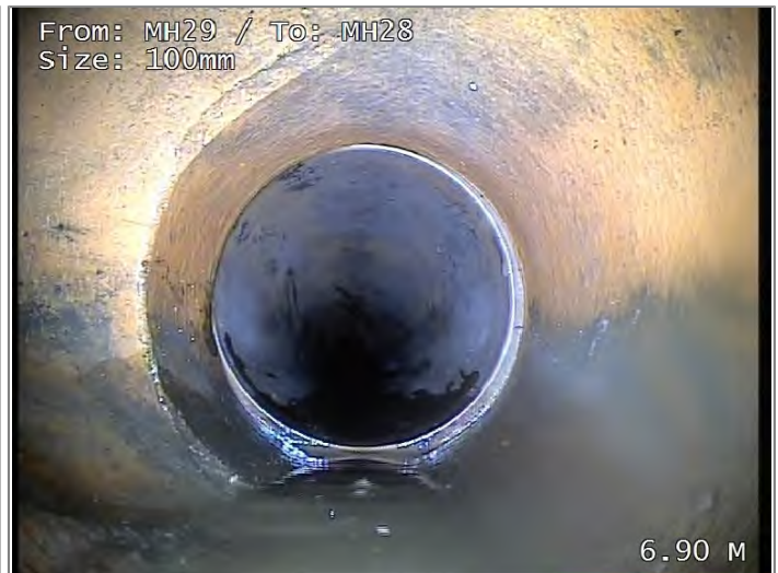
Junction at 9 o'clock, diameter 100mm
