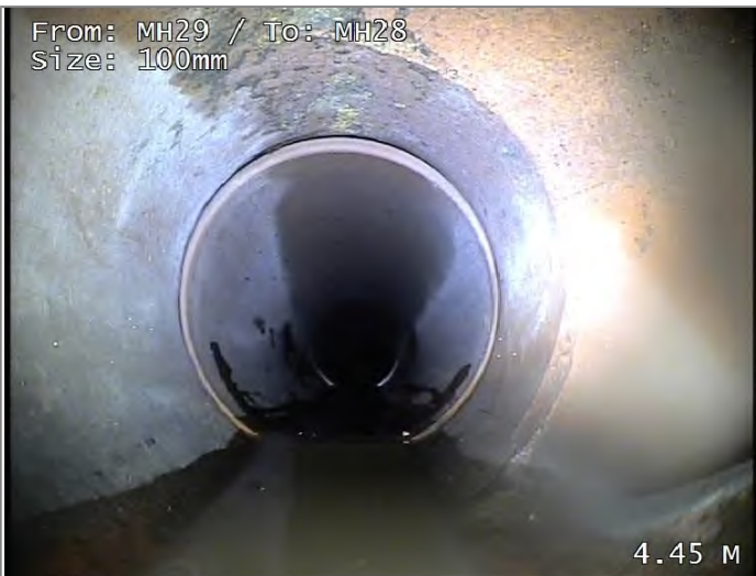
Junction at 2 o'clock, diameter 100mm
