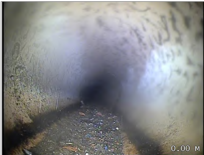
Start node type, manhole, reference MH7
