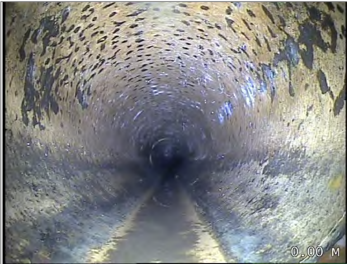
Start node type, manhole, reference MH6
