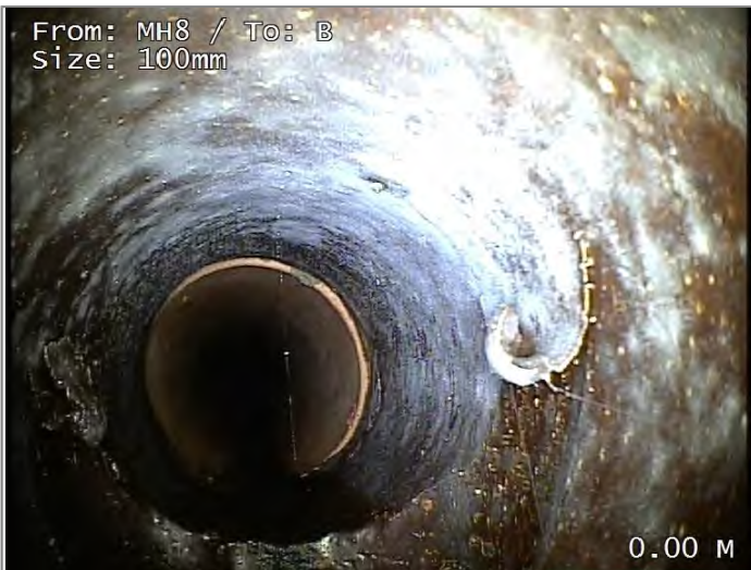
Junction at 6 o'clock, diameter 100mm
