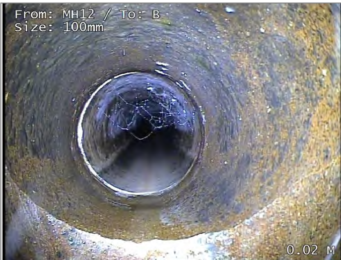
Junction at 6 o'clock, diameter 100mm
