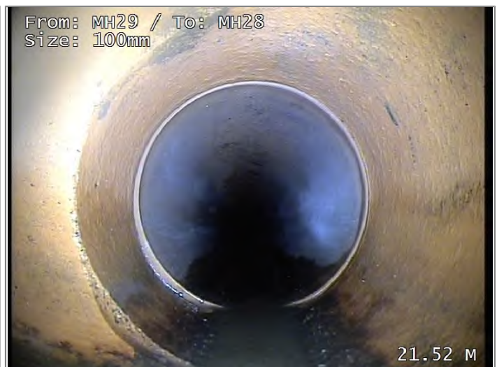
Junction at 9 o'clock, diameter 100mm
