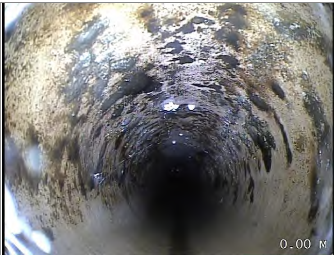
Start node type, manhole, reference MH9
