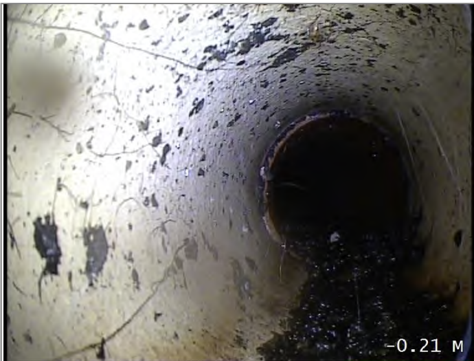
Start node type, manhole, reference MH16
