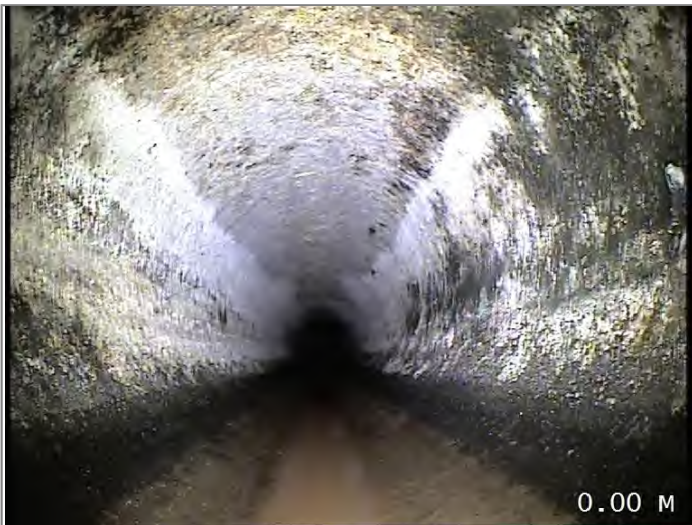
Start node type, manhole, reference MH9
