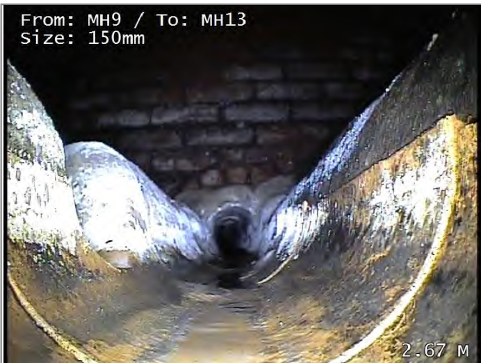
Finish node type, manhole, reference MH13
