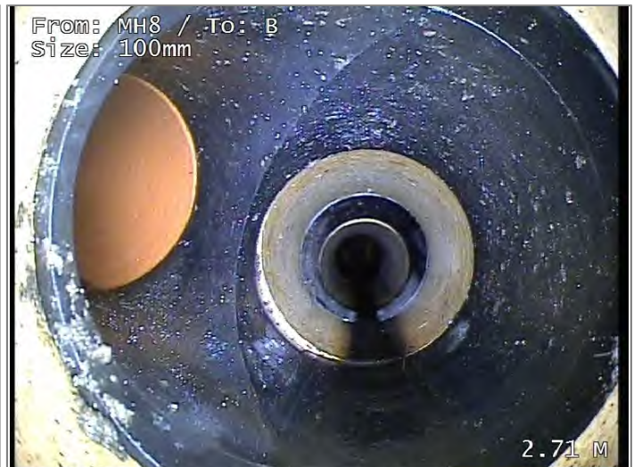
Junction at 10 o'clock, diameter 100mm
