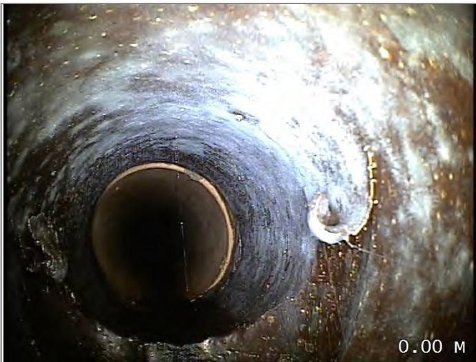
Start node type, manhole, reference MH8
