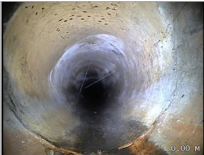
Start node type, manhole, reference MH17
