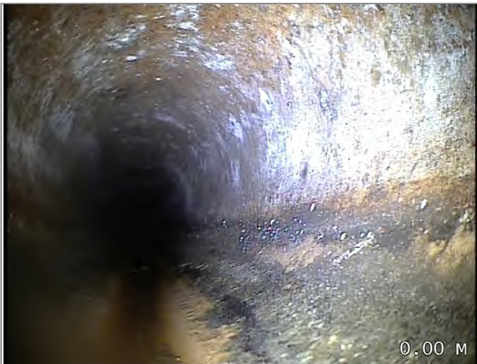
Start node type, manhole, reference MH3
