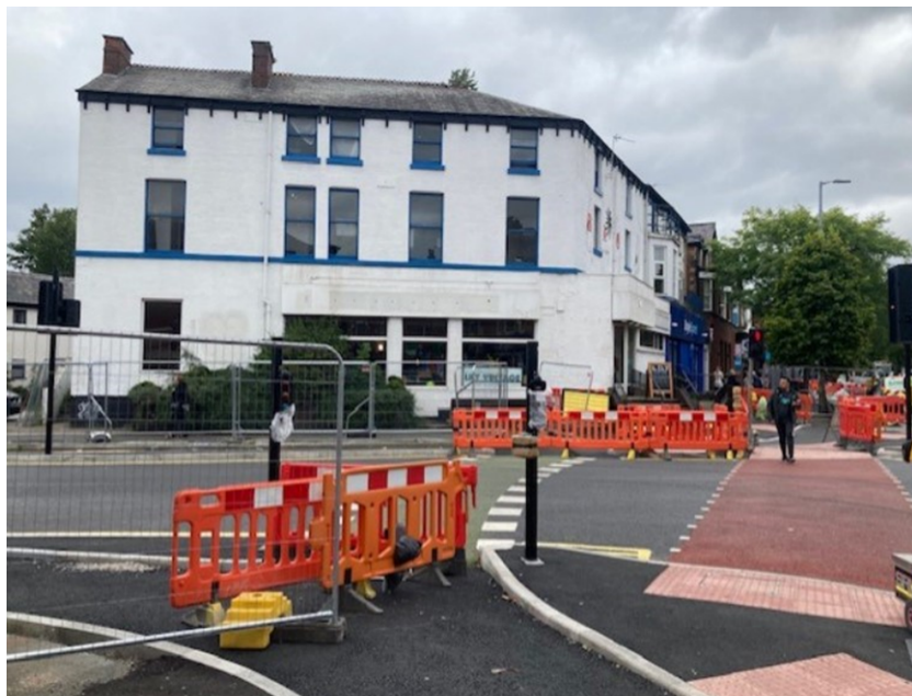
View of application site from Barlow Moor Rd/Wilbraham Rd junction
