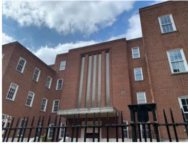
Photograph 1 – The building's northern aspect
