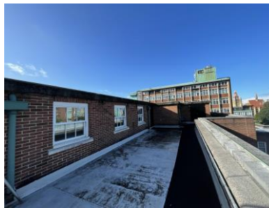
Photograph 5 – Northern aspect of eastern plant store room
