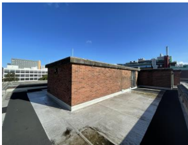
Photograph 4 – Southern aspect of western plant store room
