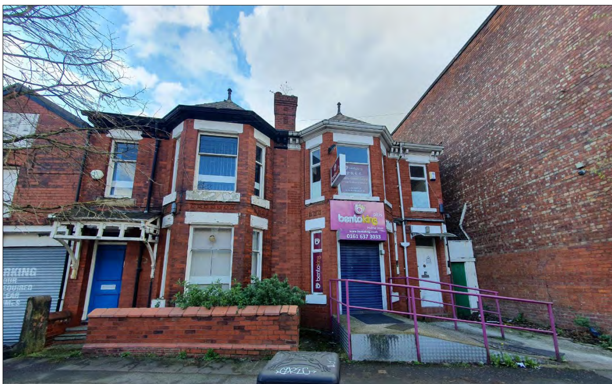
Plate 20 Photograph of double-depth terraces on Greenheys Lane, facing east
