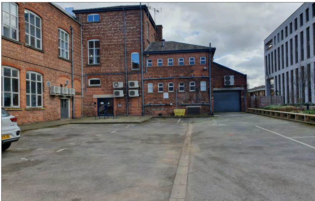
Plate 15 Photograph of the west end of the garage and car park in the west of the Site, off Greenheys Lane, facing east
