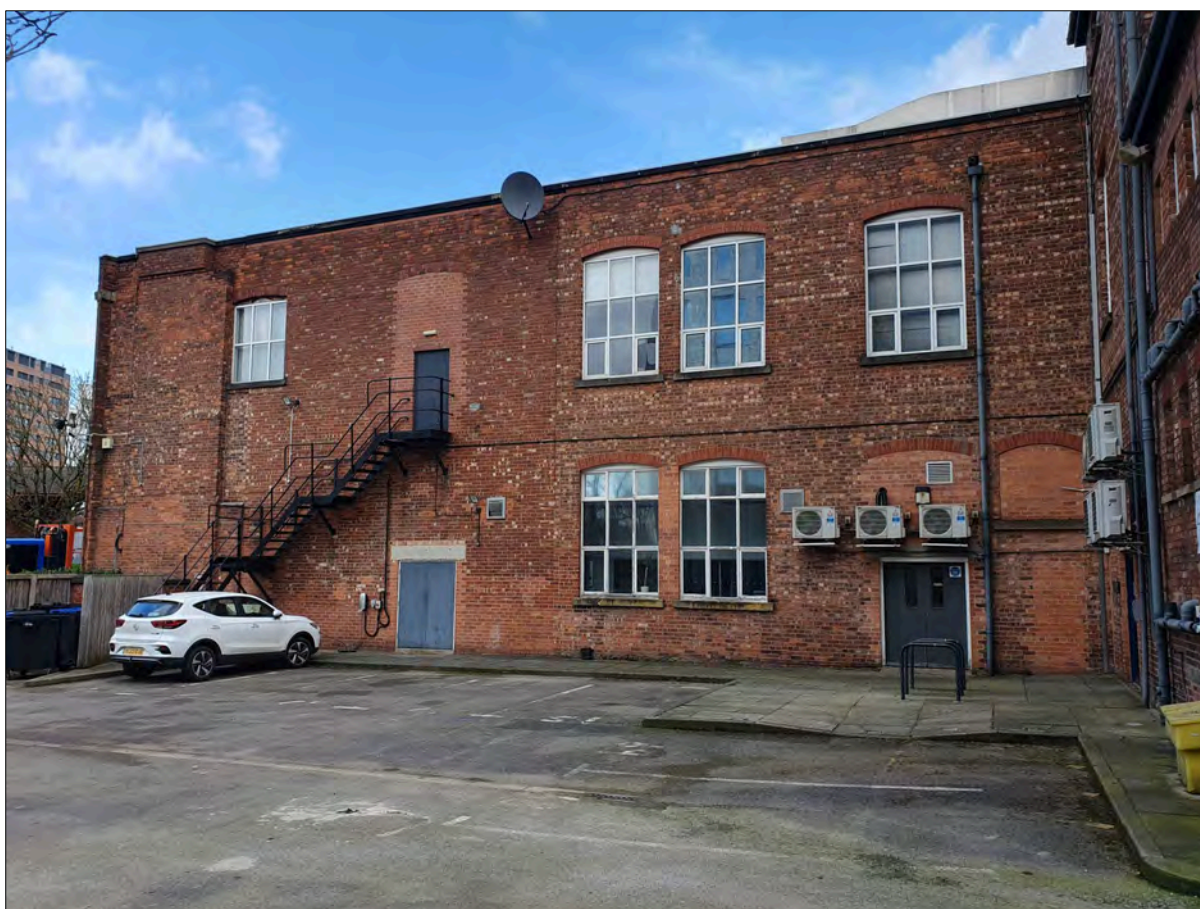
Plate 17 Photograph showing the south elevation of the garage that front Greenheys Lane, facing north
