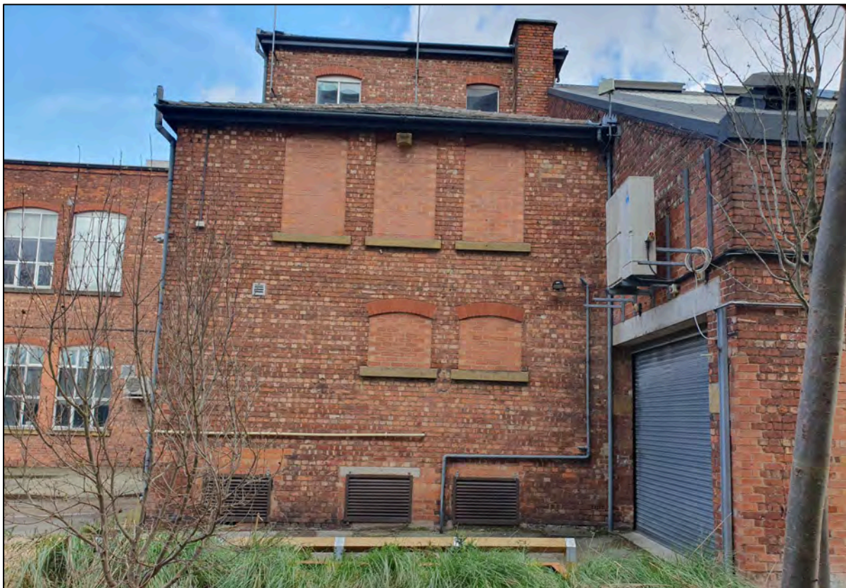
Plate 14 Photograph of west end of the garage that lies within the Site, facing north
