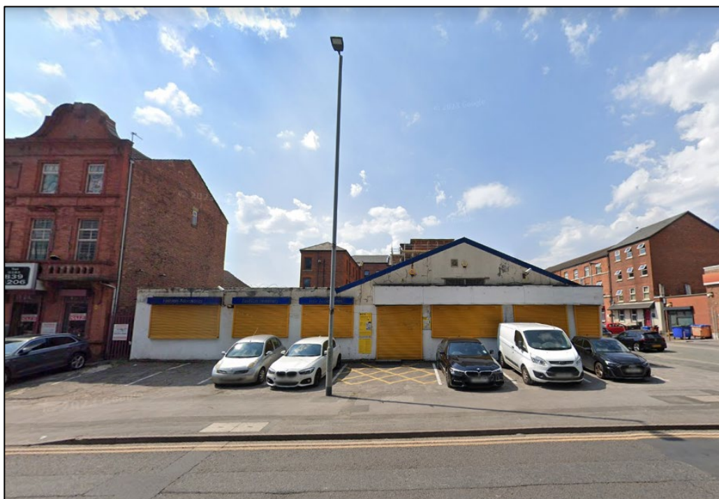
Figure 2.2 Existing building at the site (Cheetham Hill Road frontage)
